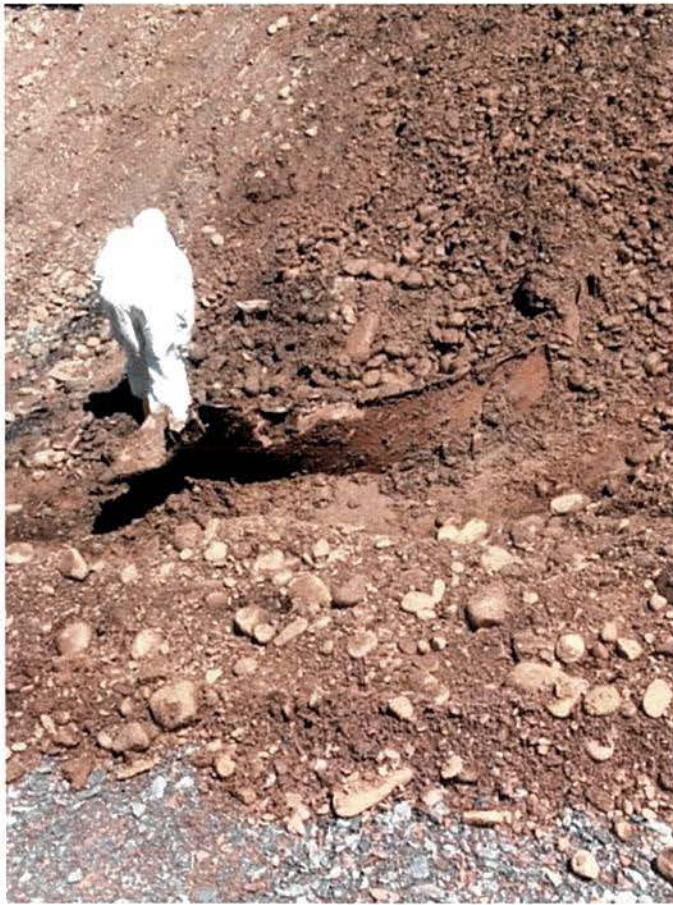
Photo 3: Silo Wall Exposed Near B-03
