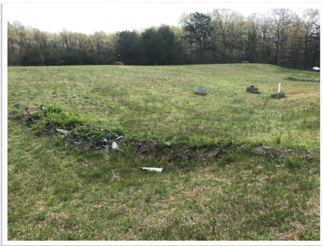
Photo: 010 Date: 04/23/18 Description: Near MW-2SU. Overgrown vegetation within rock dam. Photographer: [REDACTED]
