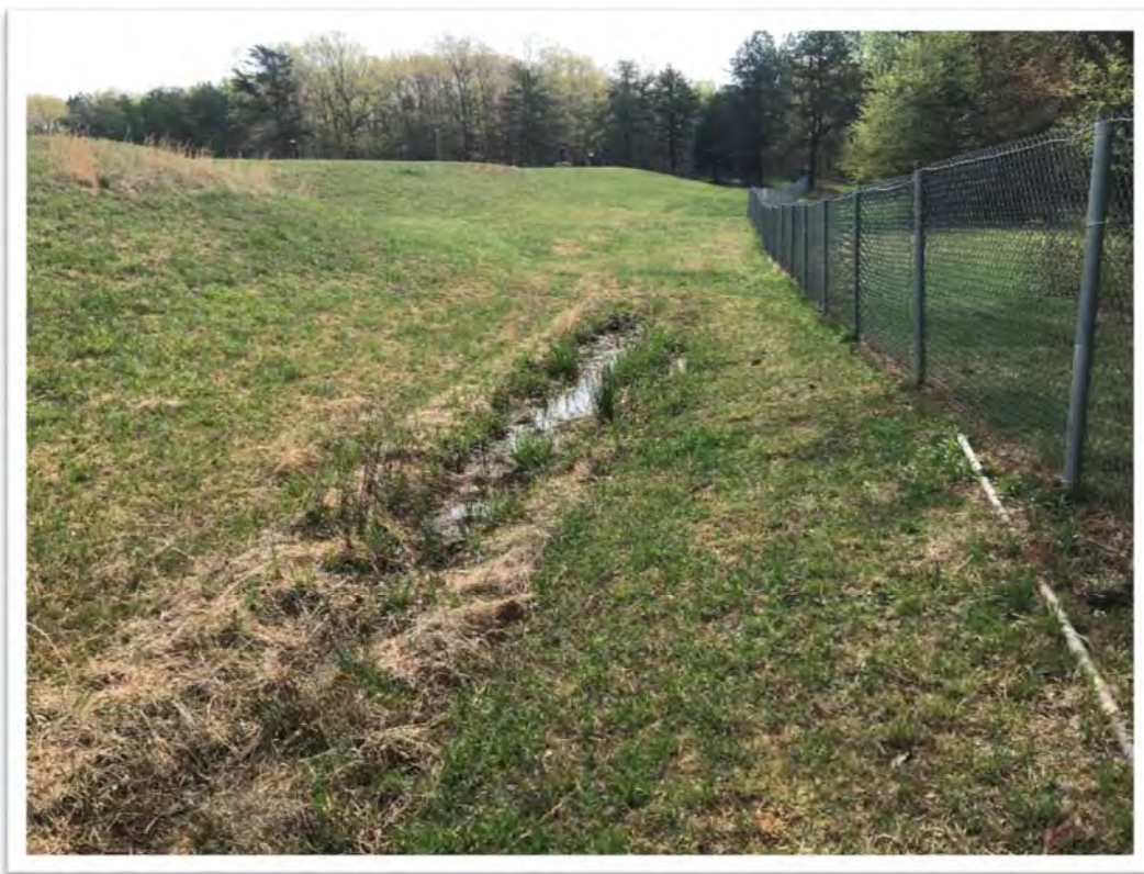
Photo: 014 Date: 04/23/18 Description: Facing southwest at northeast corner of landfill. Standing water and overgrown vegetation. Photographer: [REDACTED]
