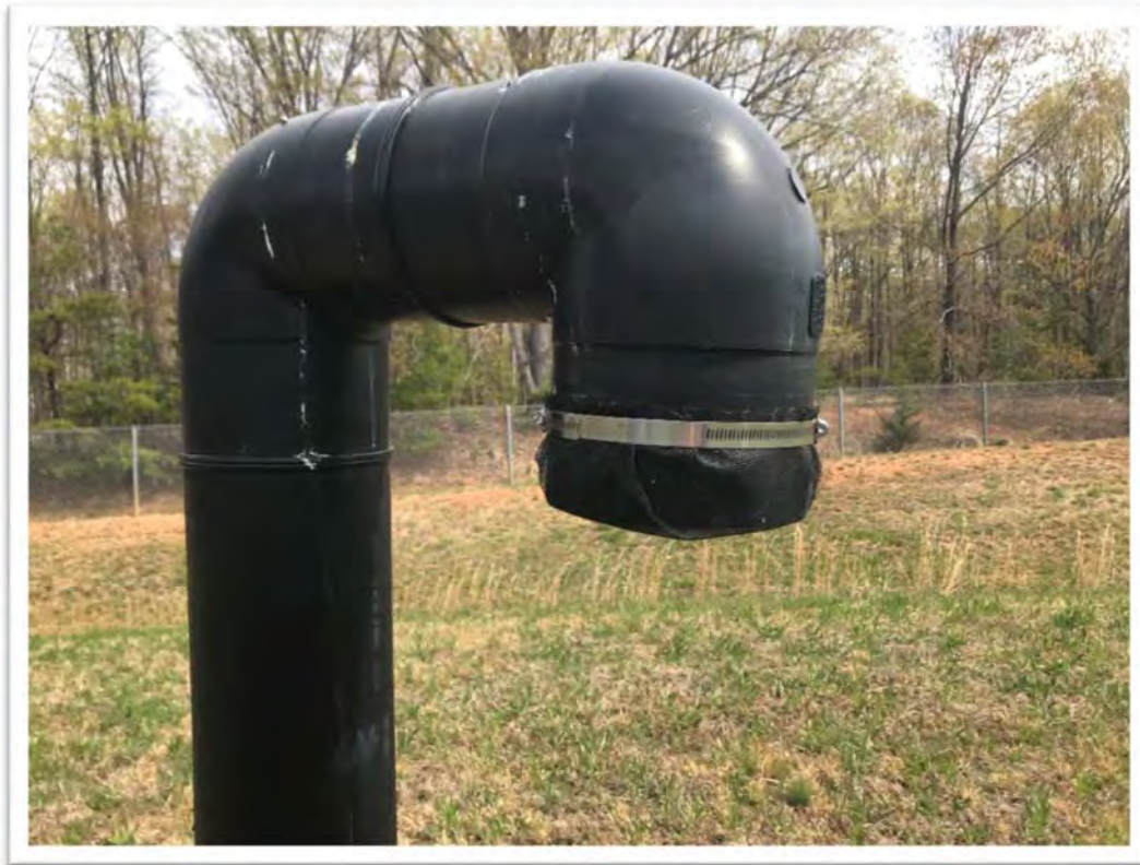
Photo: 009 Date: 04/23/18 Description: On Landfill. Gas vent, GV-4, in good condition. Photographer: [REDACTED]
