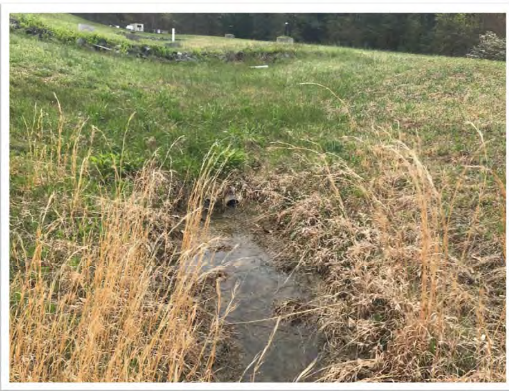
Photo: 004 Date: 04/23/18 Description: Clogged drainage pipe located at the northern portion of Landfill. Photographer: [REDACTED]
