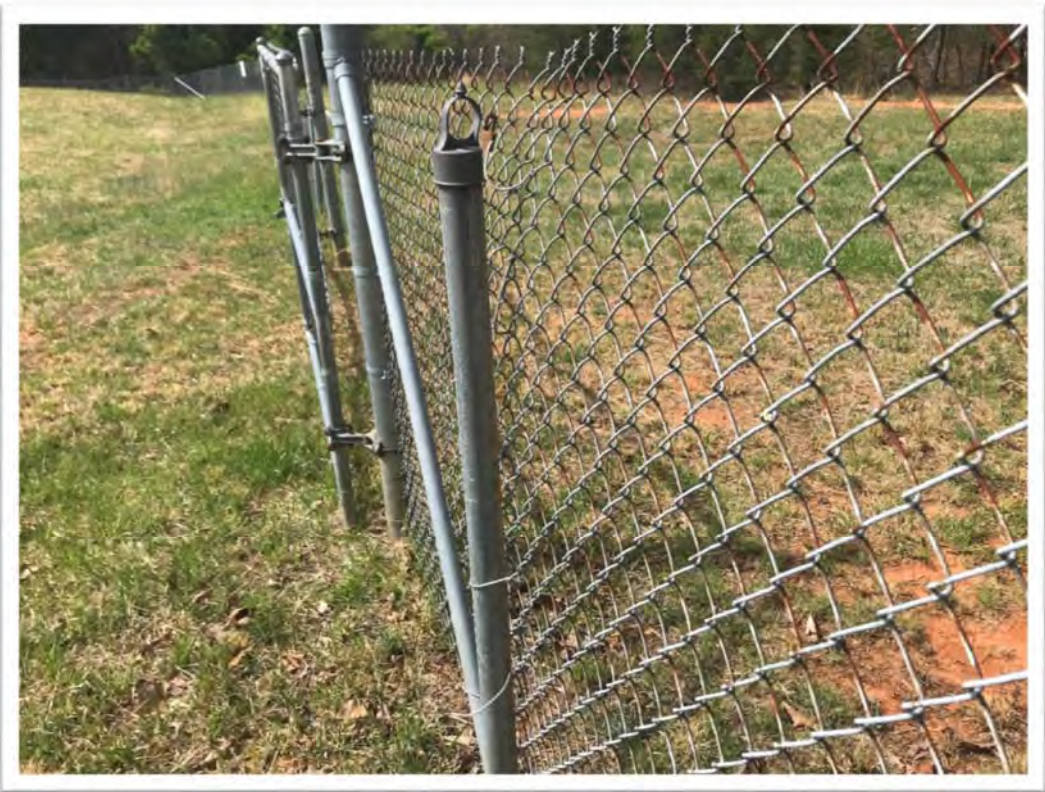
Photo: 007 Date: 04/23/18 Description: Loose fence pole at northwestern edge of landfill. Photographer: [REDACTED]
