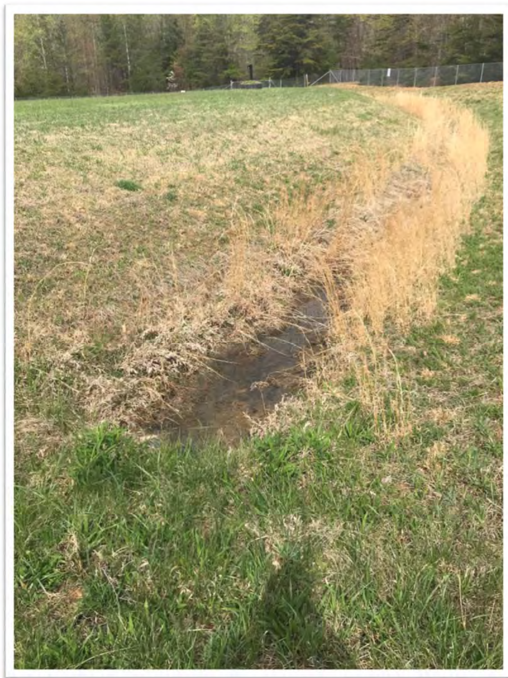
Photo: 003 Date: 04/23/18 Description: Facing northwest at Landfill. Standing water in drainage swale. Photographer: [REDACTED]
