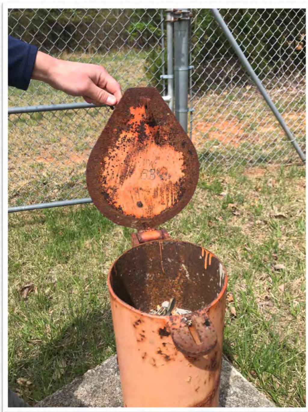
Photo: 015 Date: 04/23/18 Description: At monitoring well, MW-3B. Well protective casing missing lock. Photographer: [REDACTED]
