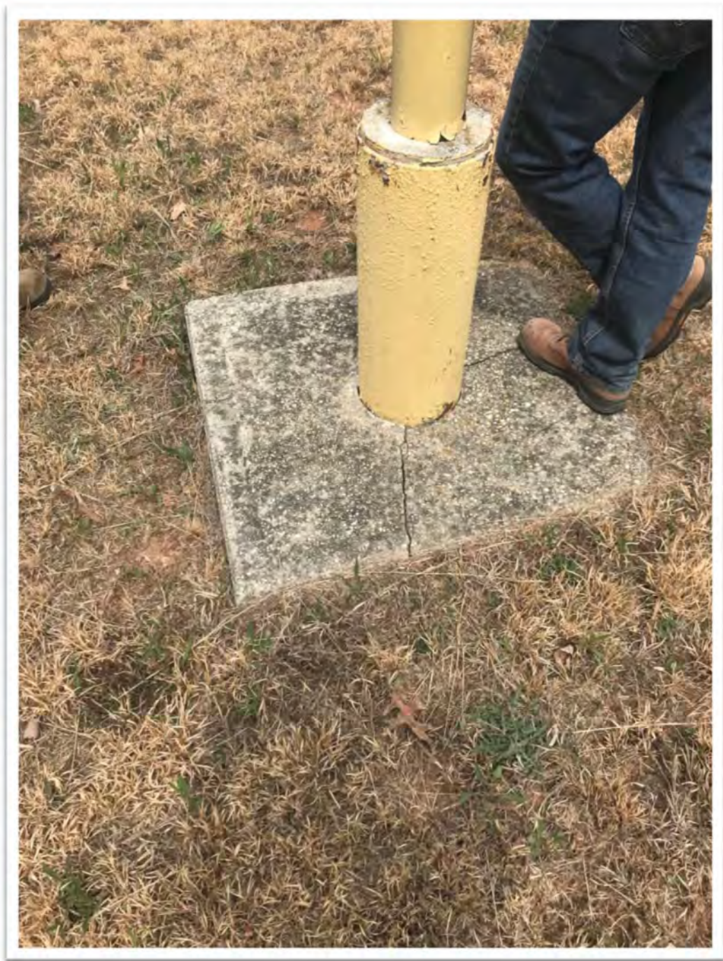
Photo: 018 Date: 04/23/18 Description: At monitoring well, MW-25SL. Well pad cracked. Photographer: [REDACTED]
