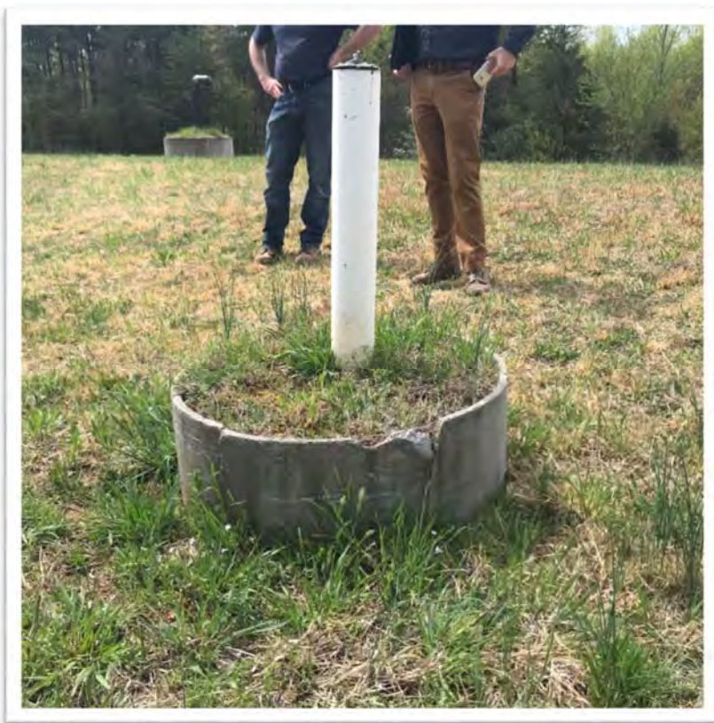
Photo: 016 Date: 04/23/18 Description: At monitoring well, MW-2SU. Concrete ring cracked. Photographer: [REDACTED]
