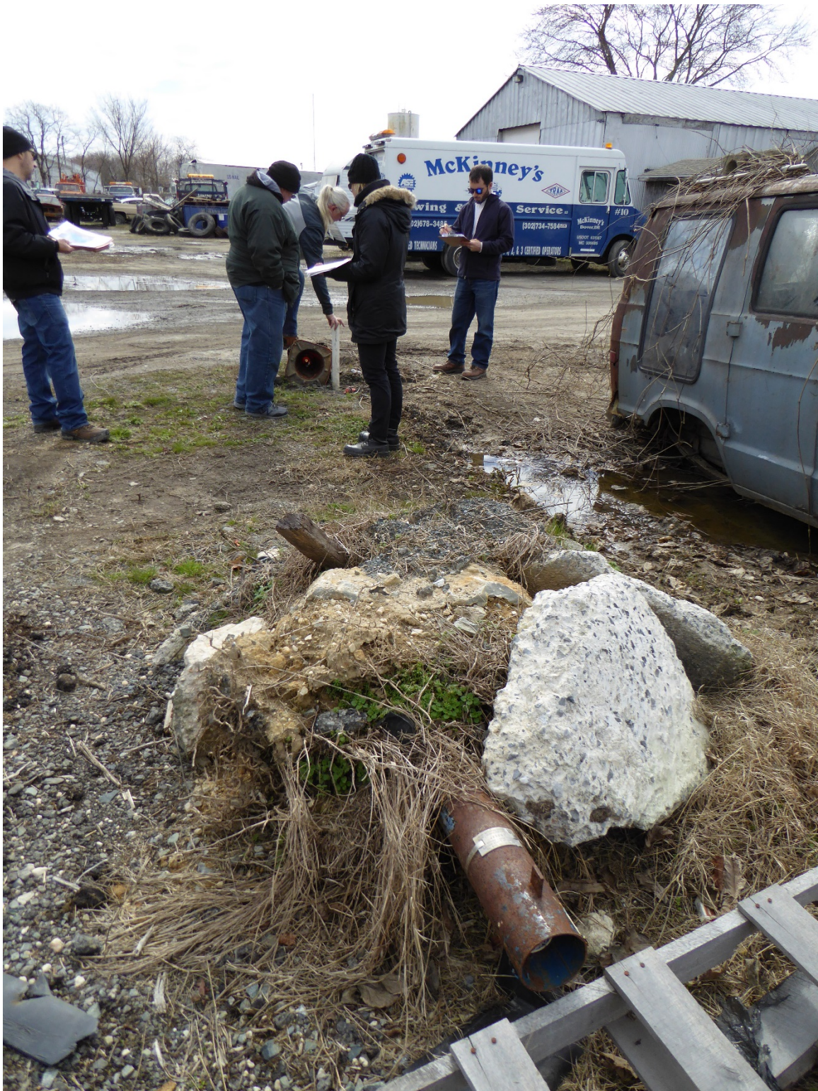
Destroyed monitoring well MW-97-10-45
