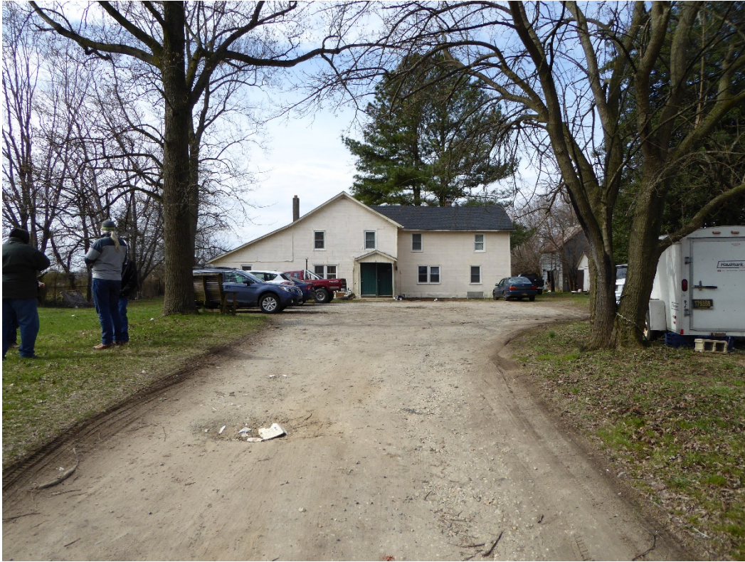
Residential building on former facility property
