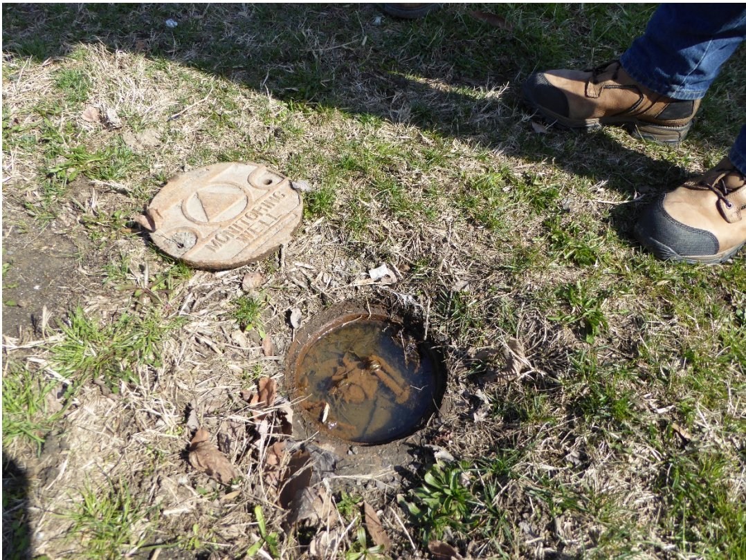
Unsecured monitoring well with standing water
