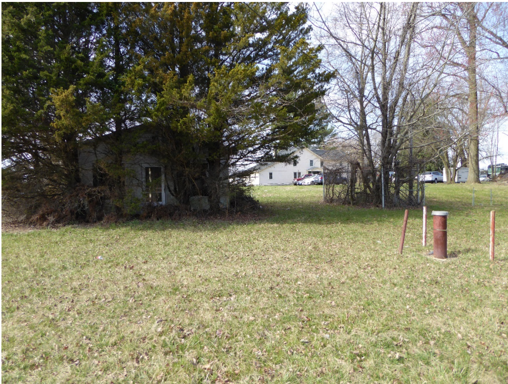
Abandoned Chem-Solv office building
