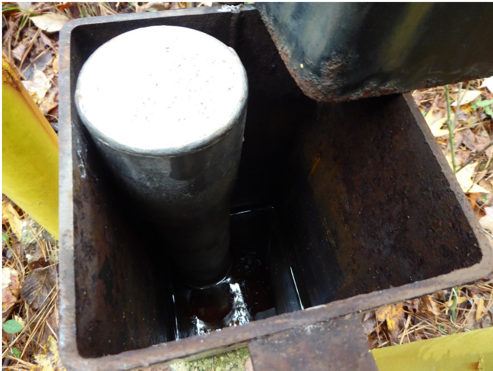
VPMW-5 (standing water outside inner well casing)
