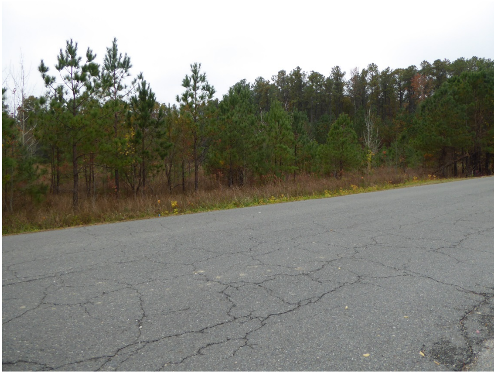
Looking southeast across Peyton Street toward former Wetland Area C
