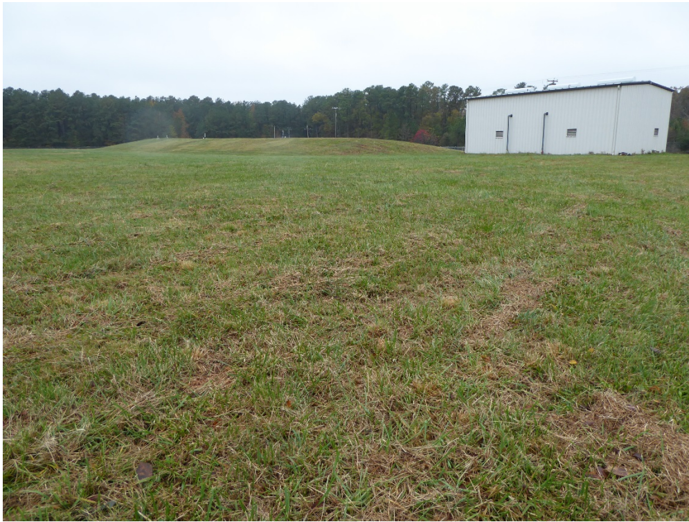
Looking northwest across original capped area
