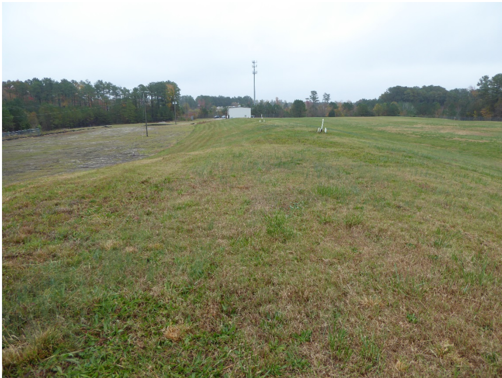
Looking northeast along newly capped area (left) and original capped area (right)
