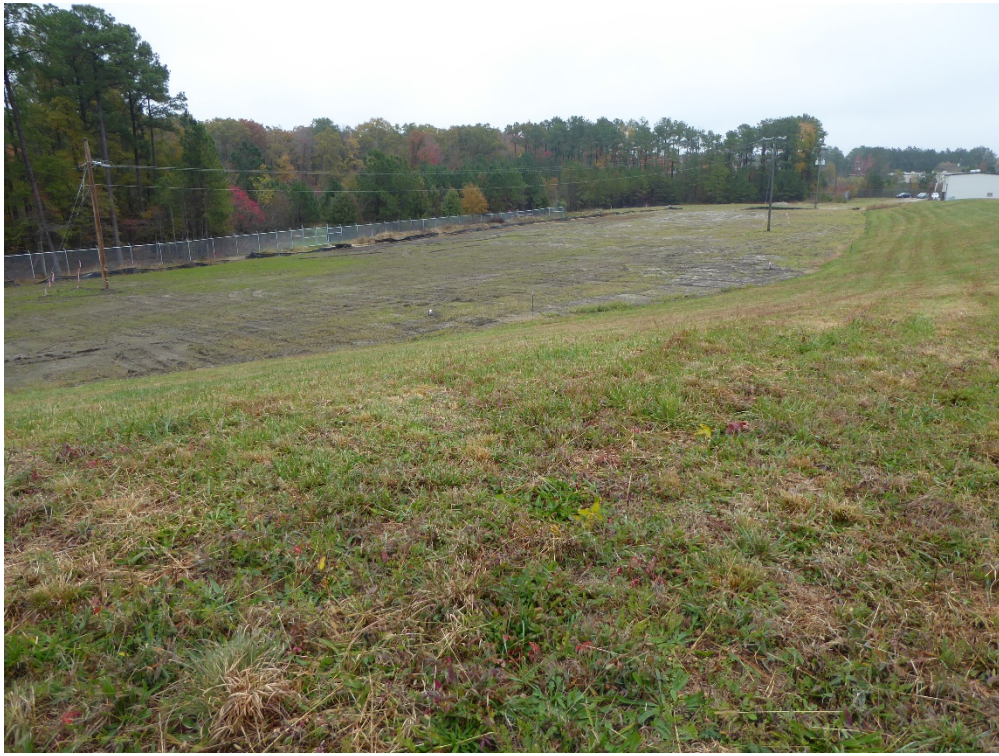
Looking northeast at newly capped area
