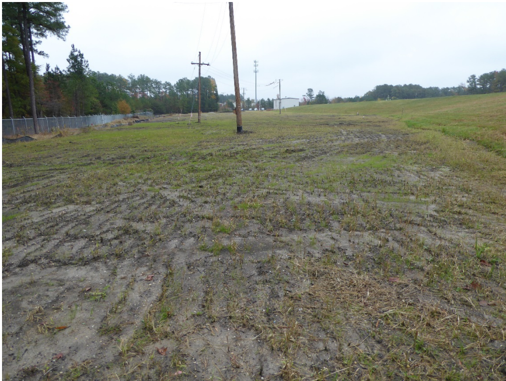
Looking northeast across newly capped area
