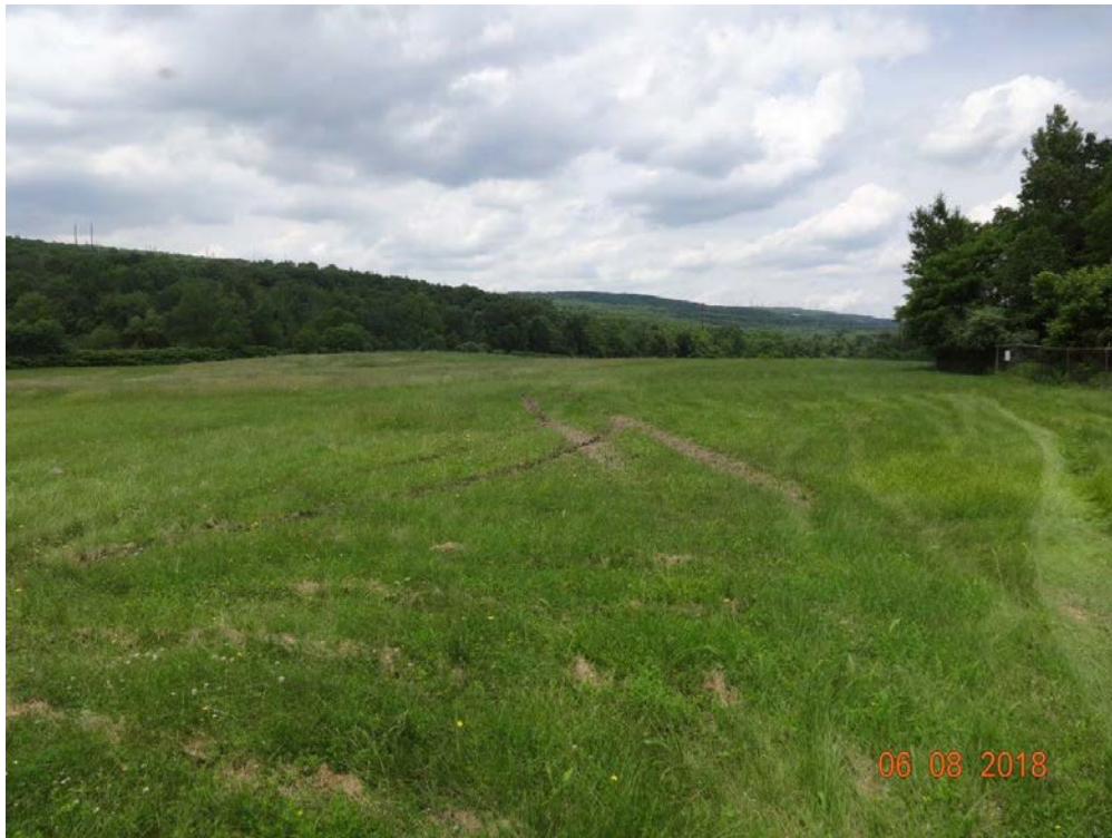
Photo G-15: 06/08/18 – Ruts on capped area
