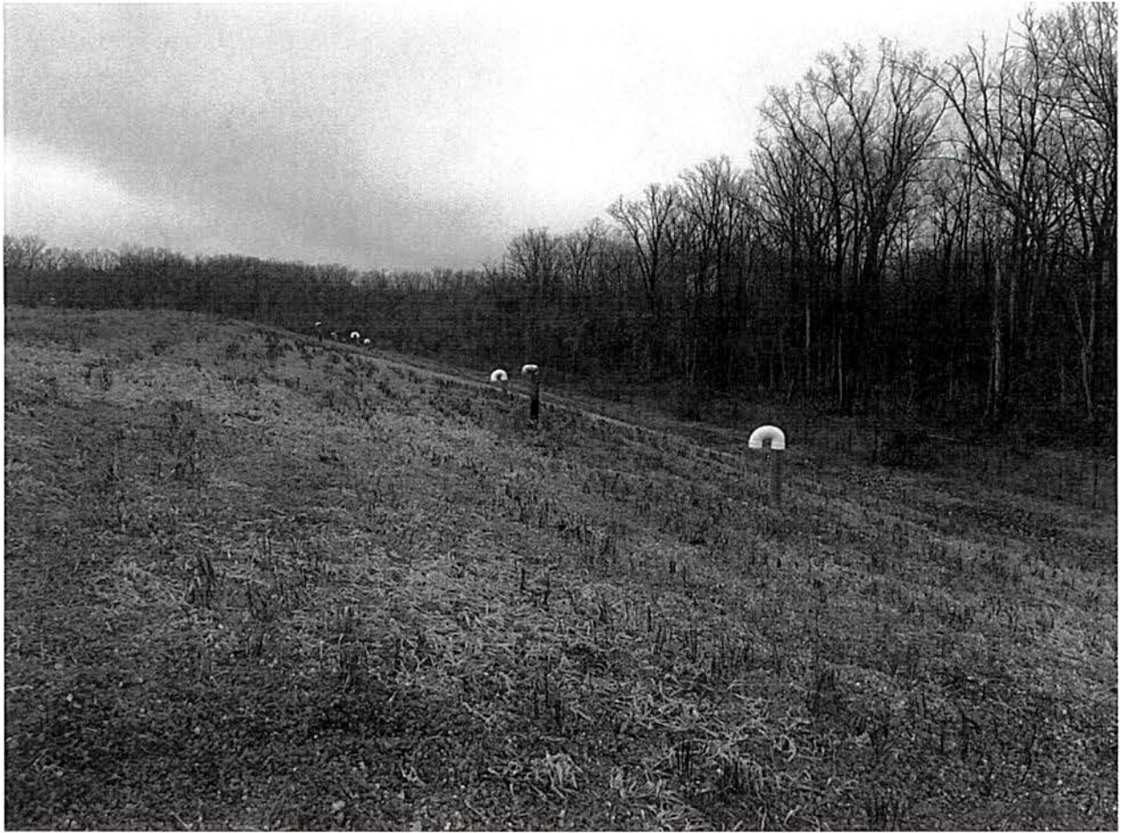
Photograph of south side of landfill. Landfill gas vents are depicted in photograph.
