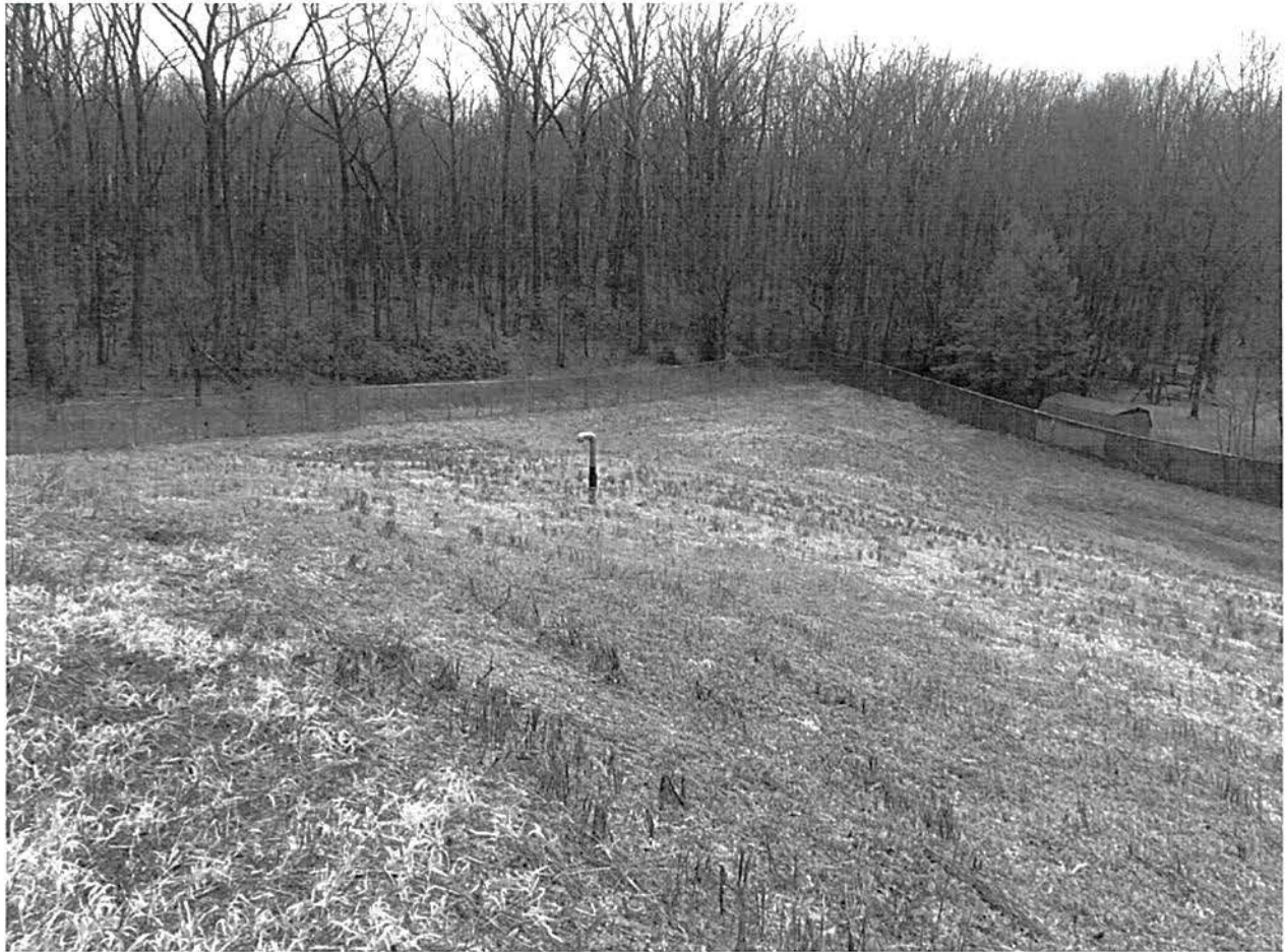
Photograph of southwest corner of landfill. Landfill gas vent in center of photo. View of wooded area to south of landfill in background.
