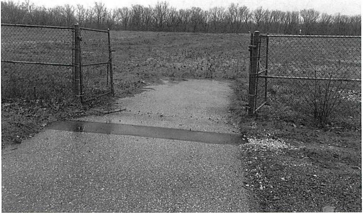
Photograph of main gate to landfill cap.
