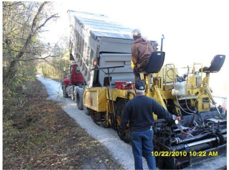
10/22/2010 Paving of the trail. SAM_0038.JPG
