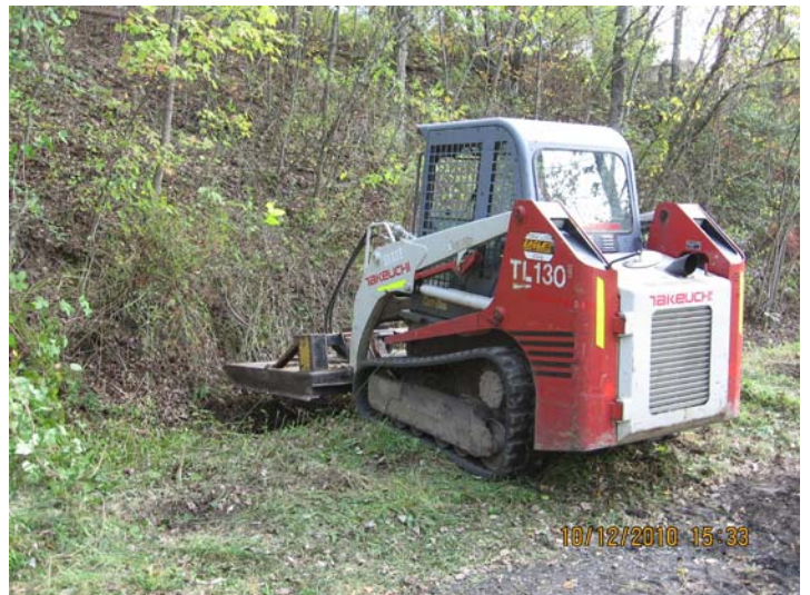
10/12/2010 ERRS skidsteer performing brush clearing - looking (SE) IMG_5450.jpg
