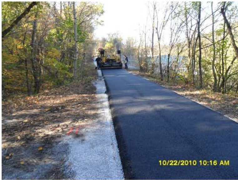
10/22/2010 Paving of the trail. SAM_0037.JPG
