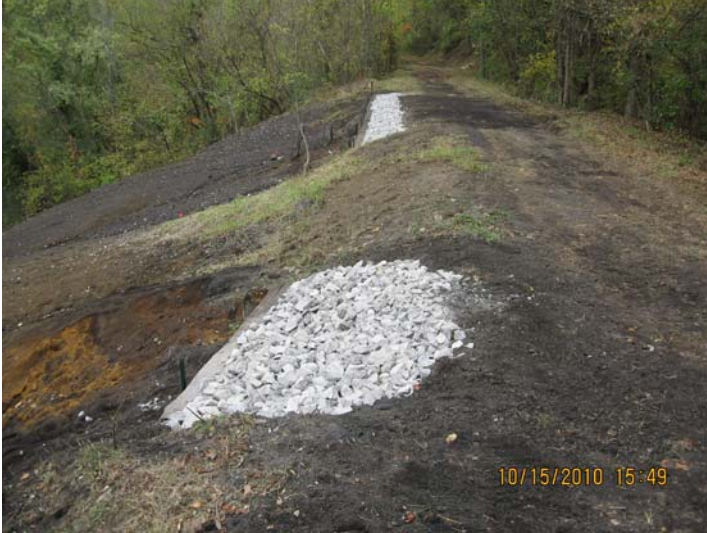
10/15/2010 Slag pile boundary with riprap installed in buttress system (N) IMG_5536.jpg
