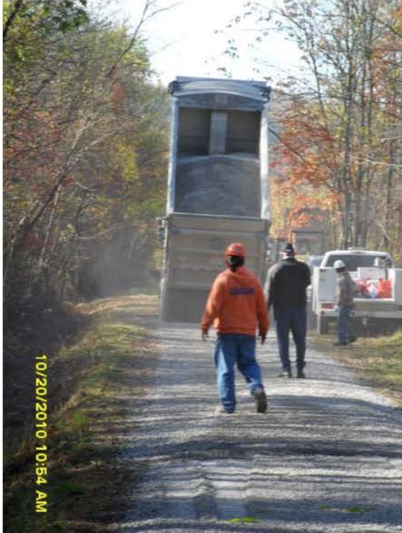
10/20/2010 Dump truck unloading and spreading crush-n-run on the trail. SAM_0023.JPG
