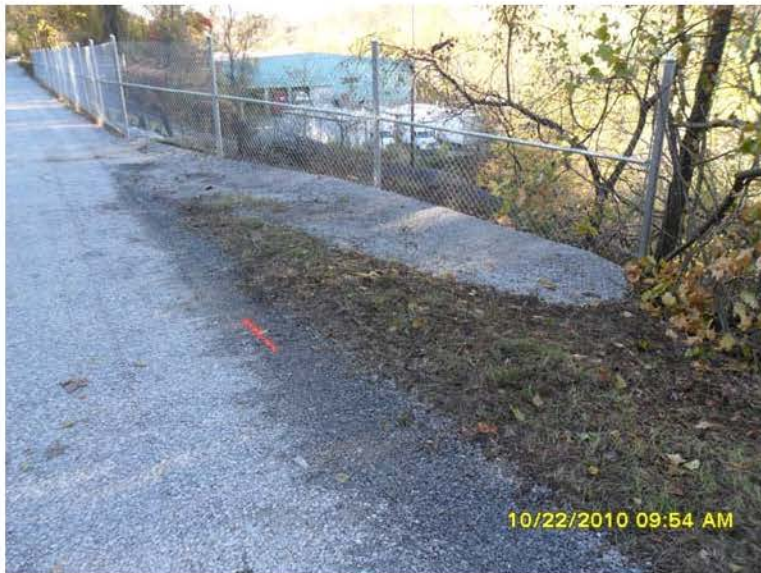
10/22/2010 Stone placed at base of fence to eliminate the gap which had previously been u... SAM_0032.JPG
