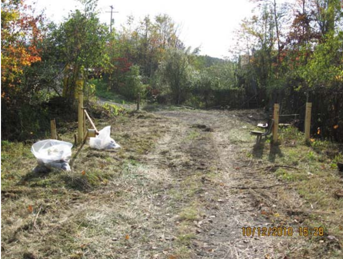
10/12/2010 Area of trail cleared and grubbed by ERRS (South) IMG_5443.jpg
