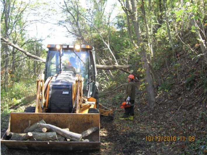
10/13/2010 ERRS crew using excavator to pull down tree - looking north IMG_5473.jpg
