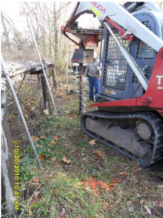
10/20/2010 ERRS using skidsteer with an auger attachment to dig the SAM_0019.JPG
