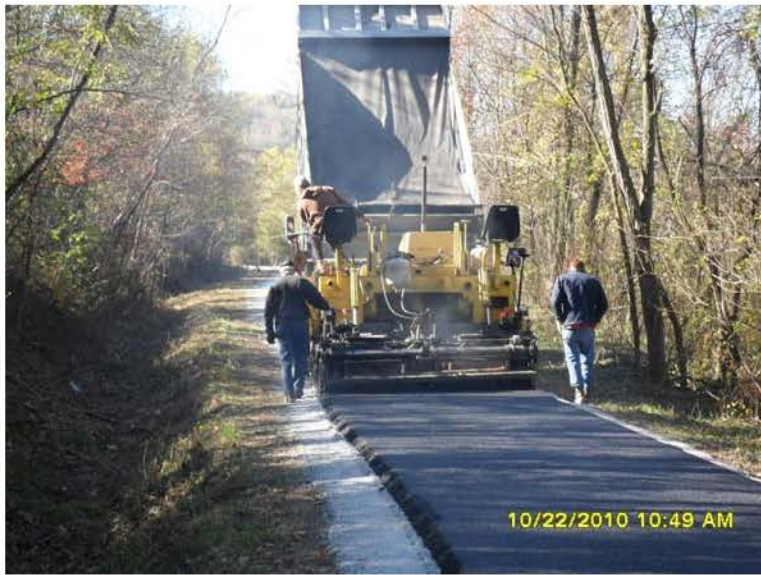
10/22/2010 Paving of trail. SAM_0041.JPG
