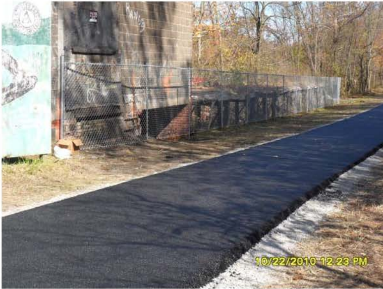
10/22/2010 Completed fence near building at trail head. SAM_0045.JPG
