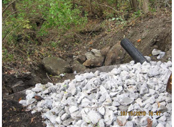
10/15/2010 Drainage swale area pipe with additional stone added for stabilization IMG_5543.jpg
