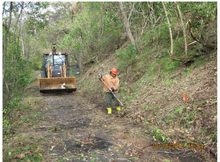
10/14/2010 ERRS crew clearing and gridding along RTT trail - looking north IMG_5515.jpg
