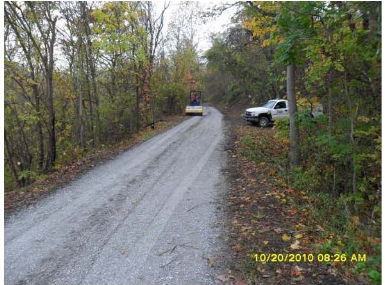
10/20/2010 ERRS compacting the recently added crush-n-run on the trail in preparation for agd\Uh SAM_0014.JPG
