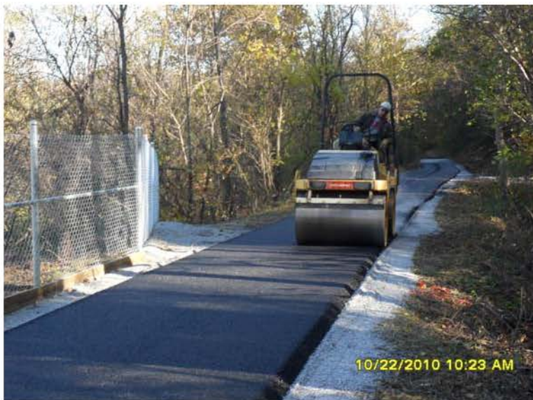
10/22/2010 Compaction on trail after asphalt was laid. SAM_0039.JPG
