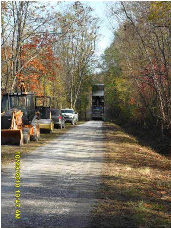
10/20/2010 Dump truck unloading and spreading crush-n-run on the trail. SAM_0021.JPG
