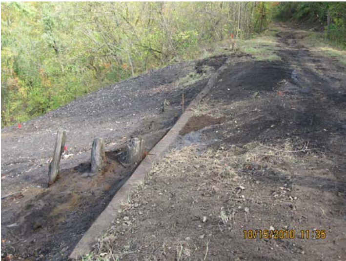
10/15/2010 Installed RR tie buttress system along slag pile area boundary IMG_5524.jpg
