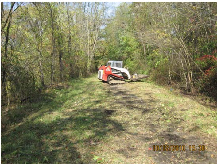
10/12/2010 ERRS skidsteer and mower deck performing brush clearing (N) IMG_5448.jpg
