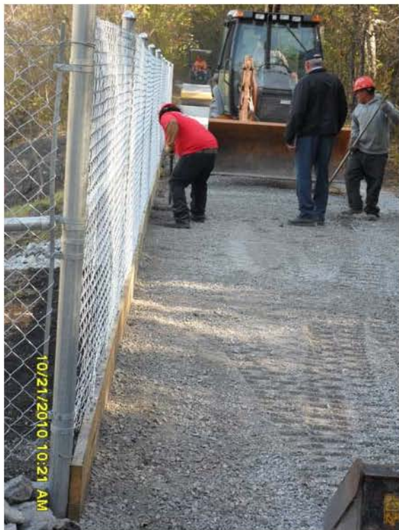
10/21/2010 In preparation for paving, ERRS placing crush-n-run on trail t... SAM_0027.JPG
