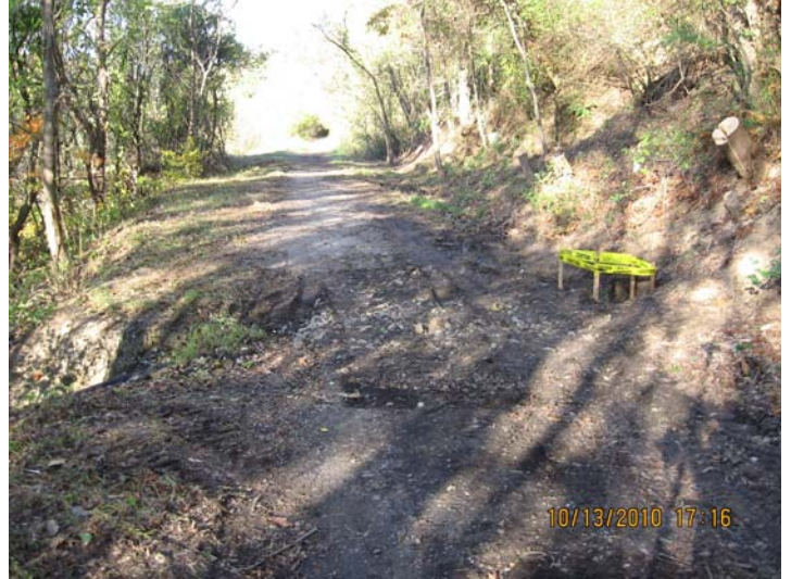
10/13/2010 Area along RTT trail where underflow drain pipe was installed IMG_5478.jpg
