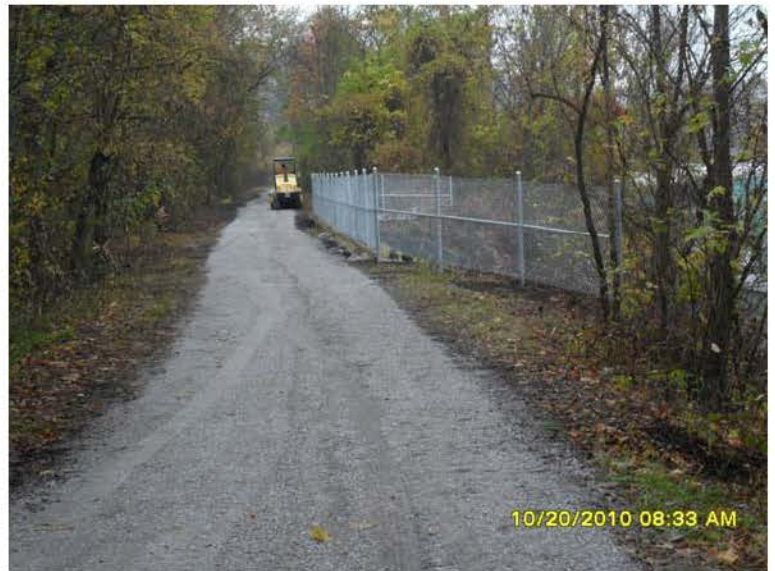
10/20/2010 View of the completed fence near the slag pile. SAM_0016.JPG
