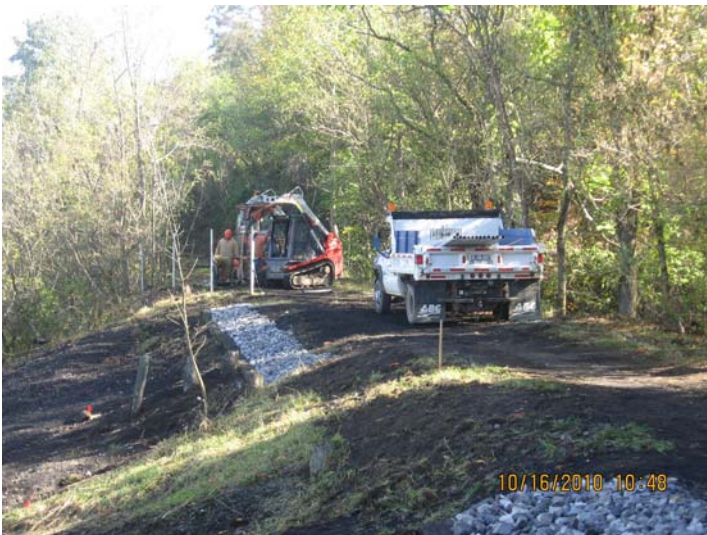
10/16/2010 ERRS crew installing fence in slag pile area looking north IMG_5544.jpg
