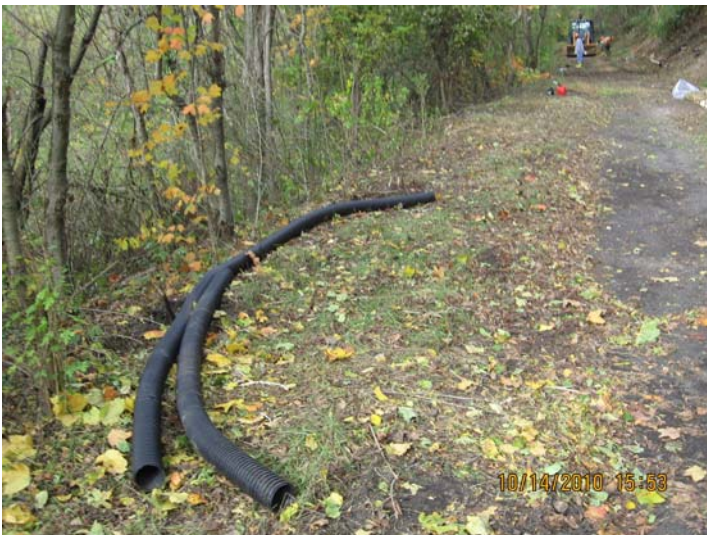
10/14/2010 Six inch CPP staged along RTT trail - looking north IMG_5507.jpg
