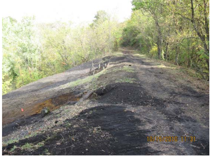
10/15/2010 Slag pile area with RR tie buttress installed - looking (N) IMG_5521.jpg
