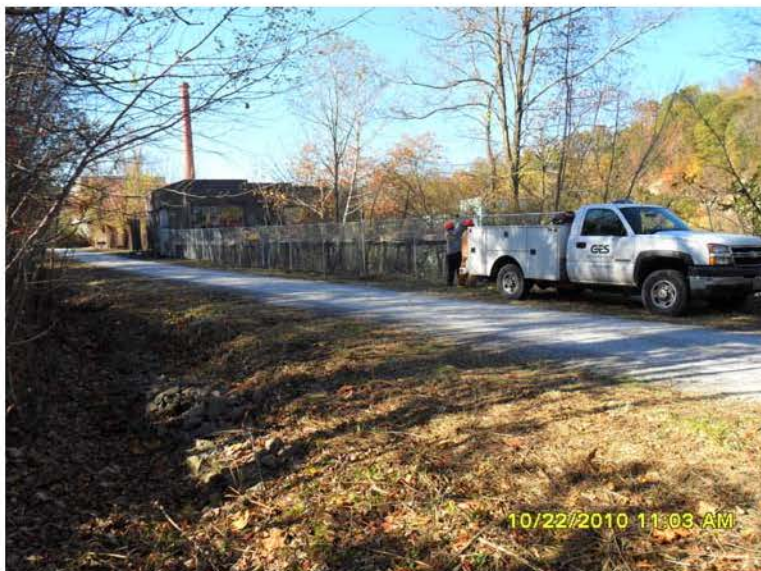
10/22/2010 ERRS erecting chain link fence near building at trail head. SAM_0043.JPG
