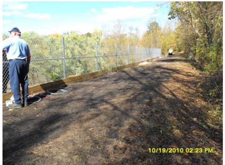
10/19/2010 Progress view of chain link fence. SAM_0012.JPG
