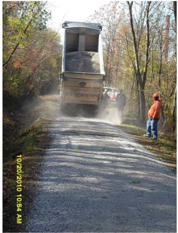
10/20/2010 Dump truck unloading and spreading crush-n-run on the trail. SAM_0022.JPG
