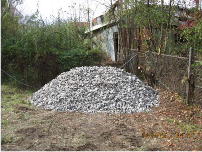
10/15/2010 Riprap stone staged near entrance to RTT trail - looking (S) IMG_5519.jpg
