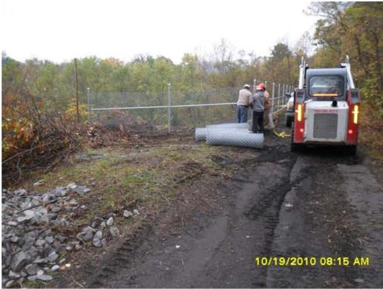
10/19/2010 ERRS erecting chain link fence. SAM_0009.JPG
