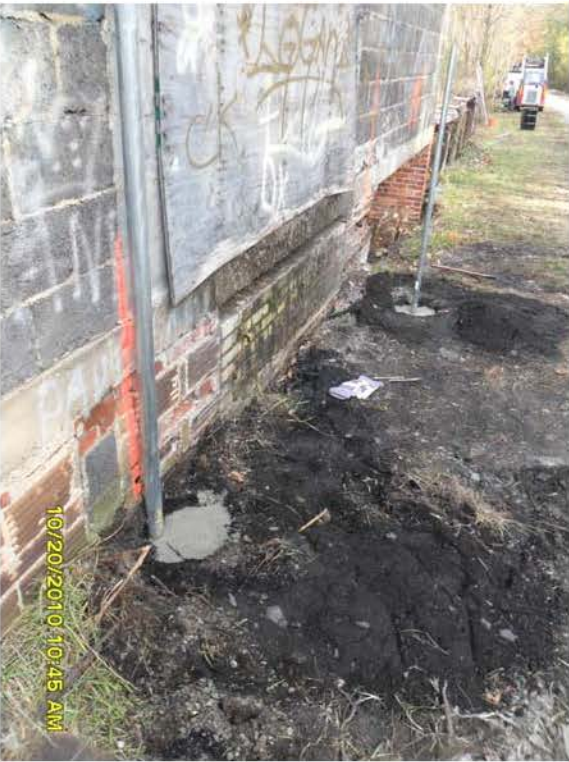
10/20/2010 Recently installed fence posts. SAM_0018.JPG
