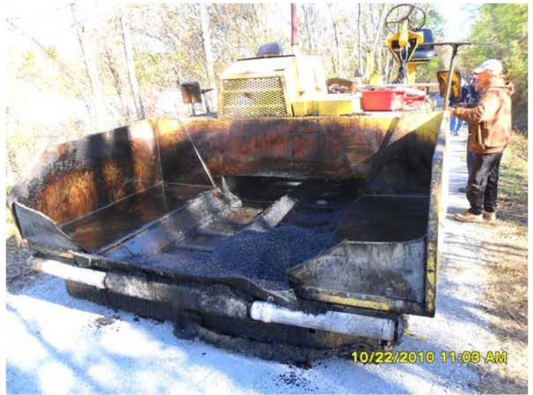
10/22/2010 View inside asphalt storage compartment. SAM_0042.JPG
