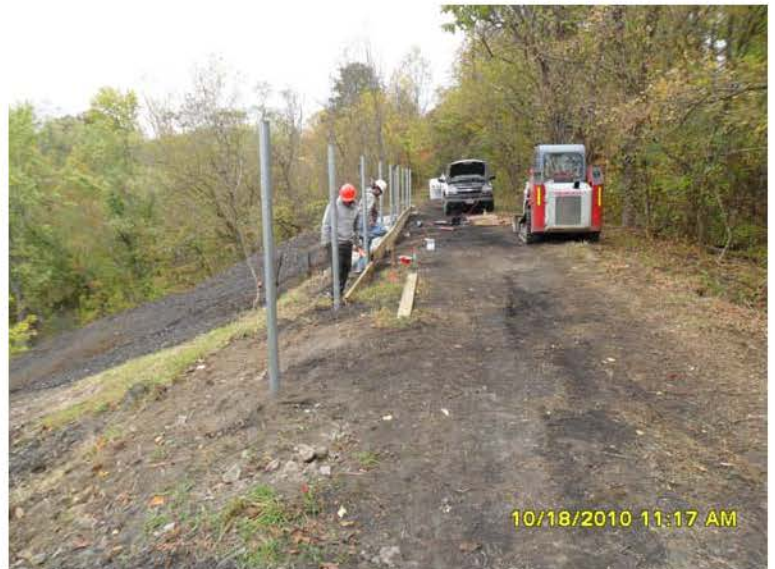
10/18/2010 ERRS installing wooden boards at base of fence. SAM_0003.JPG
