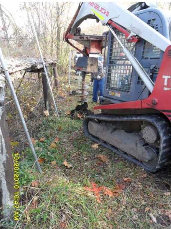
10/20/2010 ERRS using skidsteer with an auger attachment to dig the SAM_0020.JPG
