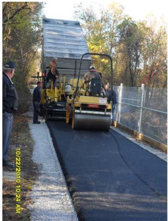
10/22/2010 Compaction on trail after asphalt was laid. SAM_0040.JPG
