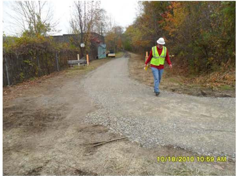
10/18/2010 View of gravel base compacted on trail. SAM_0001.JPG
