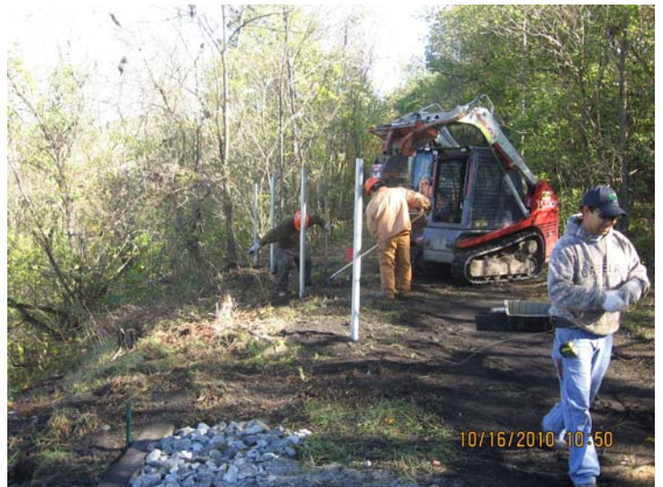
10/16/2010 ERRS installing fence posts in slag area looking north IMG_5546.jpg
