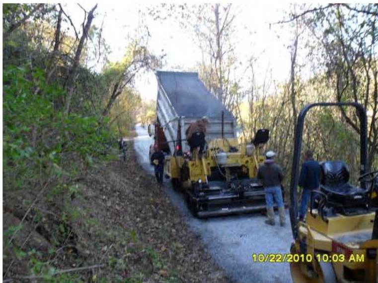
10/22/2010 Dump truck unloading asphalt into the paving machine. SAM_0034.JPG
