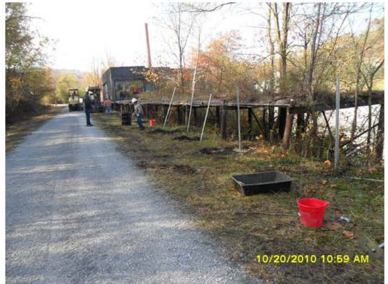
10/20/2010 ERRS installing fence posts. SAM_0024.JPG
