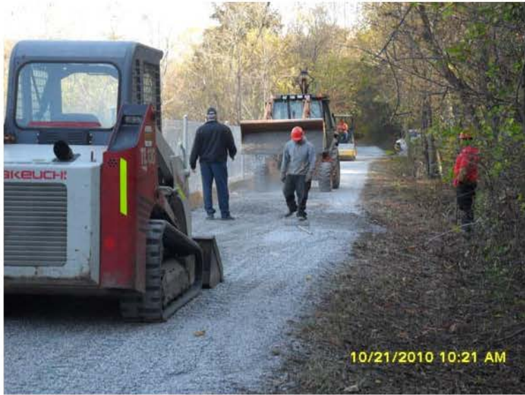
10/21/2010 ERRS placing crush-n-run on trail to fill to level it in preparation for paving. SAM_0025.JPG
