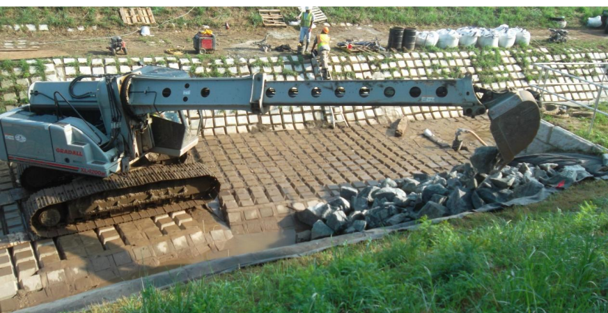
Top Left: Temporary pumps and a sandbag dam were installed to create a dry work area for rebuilding Rose Valley Creek. Upper Middle: Stream water was re-routed through 700 feet of piping and discharged into Wissahickon Creek while Rose Valley was being widened and lined. Lower Middle: Before geotextile and cabled concrete mats (CCM) were laid, workers placed a layer of stone on the floor of Rose Valley Creek. Bottom Left: For added security, rip rap was placed over the CCM on the stream embankment. Top Right: Rose Valley Creek after being repaired and widened to reduce future flooding.
