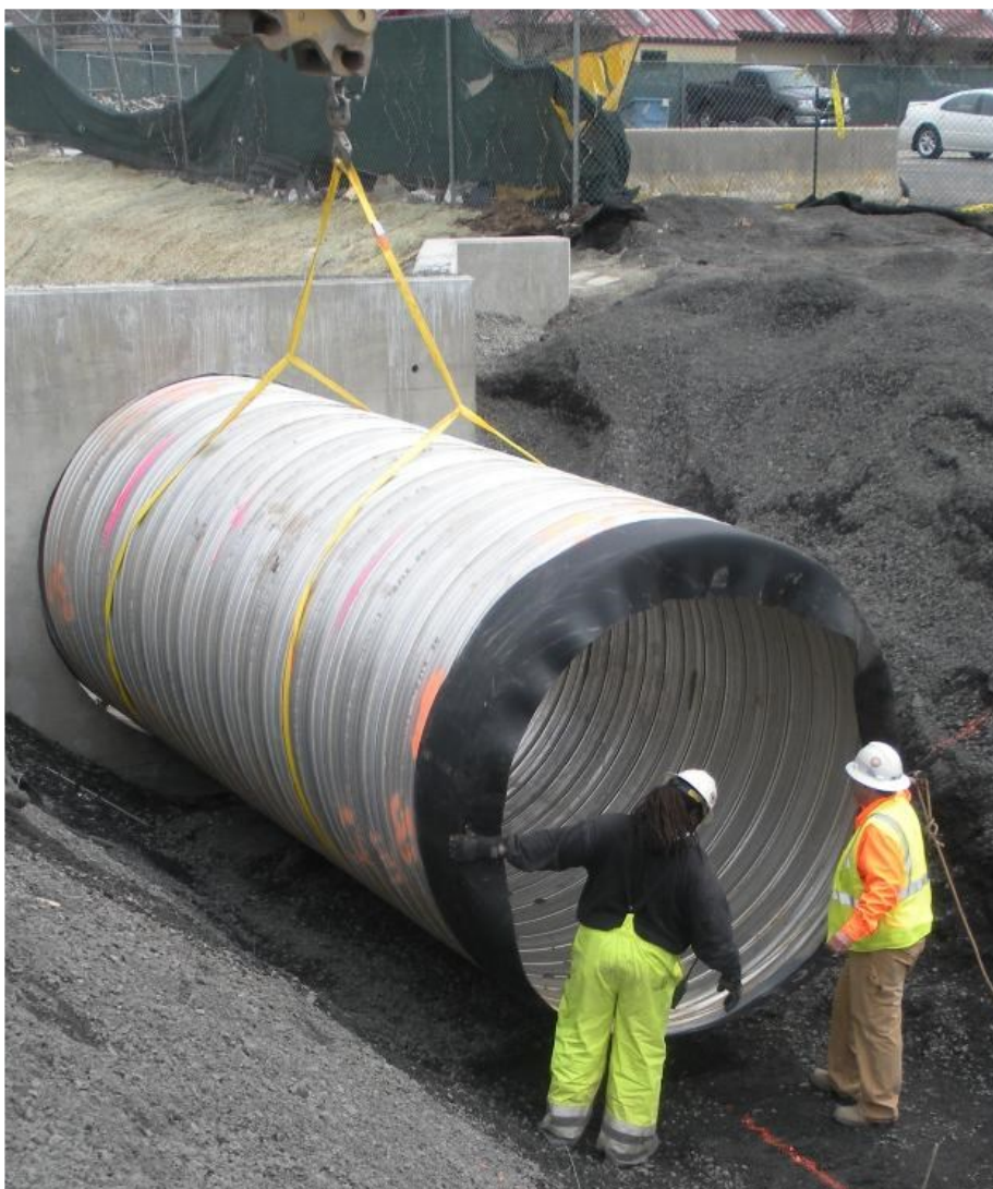
The 25-ft.-high embankment of Tannery Run, behind Butler Street businesses, was eroding and destabilizing parking lots. EPA enclosed a 325-foot portion of the stream to prevent collapse. Top Left: Crew installs the headwall to anchor the 8-ft-diameter pipe through which the stream will flow. Top Right: Water will flow from the lined open channel into the 8-ft. diameter pipe at the headwall. Bottom Left: Workers install first section of 8-ft-diameter pipe. Bottom Right: Liner and pipe were covered with 2,640 cubic yards of stone; the enclosed area was finished with soil and seeded.
