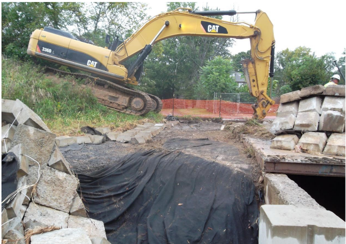
Upper Left: During Tropical Storm Lee, water and debris burst through the old sluice gate at Maple Ave., sweeping down Rose Valley Creek and destroying the recently installed cabled concrete mats (CCM). Although a setback, the experience helped EPA and the US Army Corps of Engineers to improve and strengthen the stream liner system. Lower Left: Contractor conducting CCM repair after the storm. Upper Right: Restored and strengthened stream liner at Rose Valley Creek headwall. Lower Right: A new swing-gate was installed at Maple Avenue/Rose Valley Creek sluiceway. The gate is designed to release water slowly during future storm events.
