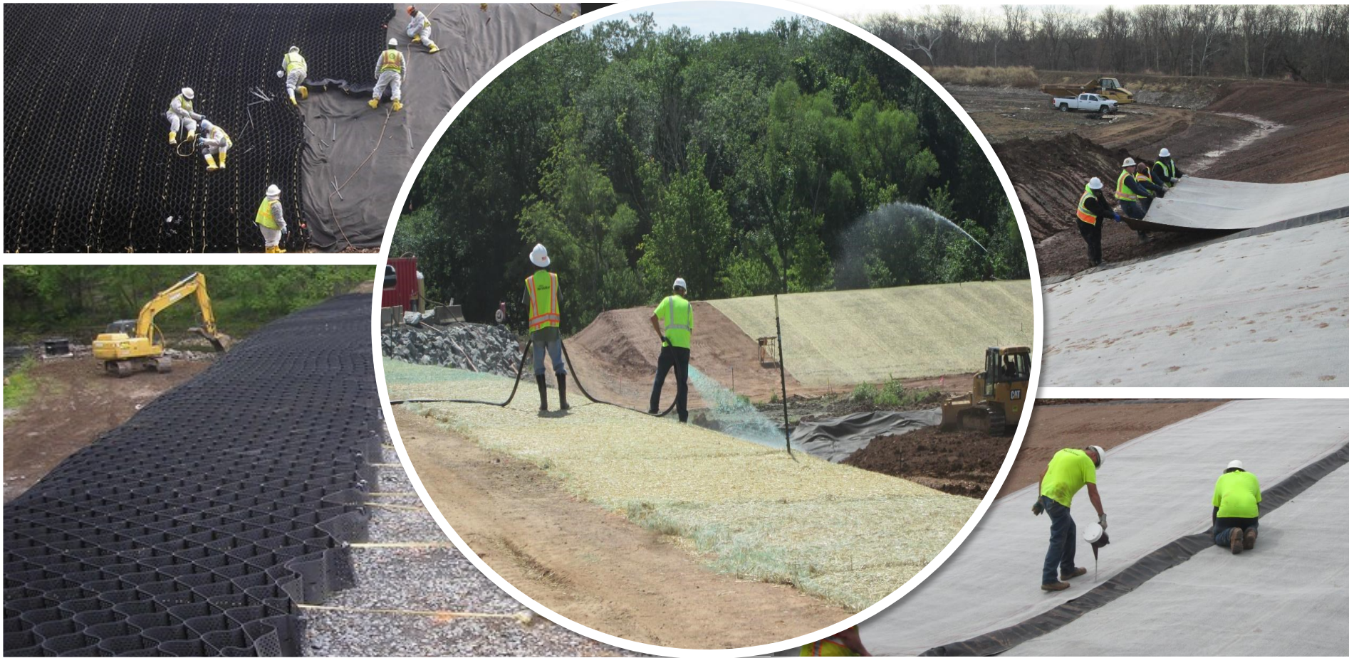
Geotextile was laid over the entire 32-acre site. Additional components of the cap were layered over the textile. Top Left: Workers secure high-density polyethylene geocells resembling a honeycomb over geotextile on a steep embankment of the Wissahickon. Bottom Left: A crane was used to fill geocells with stone. Soil was later placed over the geotextile and geocells and seeded. Top Right: Workers place geosynthetic clay-impregnated liner (GCL) on an inside section of the pond berm to increase structural stability. Bottom Right: Workers pore bentonite along the seams of the clay liner. Center: Workers hydro-seeding berm. Straw mats prevent erosion and help seeds to sprout.
