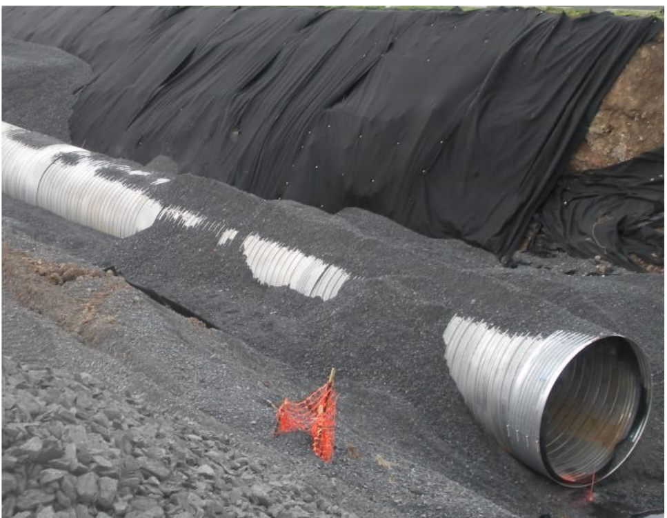
The 25-ft.-high embankment of Tannery Run, behind Butler Street businesses, was eroding and destabilizing parking lots. EPA enclosed a 325-foot portion of the stream to prevent collapse. Top Left: Crew installs the headwall to anchor the 8-ft-diameter pipe through which the stream will flow. Top Right: Water will flow from the lined open channel into the 8-ft. diameter pipe at the headwall. Bottom Left: Workers install first section of 8-ft-diameter pipe. Bottom Right: Liner and pipe were covered with 2,640 cubic yards of stone; the enclosed area was finished with soil and seeded.
