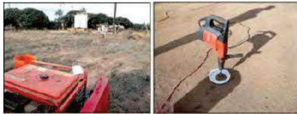
Figure F-12. High-Powered Drill and Portable Generator.
