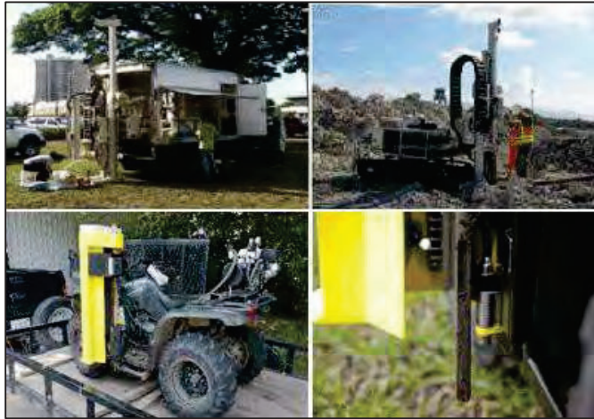
Figure G-2. Direct push drill rigs.
