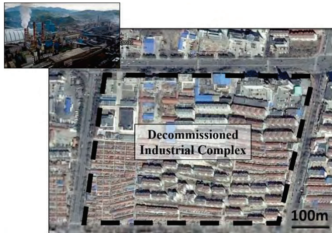
Figure C-22. Former industrial complex proposed for demolition and redevelopment for residential housing.
