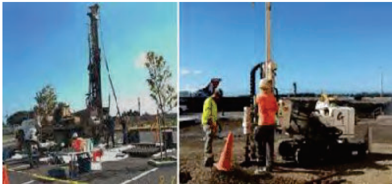
Figure G-11. Hollow-stem auger drill rig.
