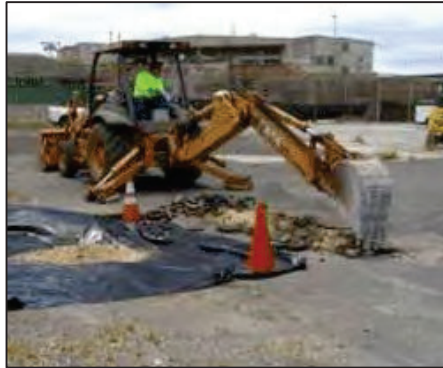
Figure G-9. Use of trenches for site investigation to identify the presence and approximate thickness of known, lead-contaminated fill at strategic locations across a site.
