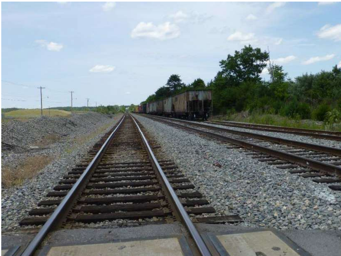
The Norfolk Southern rail line that runs north-south through the center of the Site
