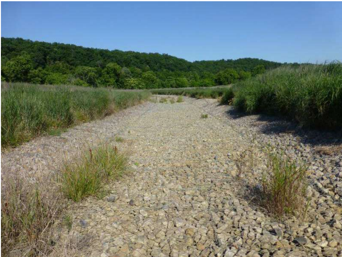
Stormwater discharge culvert from SB 2
