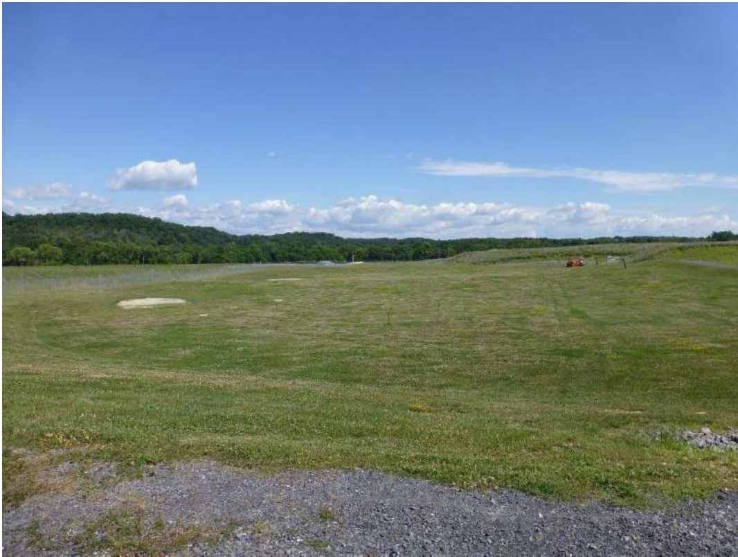
View of VB 9, looking northwest. The PRP is aware of the two bare low spots (shown on the left side of the photo) and plans to address the areas in the fall of 2017
