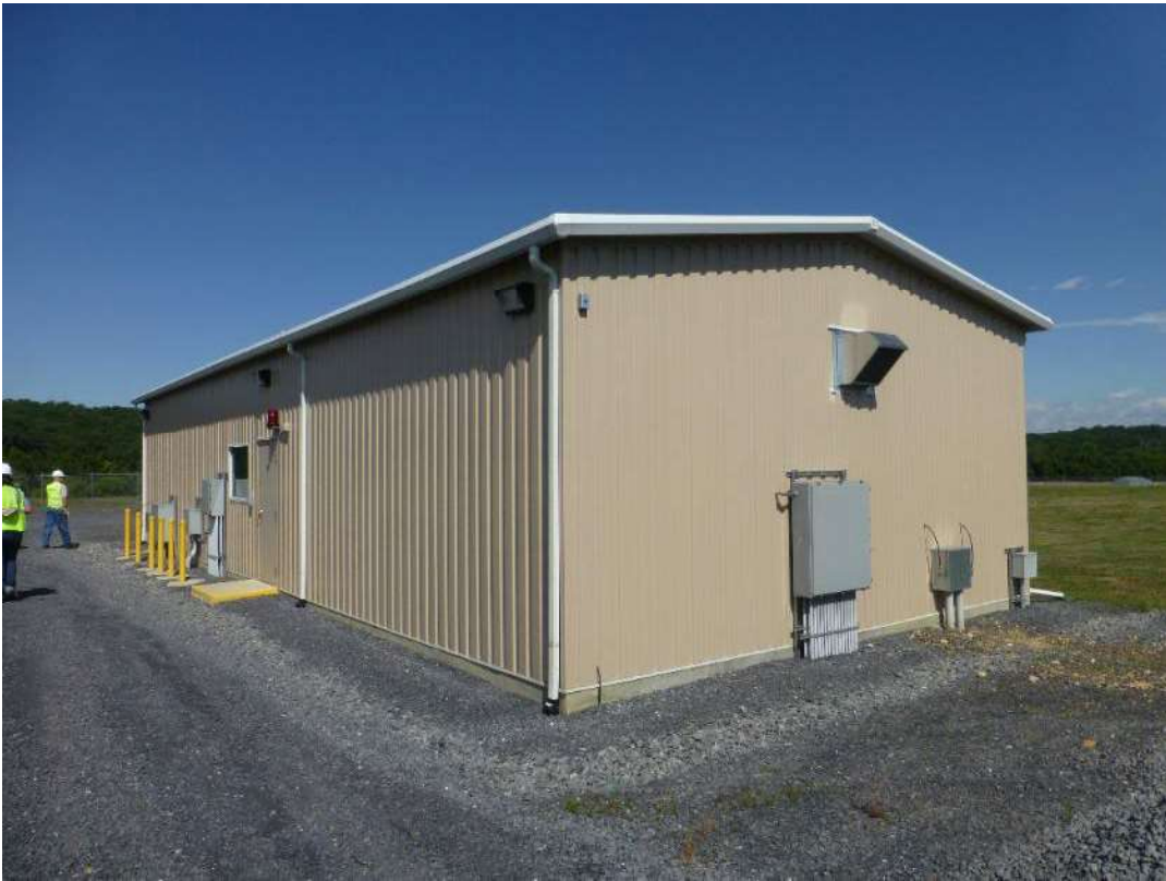
Exterior of the VB extraction equipment building
