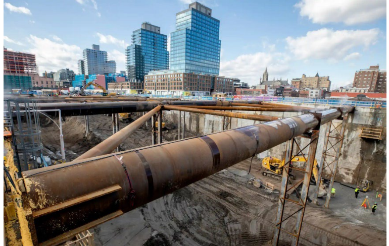
Structural support within the 8-million-gallon CSO tank
