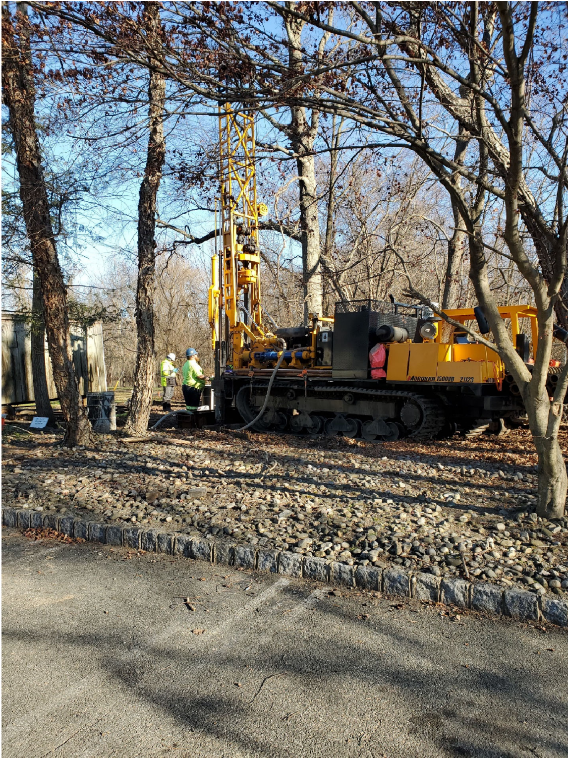
Installation of Monitoring Well 31 I – 12/20/23
