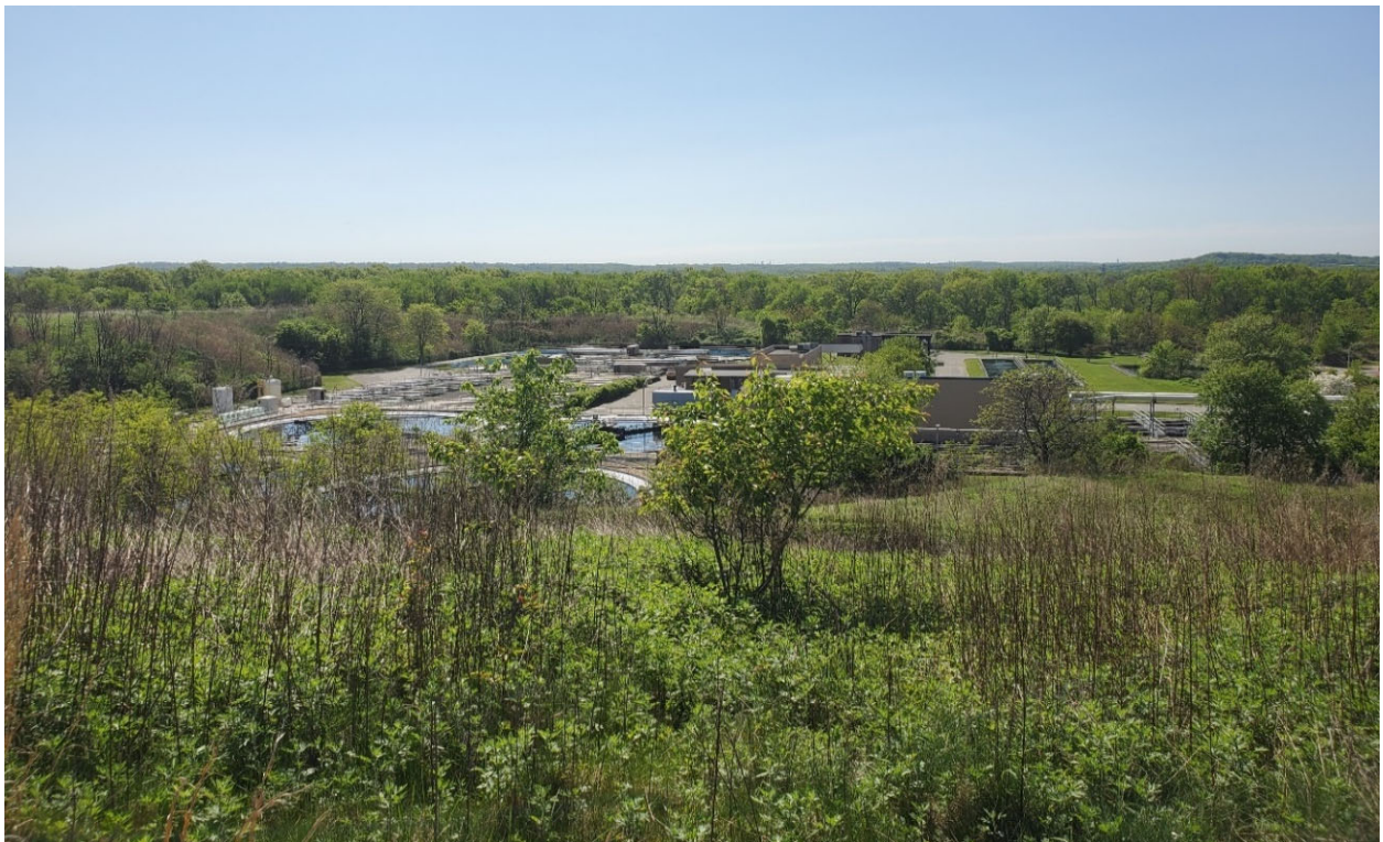
South Fill Area/Parsippany-Troy Hills Wastewater Treat Plant – 5/7/24
