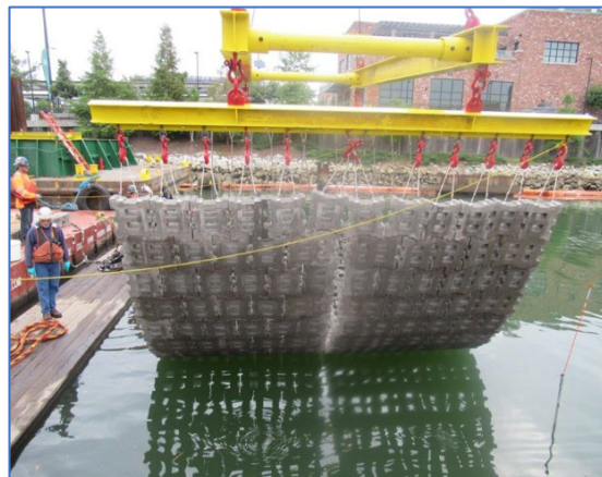
Articulated concrete mat being placed in 4 th Street Turning Basin
