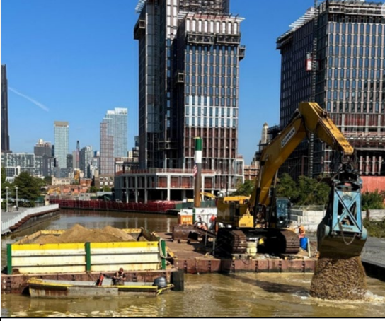
Capping material being placed in Gowanus Canal
