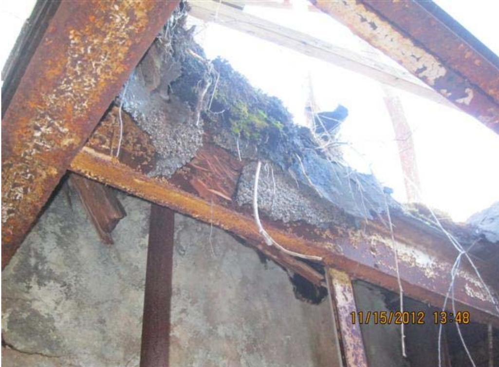
View of the SACM roofing material from the boiler room catwalk at Area F2.
