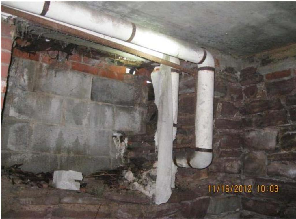
View of the asbestos pipe insulation identified at the Area C basement.
