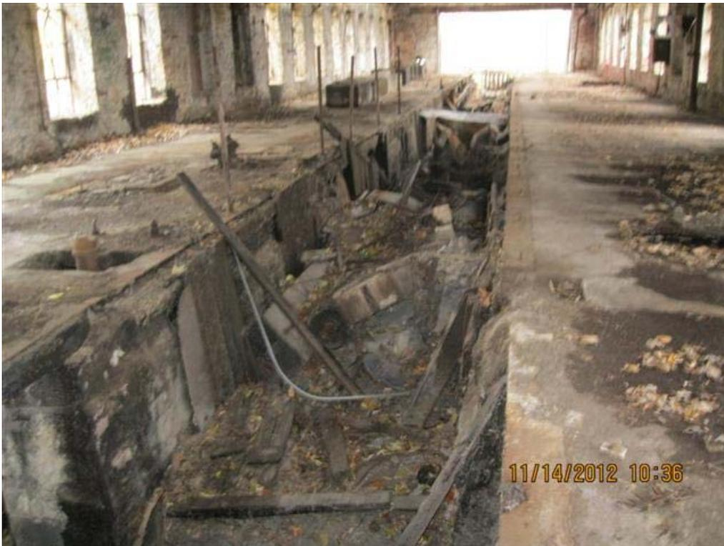
View facing north of the collapsed area at the main floor at Building E.
