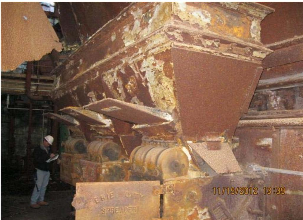
View of the deteriorated Boiler at Area F2. Note the ash piles on equipment.
