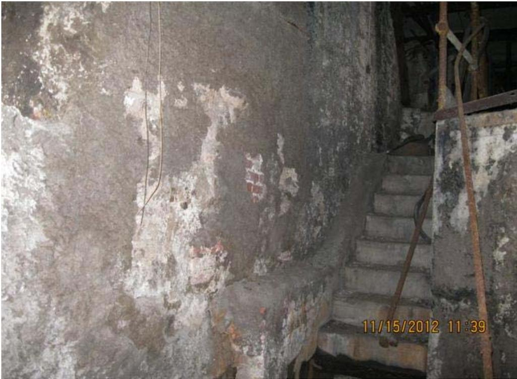
View of the lint/process fluff on the wall at the basement of Area D.
