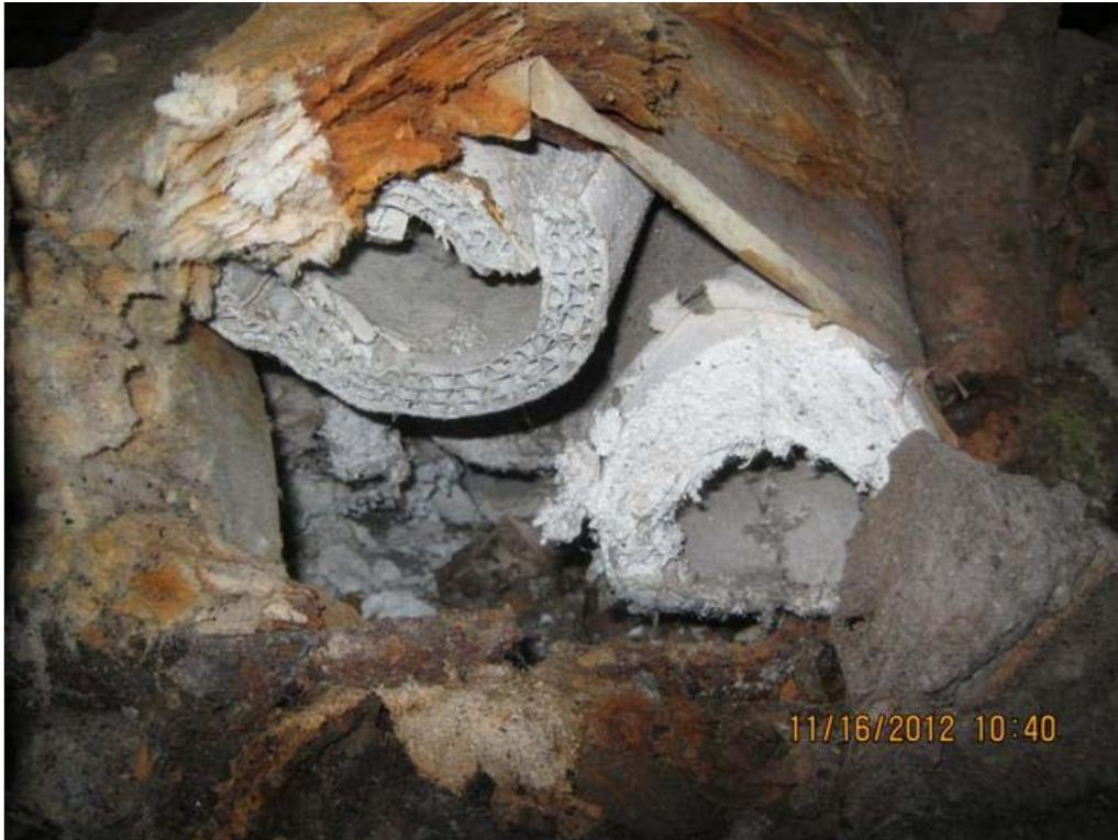
Close-up view of the asbestos pipe insulation in the deteriorated drum at the Area C basement.
