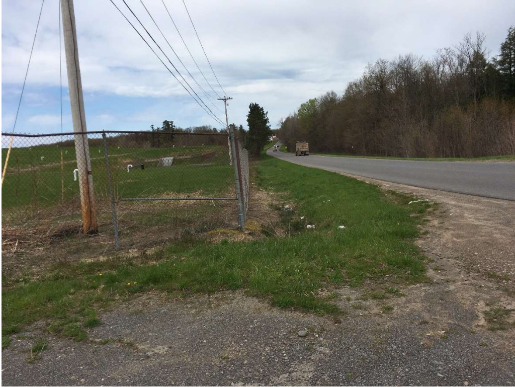
Photo of Eastern Perimeter Fence Facing North
