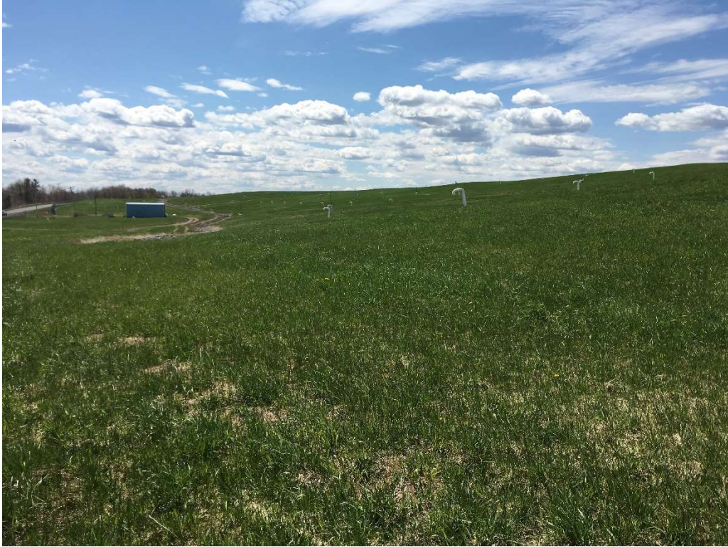
Photo of Eastern Side Slope Facing South
