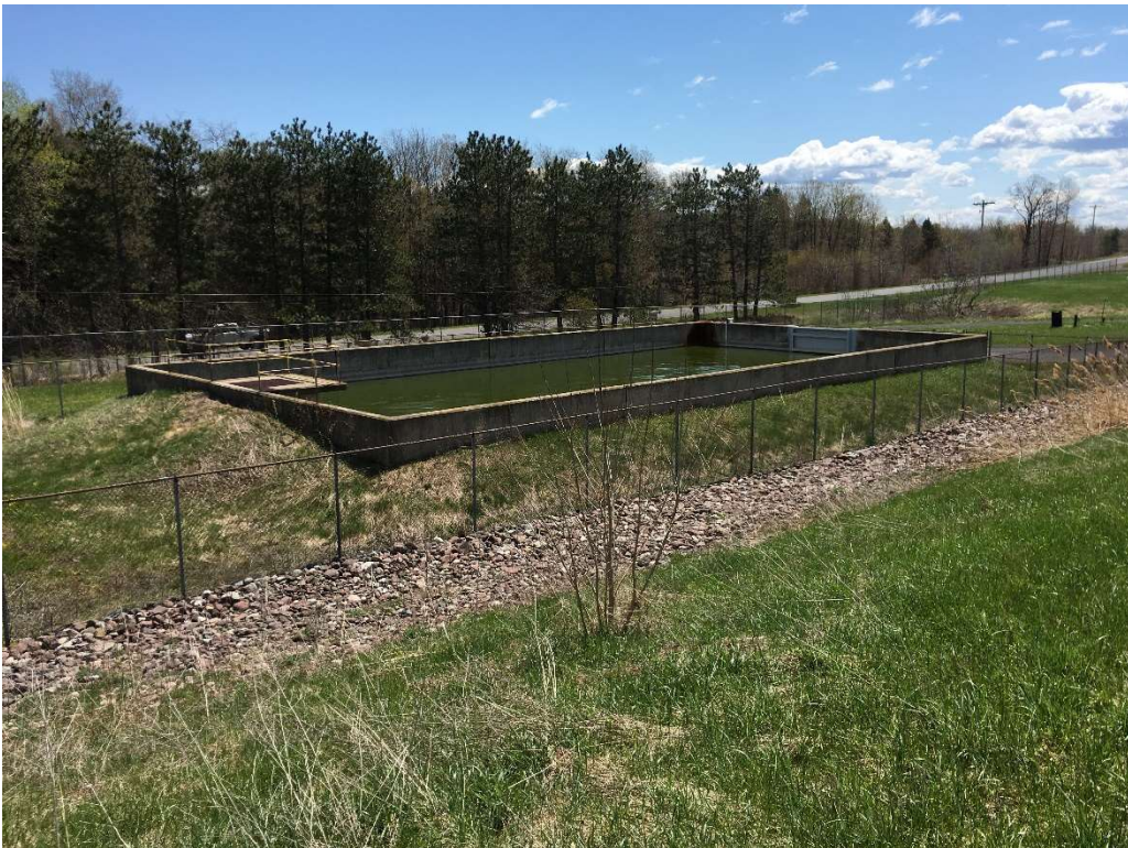
Photo of On-site Leachate Storage Structure
