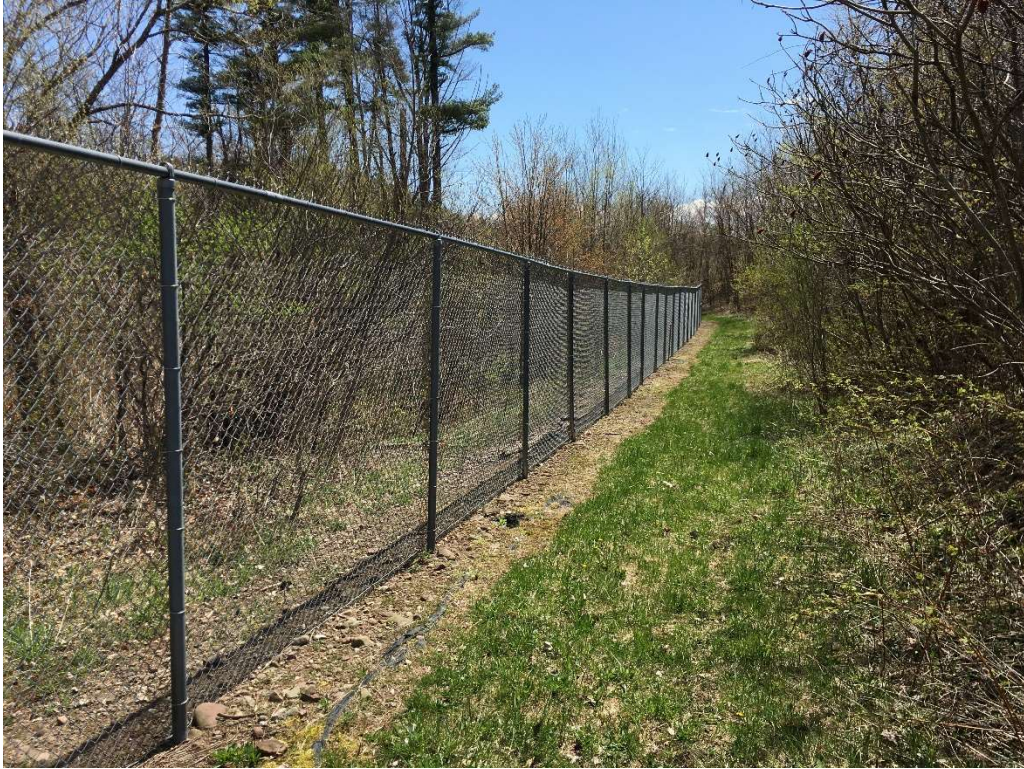
Photo of Northern Perimeter Fence Facing East
