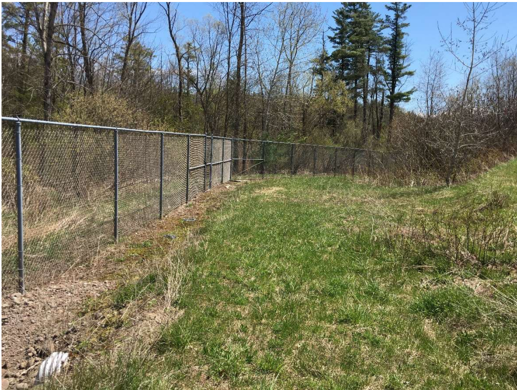
Photo of Northern Perimeter Fence Facing East
