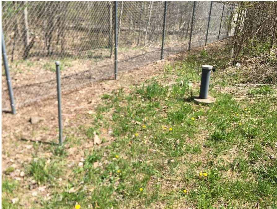
Photo of Perimeter Monitoring Well – North Side
