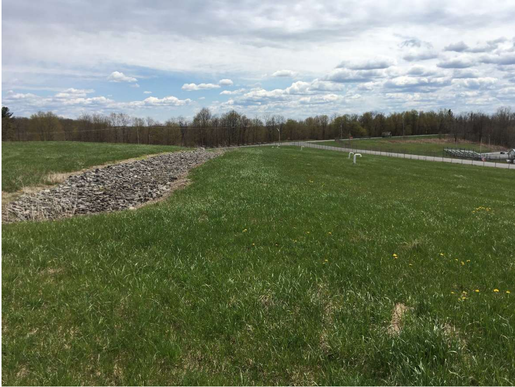
Photo of Southeast Downchute
