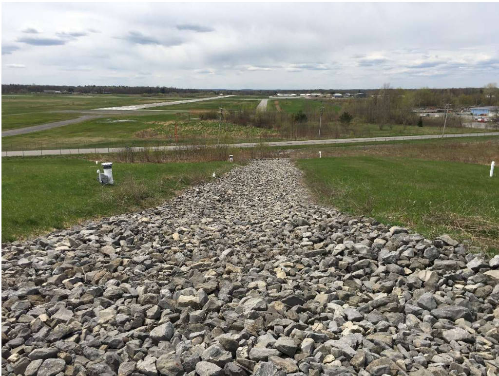
Photo of Southern Downchute
