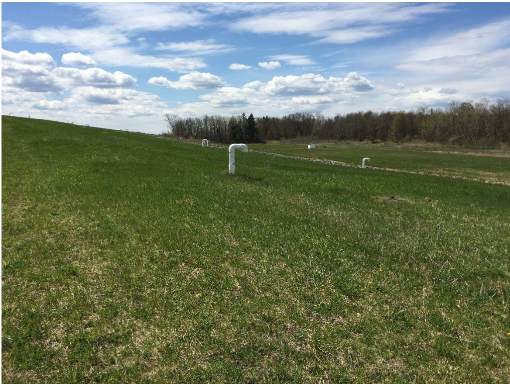
Photo of Western Side Slope Facing South
