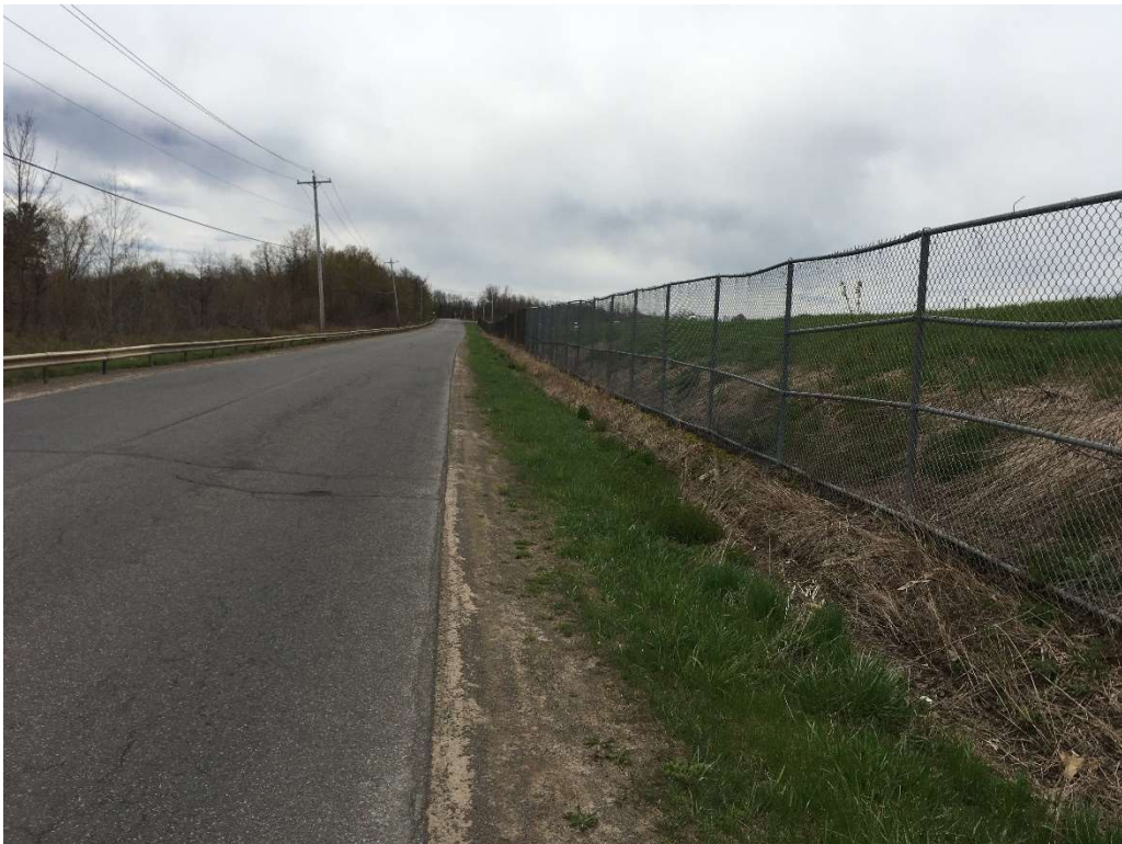
Photo of Eastern Perimeter Fence Facing South
