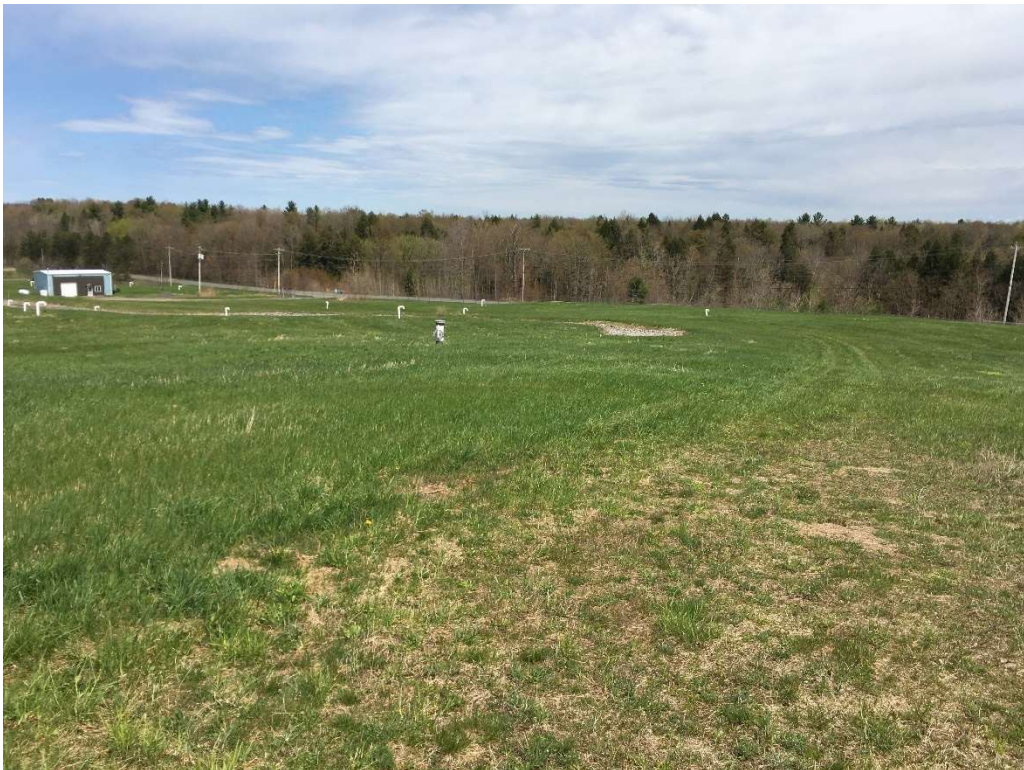
Photo from Top of Cap Facing East
