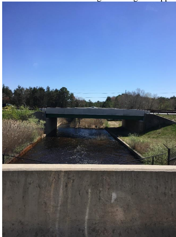
View downstream of Upper Reservoir spillway, looking east towards Lower Reservoir
