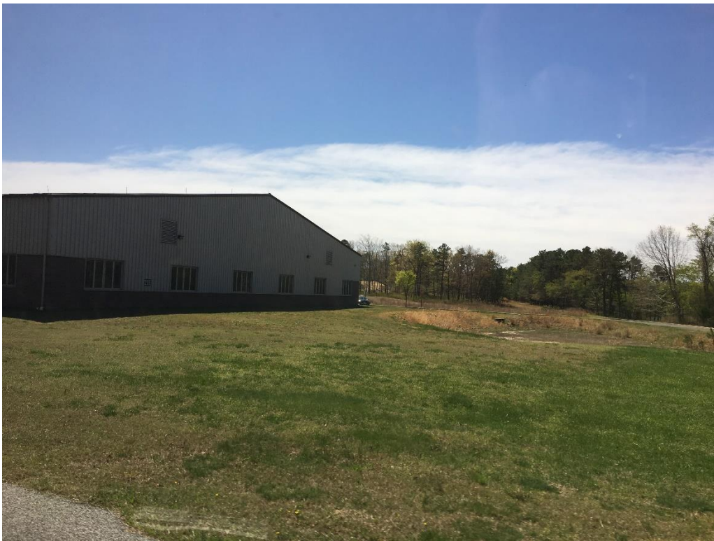
OU09 - Area A, looking southeast from Card Road
