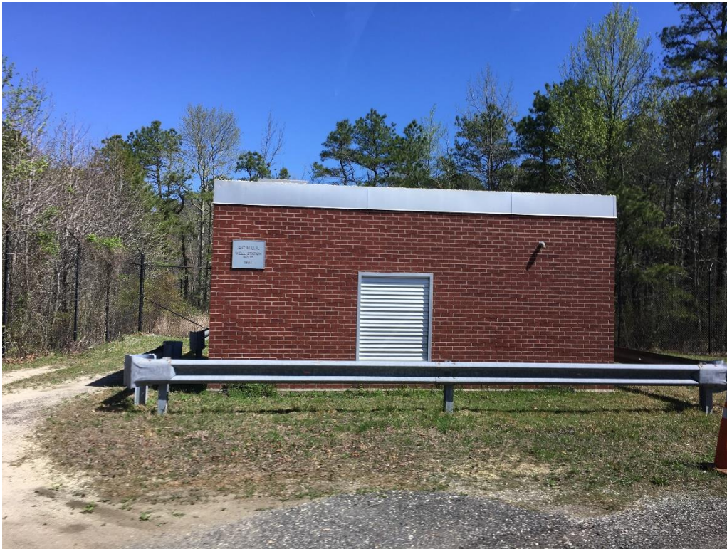
Typical ACMUA well location along north edge of Upper Reservoir
