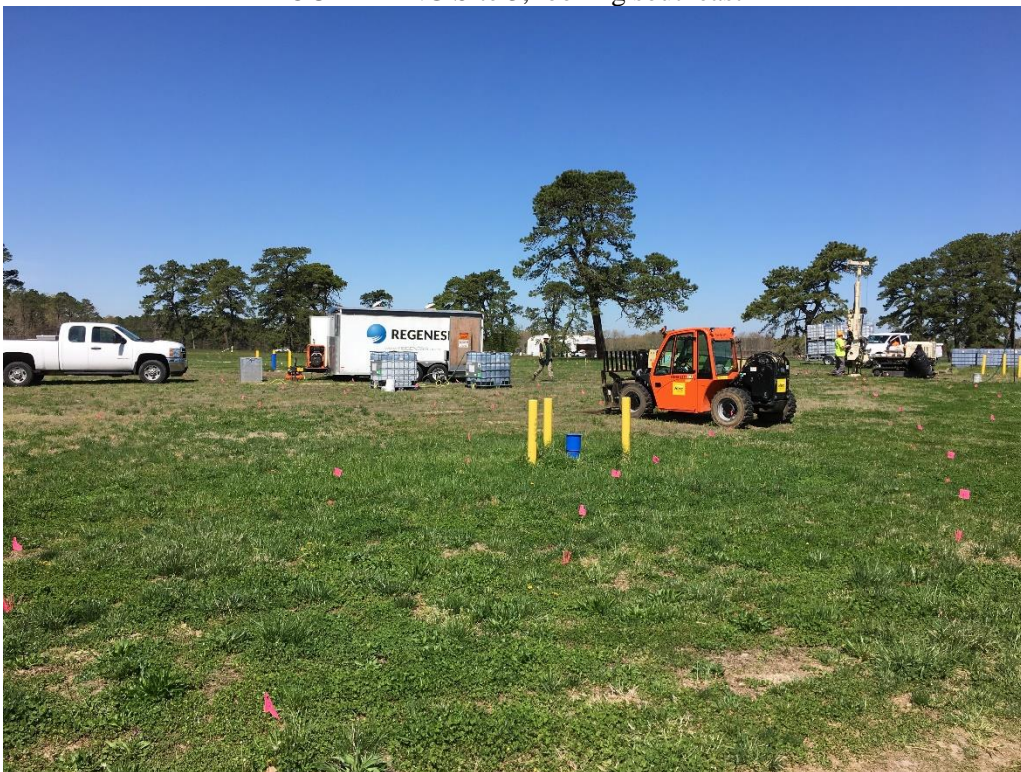
OU13 - Area E In Situ Adsorption injections, looking northwest
