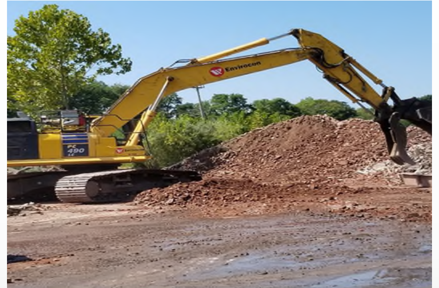
Crushing brick with backhoe attachment
