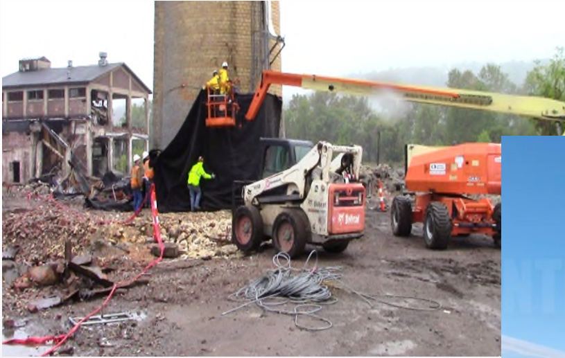
Wrapping brick stack w/explosives
