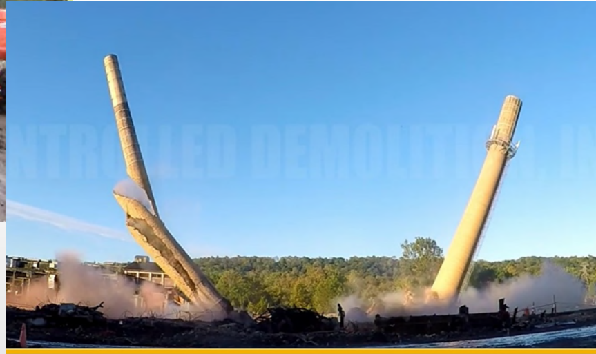
Brick stacks being felled
