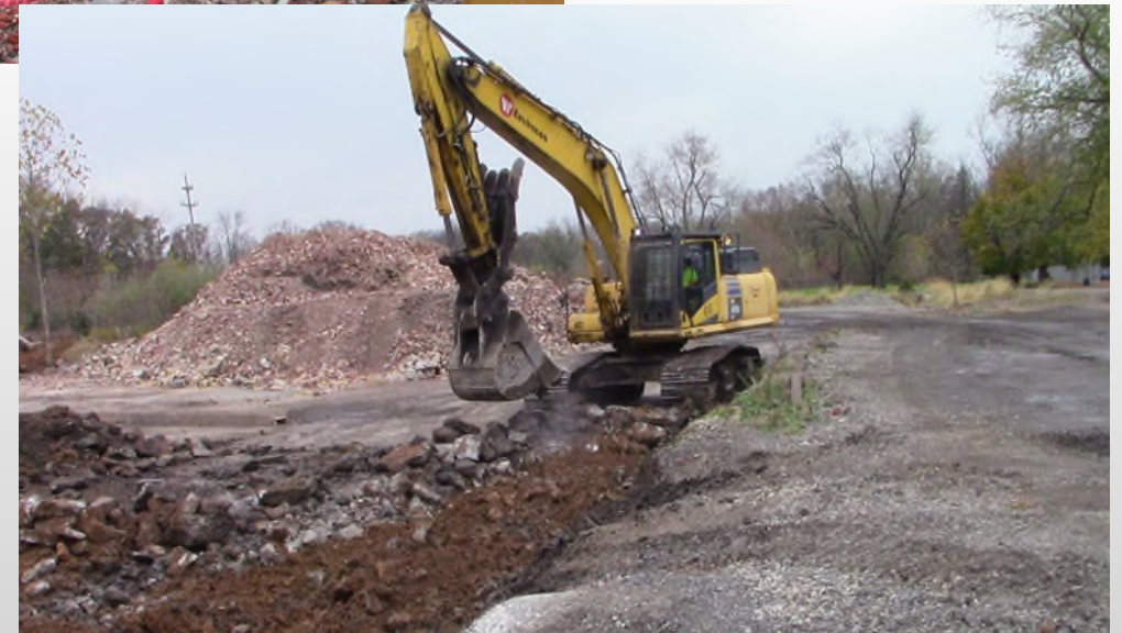
Removing Building 1/50 slab
