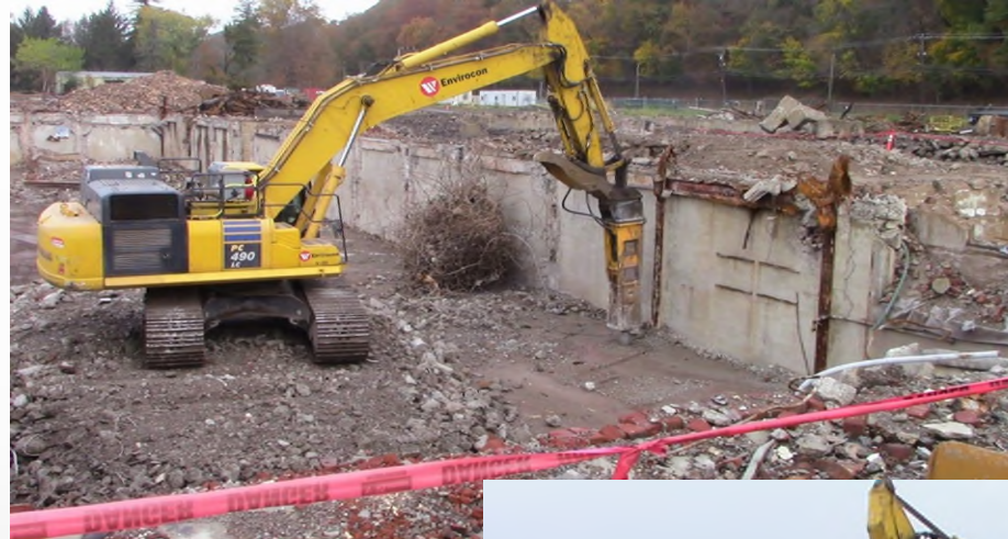
Perforating slabs in Group B
