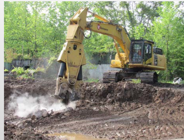
Removal of Residual Concrete Building 83B
