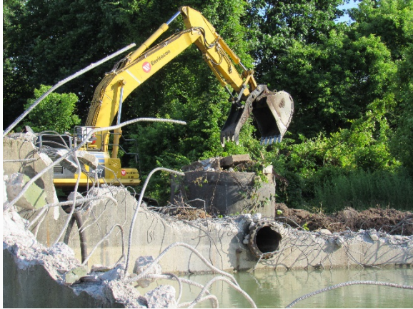
Demolition of Clarifier
