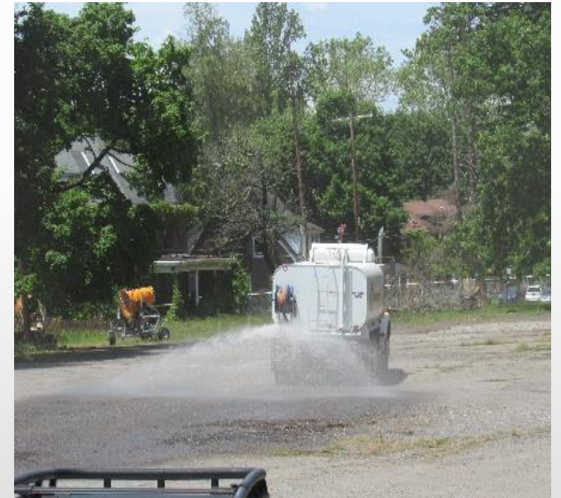
Water truck being used to provide dust suppression
