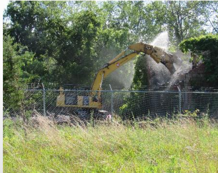
Demolition of Building 126 with dust suppression from behind building
