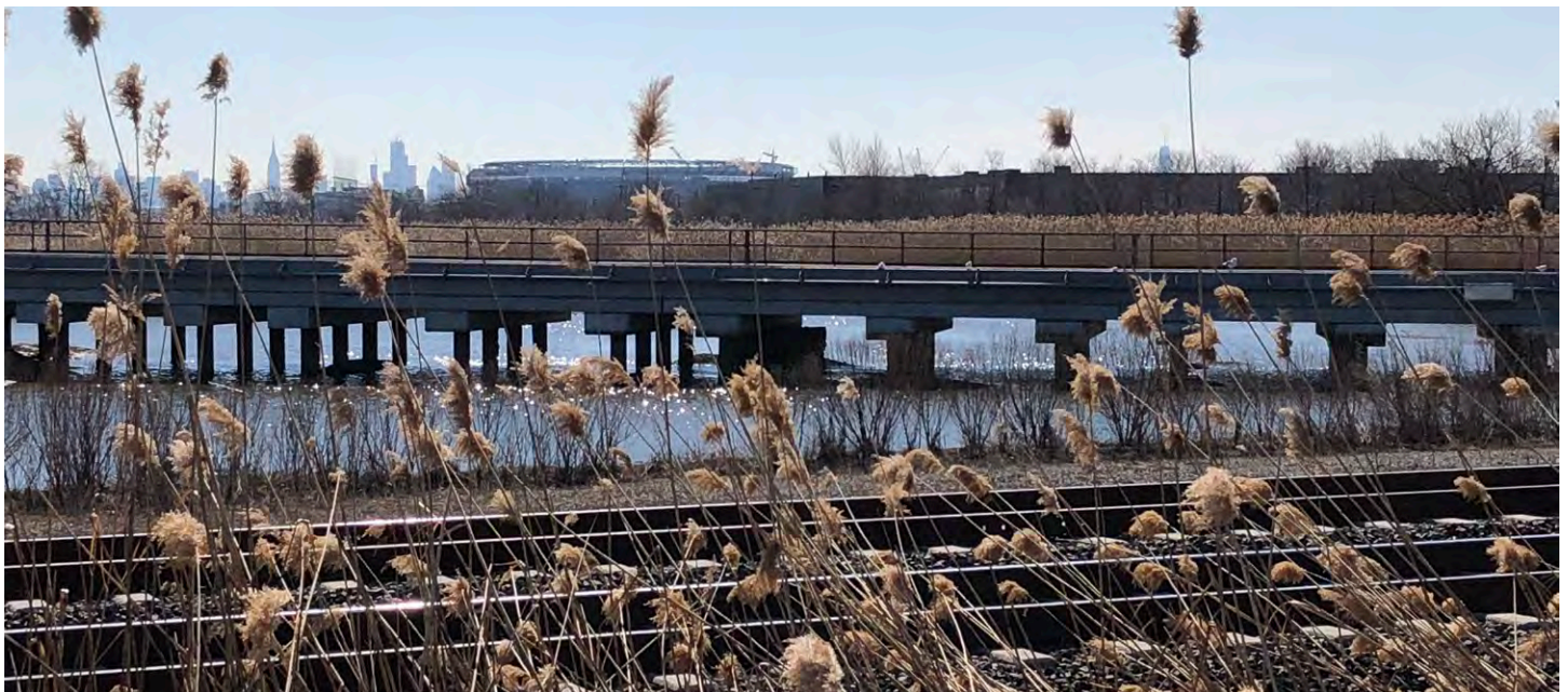
VIEW OF THE LAGOON IN UOP PROJECT AREA POST-NTCRA CONSTRUCTION, FACING EAST
