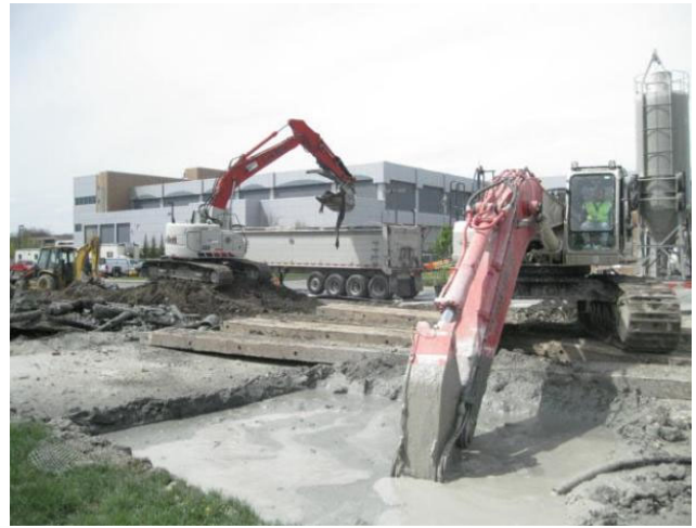
In-Situ Soil Solidification/Stabilization (ISS) by Excavator Mixing
