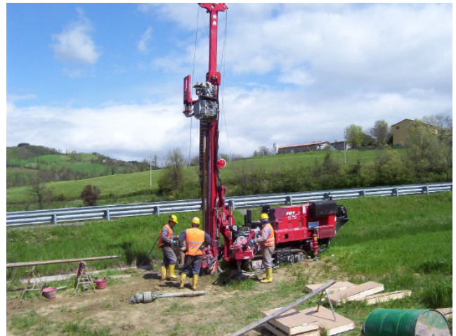
Drill Rig for Jet Grouting
