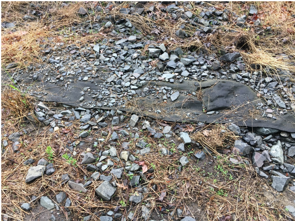
Riprap liner found to be exposed in the southern portion of the rip rap
