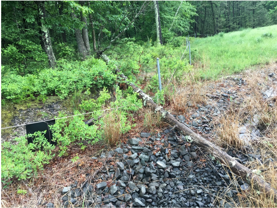
Fallen tree on south portion of cable fence at Site 3
