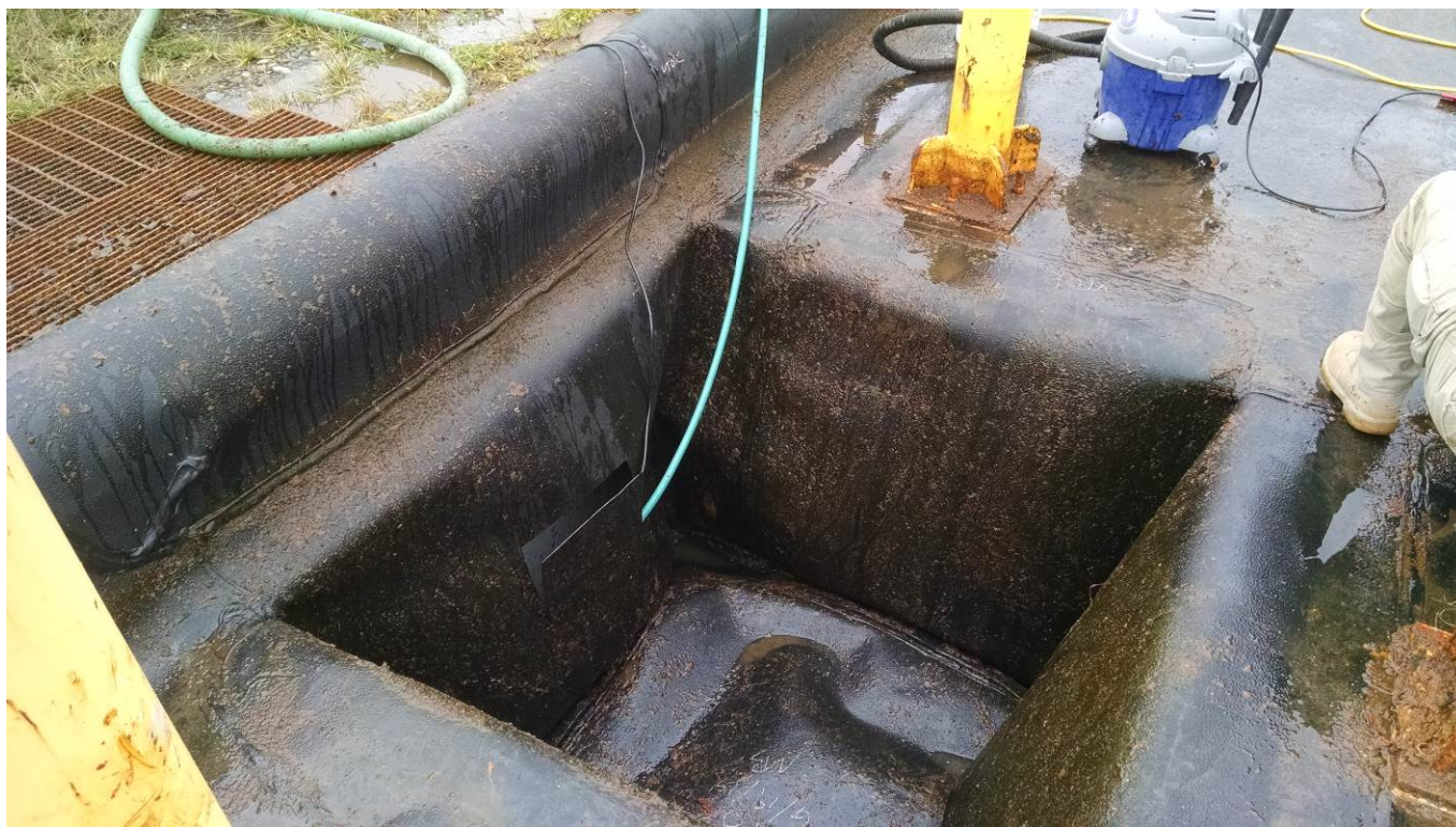
5 – December 16, 2015: Removal of water beneath HDPE cover in sump
