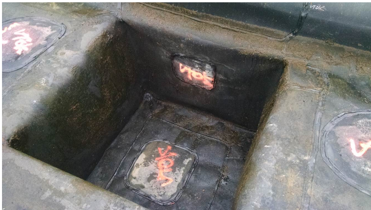
11 - December 16, 2015: Sample Location 6 Sump base (see also additional vertical repair used to remove water below sump)
