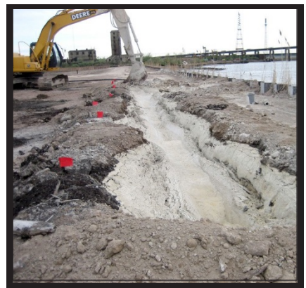
Slurry Wall Installation
