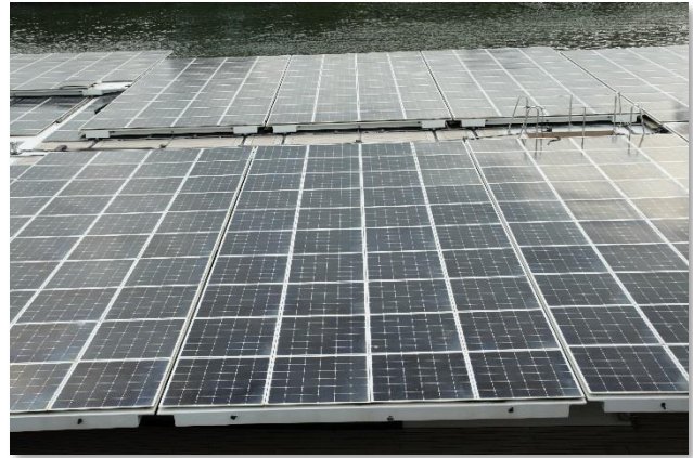
Figure 6. Rooftop solar arrays can provide energy cost savings.
