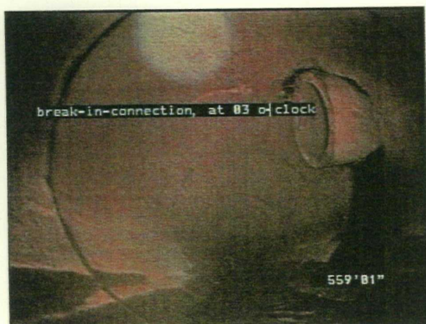
IMAGE: 15a, TAPE #: 01, 00:00:00 559.1FT, break-in-connection, at 03 o'clock
