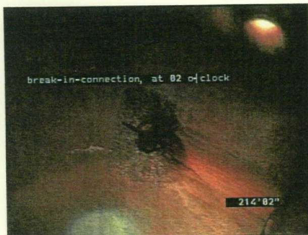
IMAGE: 6a, TAPE #: 01, 00:00:00 214.2FT, break-in-connection, at 02 o'clock
