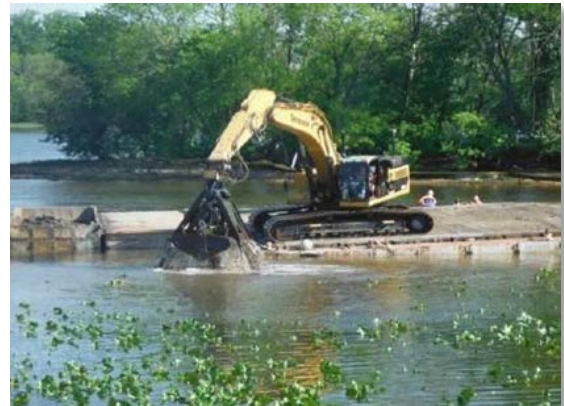
Figure 3. Dredging activities during OU5 cleanup.
