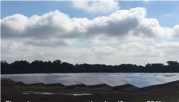
The solar power array on the site. (Source: EPA)
