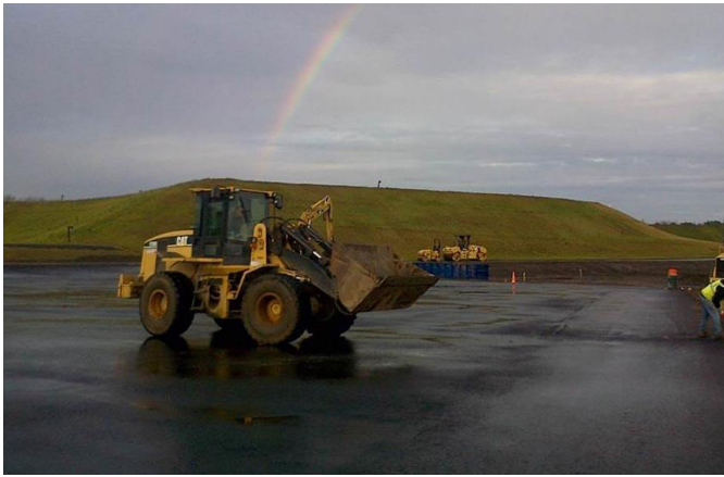
Nearing the completion of landfill cap construction in 2012.
