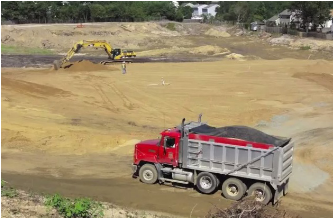
Construction underway on the landfill cap in 2011.
