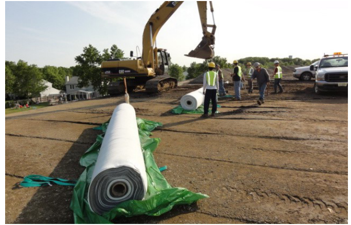
Preparing to unroll the geosynthetic clay liner.
