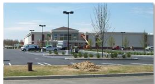
Figure 5. A monitoring well between parking areas in front of the Stop & Shop.
