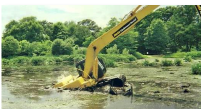
Figure 3. Cleanup included ground water treatment and soil and sediment removal. (Source: EPA and Nassau County websites)
