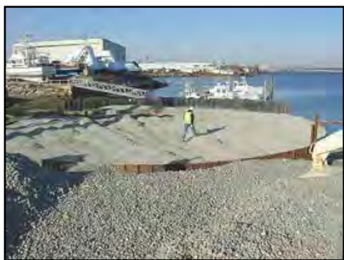
Construction of the Marine Bulkhead
