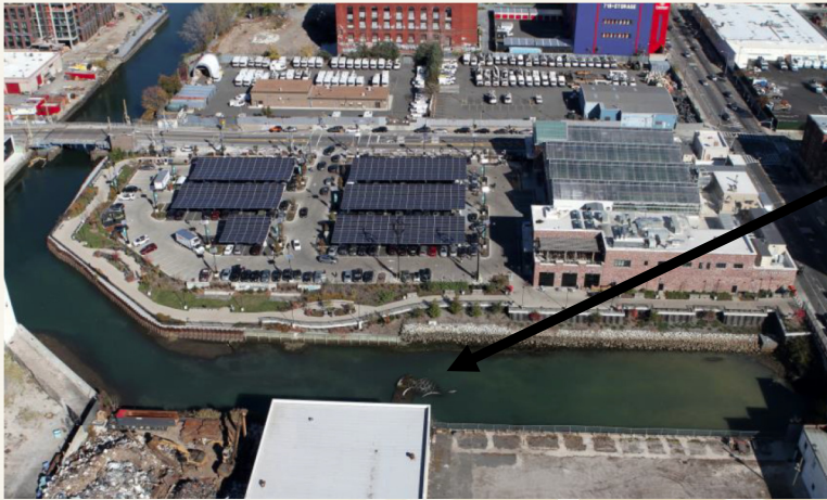
Overhead view of the 4 th Street turning basin.
