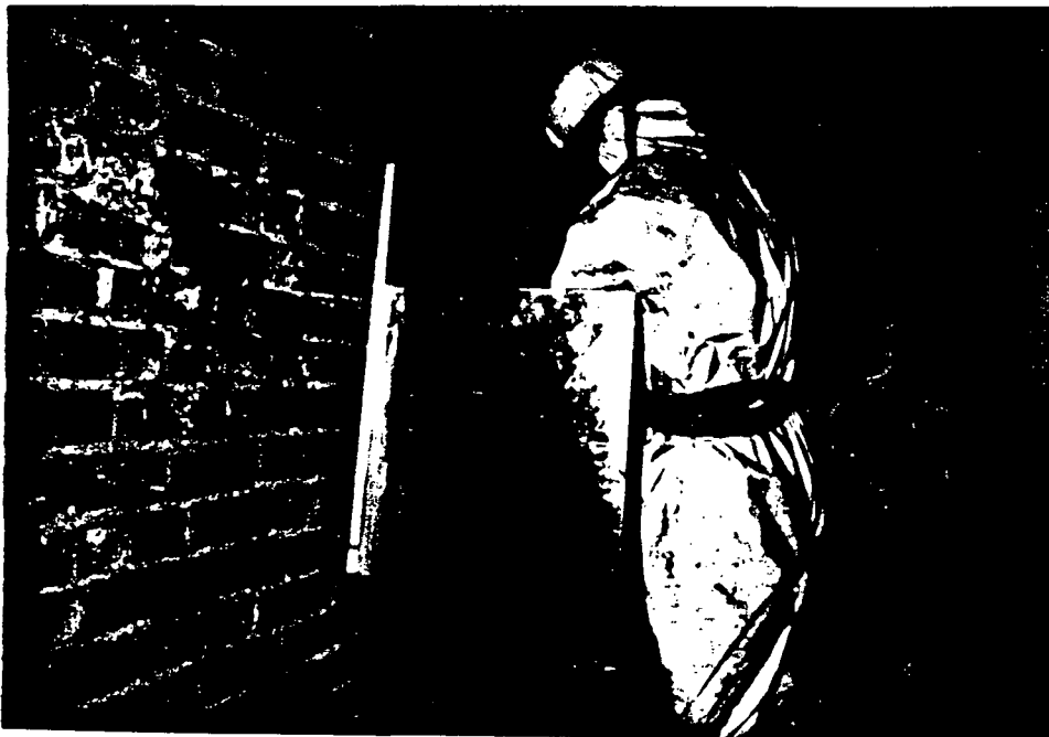
28. June 25, 1985 1420 Collection of brick wall sample NJP3-10-rm #1.
