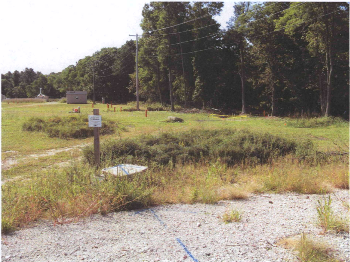
Photograph showing the proposed soil excavation area (near yellow tape to the right at the tree line) in relation to the existing extraction wells (shown in sheds in background). Groundwater monitoring wells in orange.
