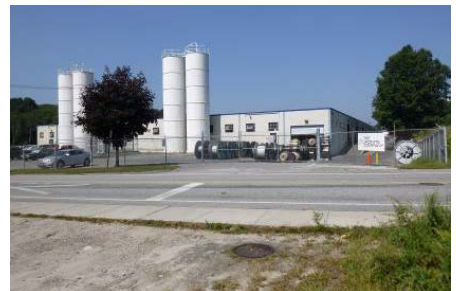
Figure 7: The former PAC facility (top) and Okonite Company, Inc. (bottom).
