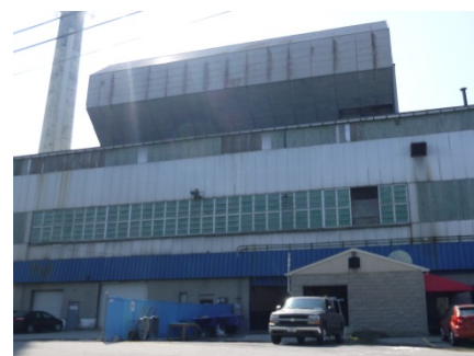
Figure 9: Rear view of the 23 Ashton Park Way facility.
