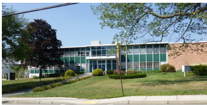
Figure 10: The former Peterson Puritan facility location is now home to Dean Warehouse Services and the Rhode Island Textile Company.
