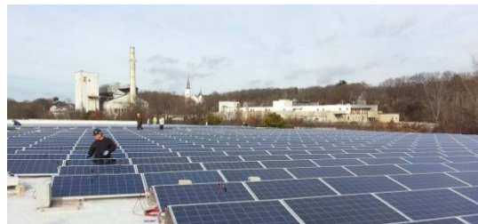
Figure 12: Rooftop MEGAWATT Energy Solutions solar panel installation.
