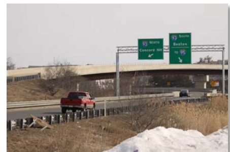
Figure 6. New I-93 interchange
