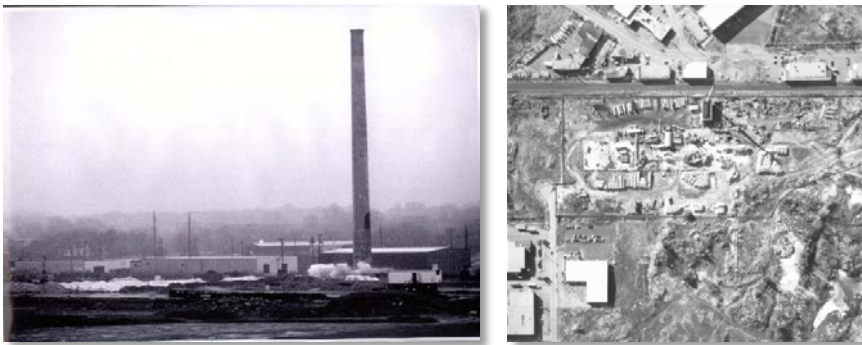
Figures 3 and 4. Site prior to cleanup and redevelopment
