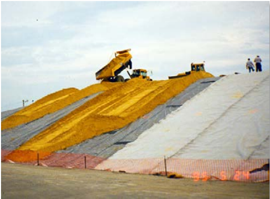
Figure 5. Cleanup underway on site
