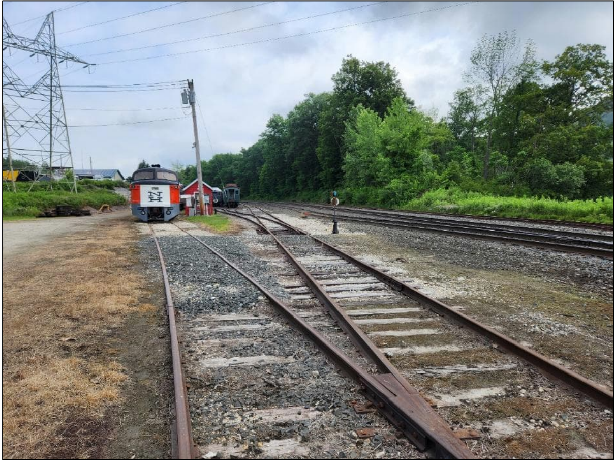
Photograph 4.16: STG-013 overview of northern APE, featuring active tracks and ballast. Facing north.
