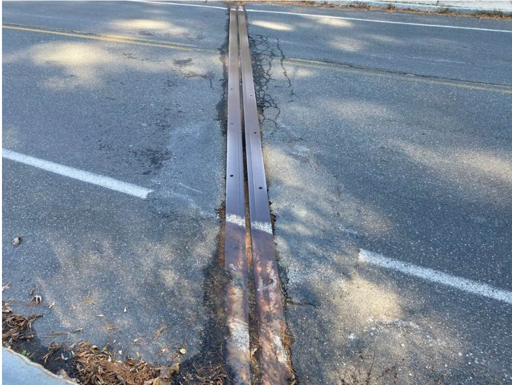
Photo 3: East deck joint filled with sand and debris. Note the approach pavement pulling away from the armor and patches.
