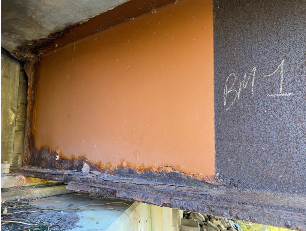
Photo 7: Rusting with delamination at the east end of beam 1. Also, note the delamination in the cover plate and the associated welds.
