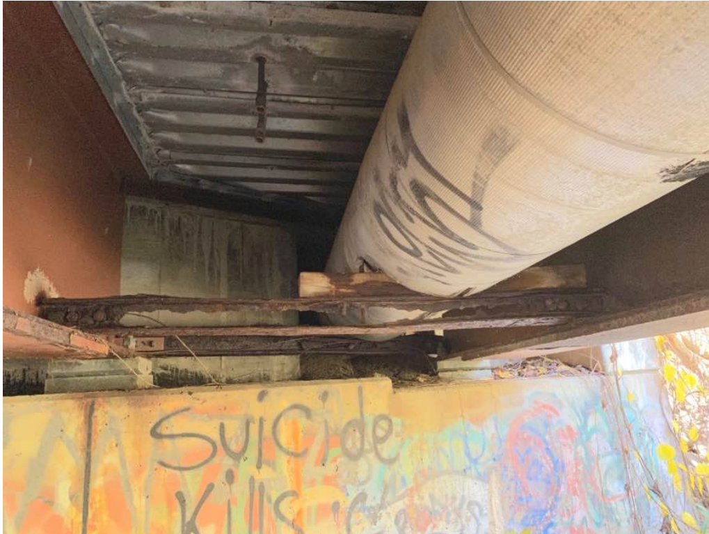
Photo 5: Rusted utility support at the west end of bay 1. Also, note the fill spilling through the utility bay in the backwall.
