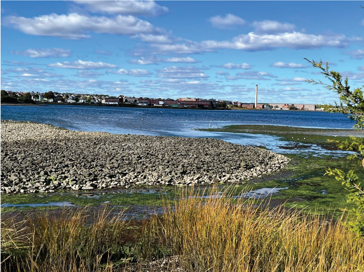
Figure 21: Cogg-East Cap looking northwest showing the eastern portion of the cap.
