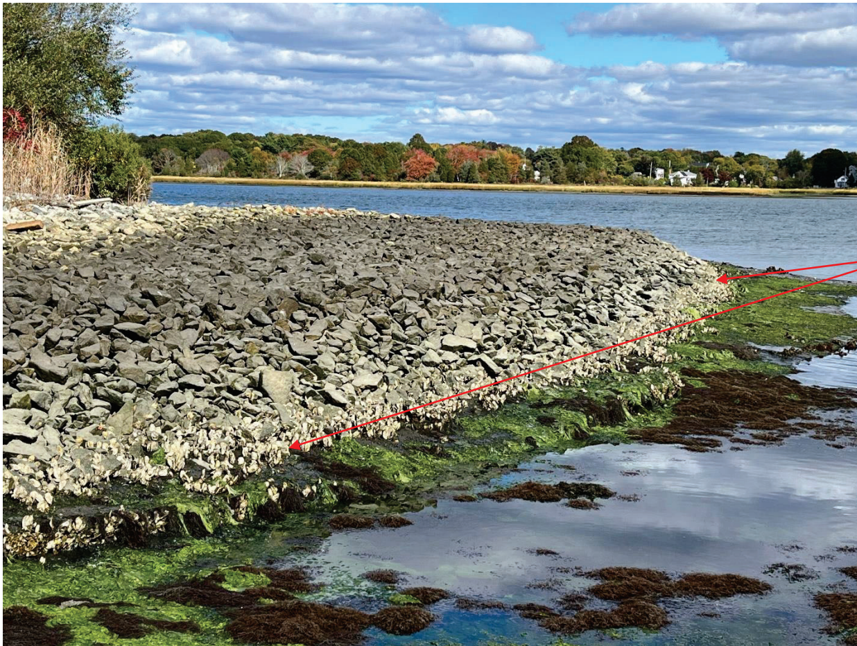
Figure 13: Pilot CDF Shoreline Cap looking east showing the southern part of the cap. Note the many oysters that have self-colonized along the toe-of-slope.
