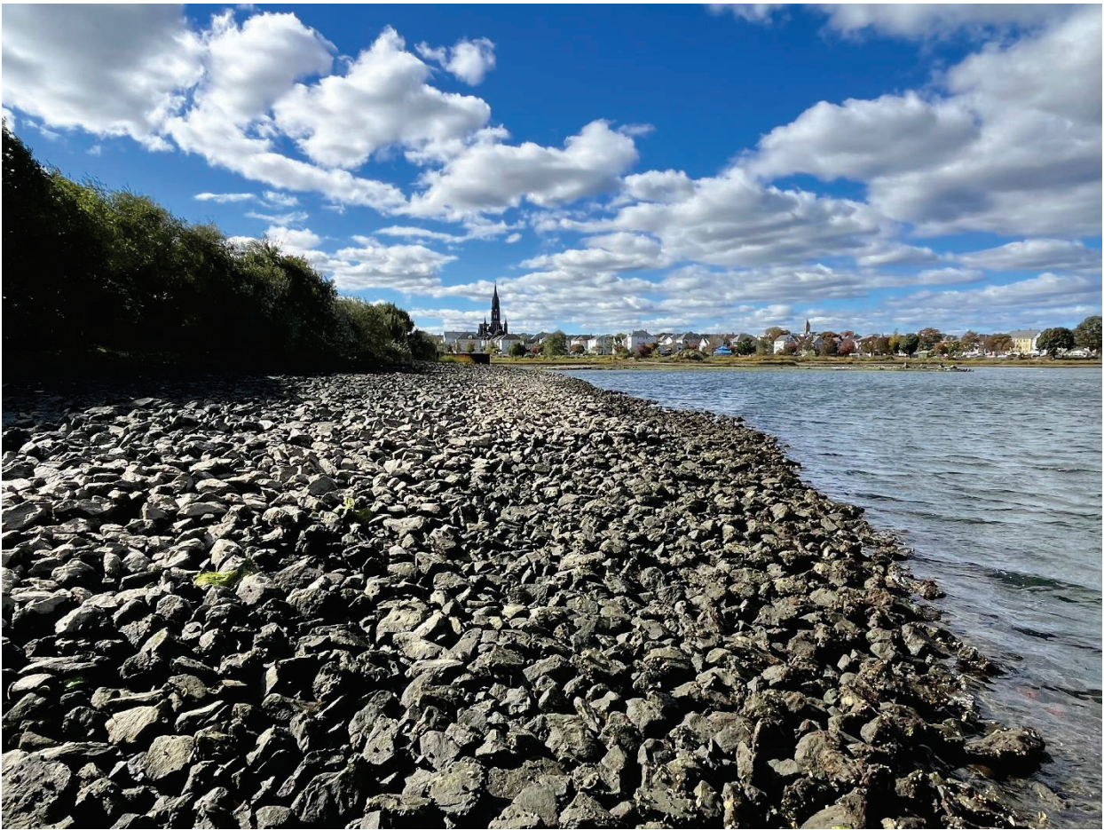
Figure 15: Pilot CDF Shoreline Cap looking west showing the northern portion of the cap.
