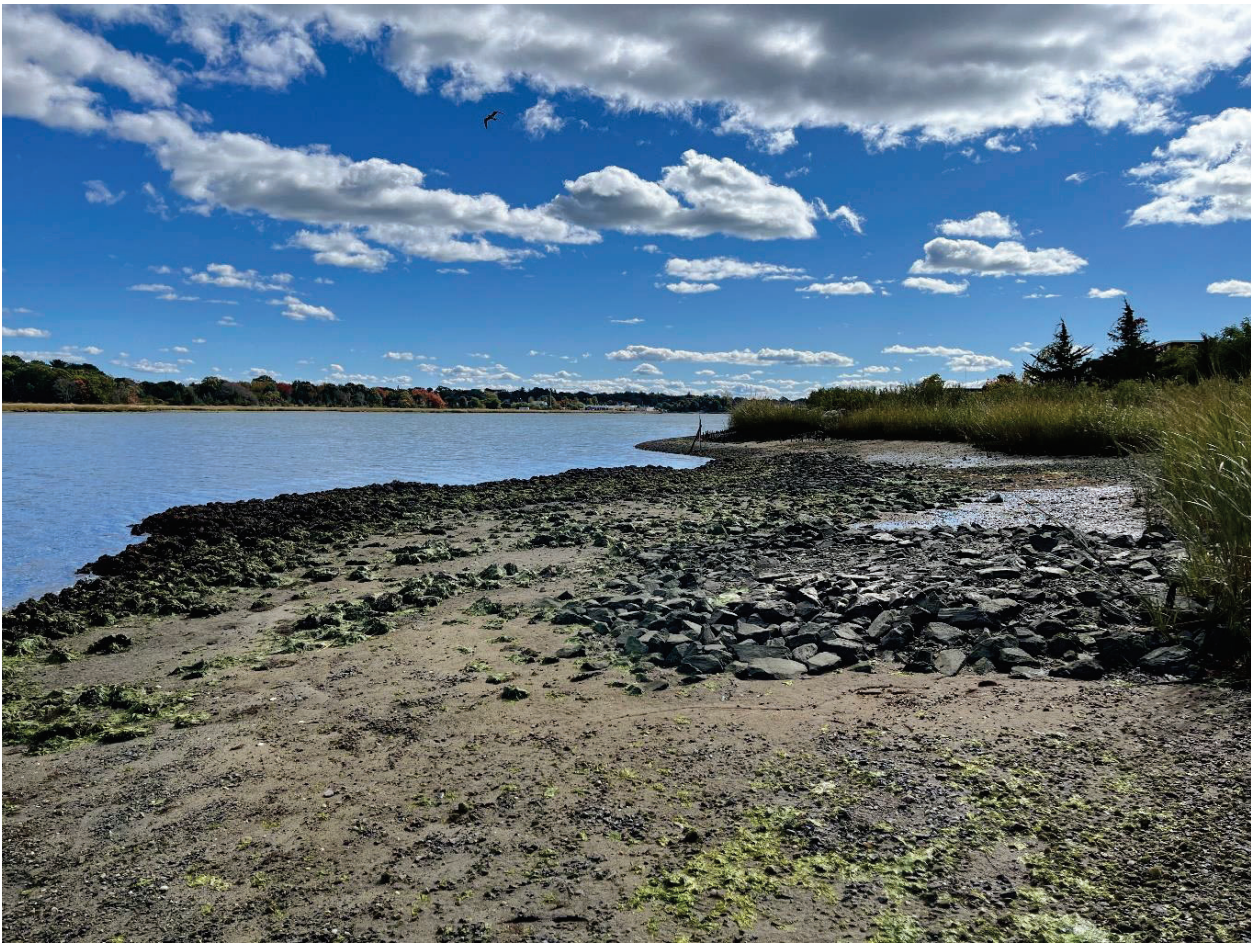
Figure 11: L-014 Cap: Looking south. The sandy topsoil in the foreground is topsoil that eroded from the abutting WZ-4 saltmarsh restoration, and NOT the underlying sediment cap isolation layer.
