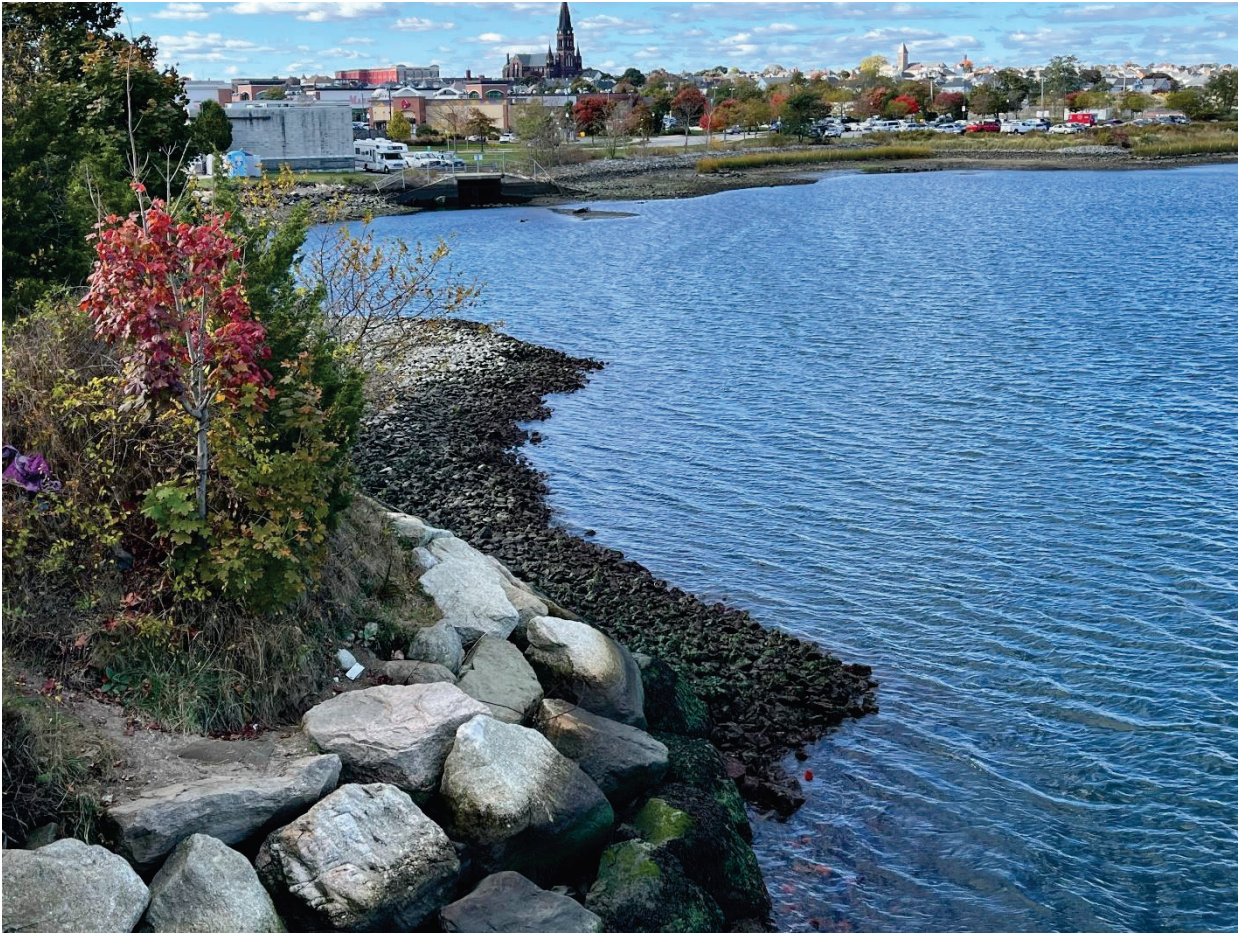
Figure 18: Cogg-West Cap looking west from the opening of the Coggeshall Street bridge.
