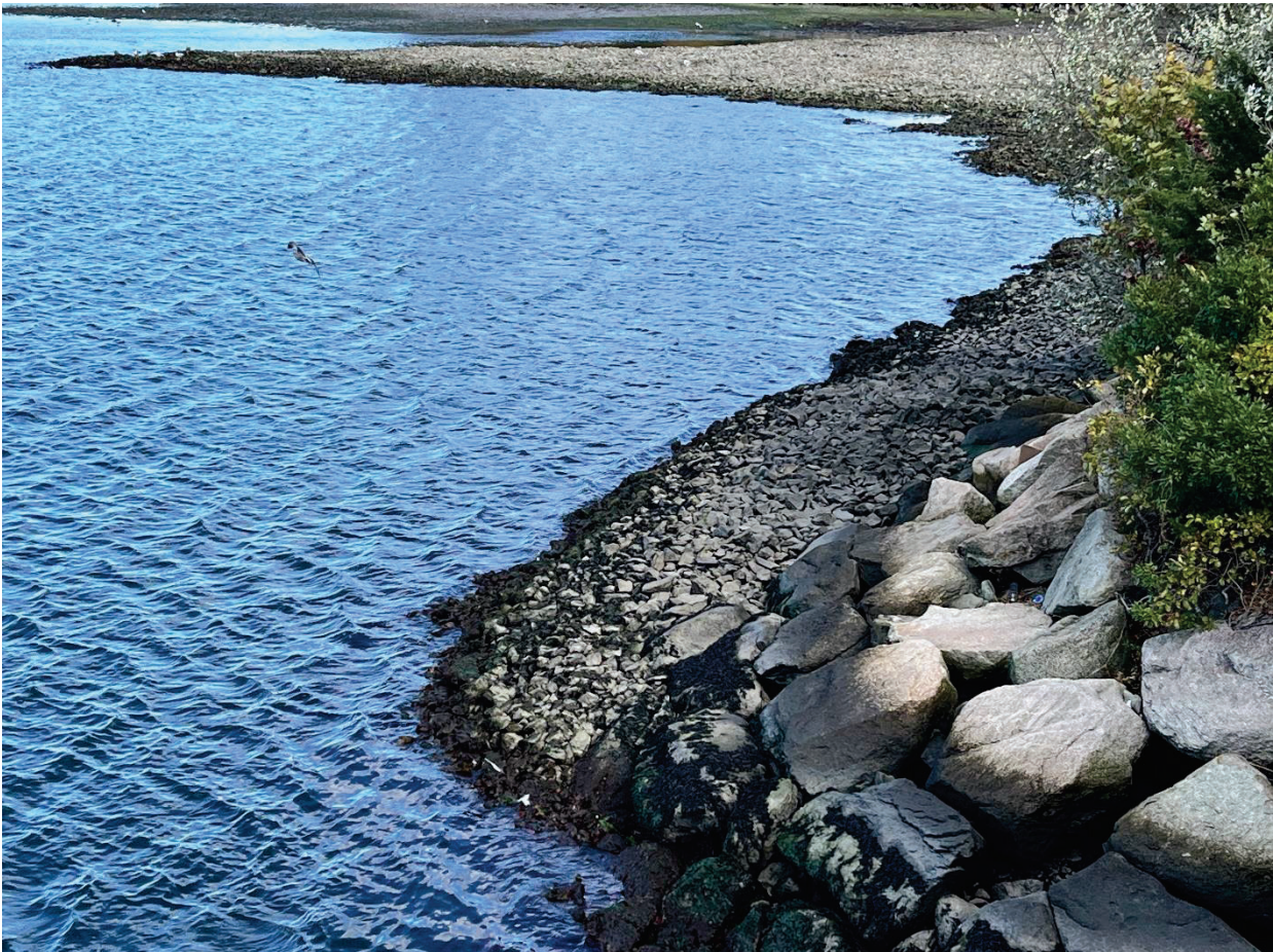
Figure 19: Cogg-East Cap looking east from the opening of the Coggeshall Street bridge.
