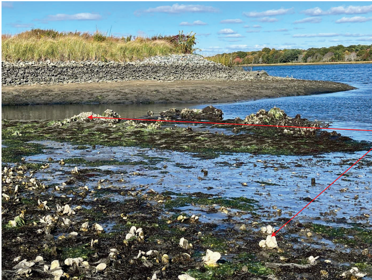
Figure 16: Parcel 265 Cap looking north. Note that due to the extreme low tide this is by far the most of this cap that has been visible during these shoreline visual inspections.
