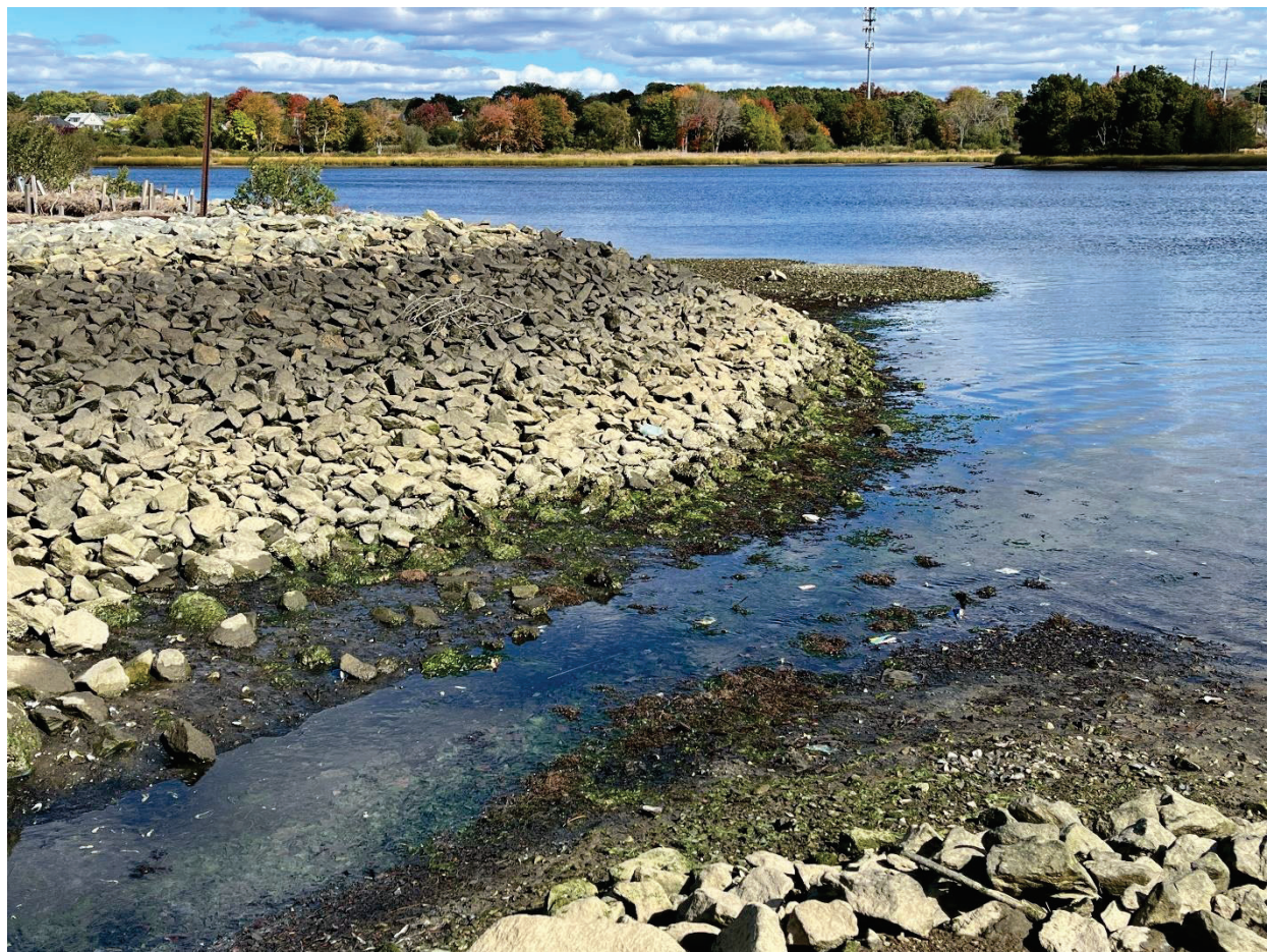
Figure 5: Aerovox Cap: Looking northeast showing the southern area of the cap and the abutting Hadley Street storm drain swale in the foreground.
