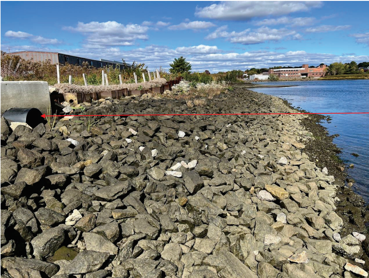
Figure 3: Aerovox Cap: Looking north showing the South Trench storm drain outlet.
