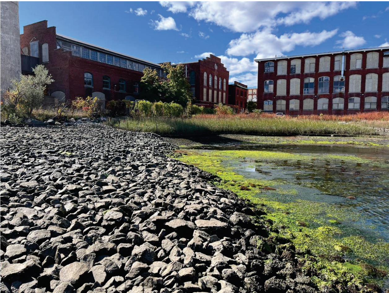
Figure 9: Crib Cap: Looking west showing the northern east-west trending edge of the cap. The restored WZ2/3 saltmarsh plantings are in the background beyond the cap armor stone.
