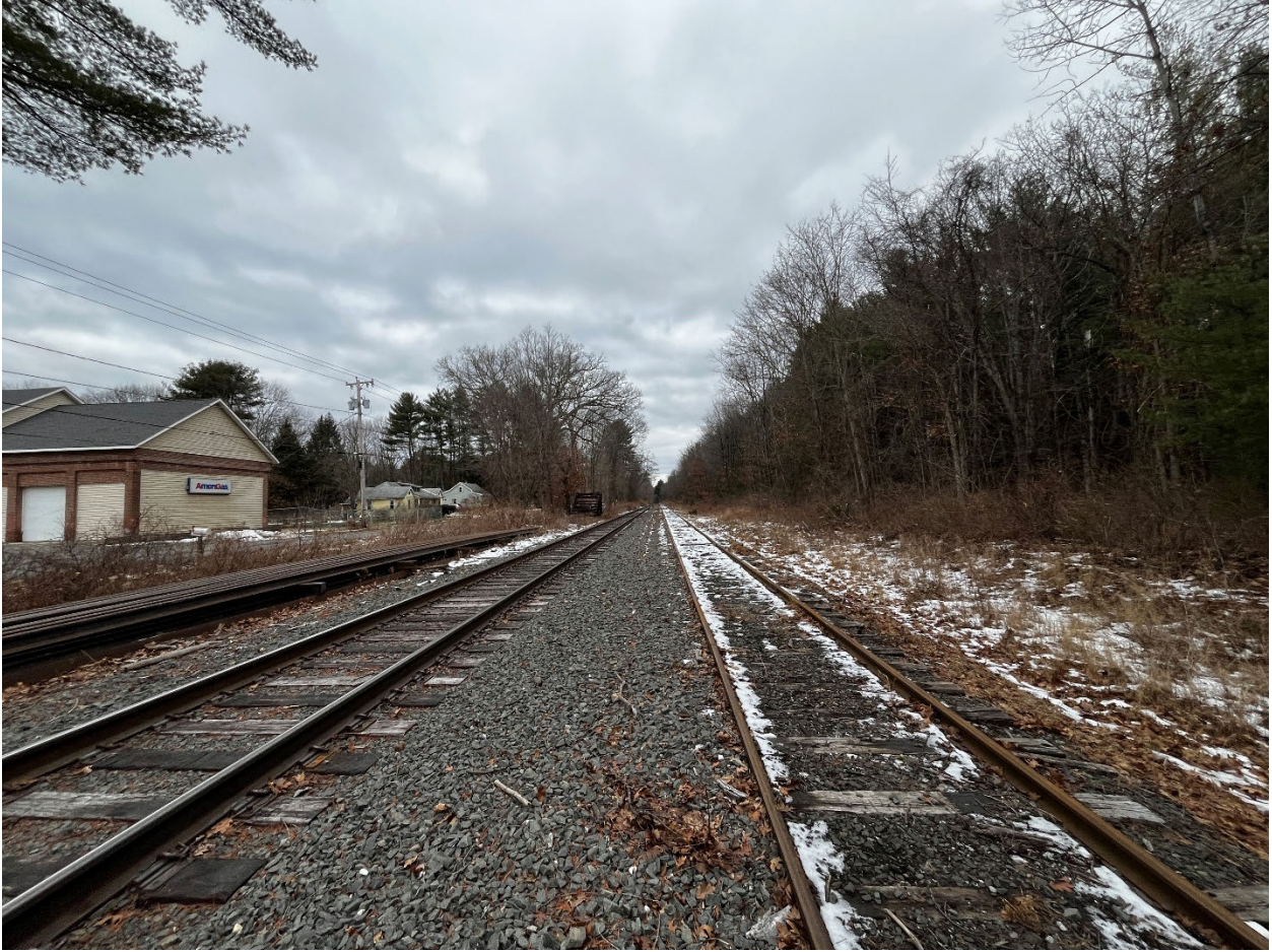
Approximately 0.85 miles of railroad siding along Van Deusenville Road, Great Barrington, near Reach 8.
