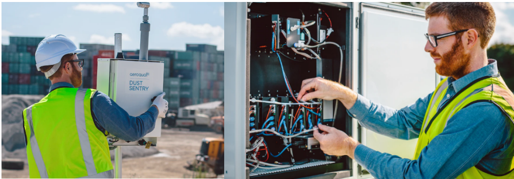
Figure 2 Deployable particulate air monitoring station, photos courtesy of Aeroqual, Inc.
