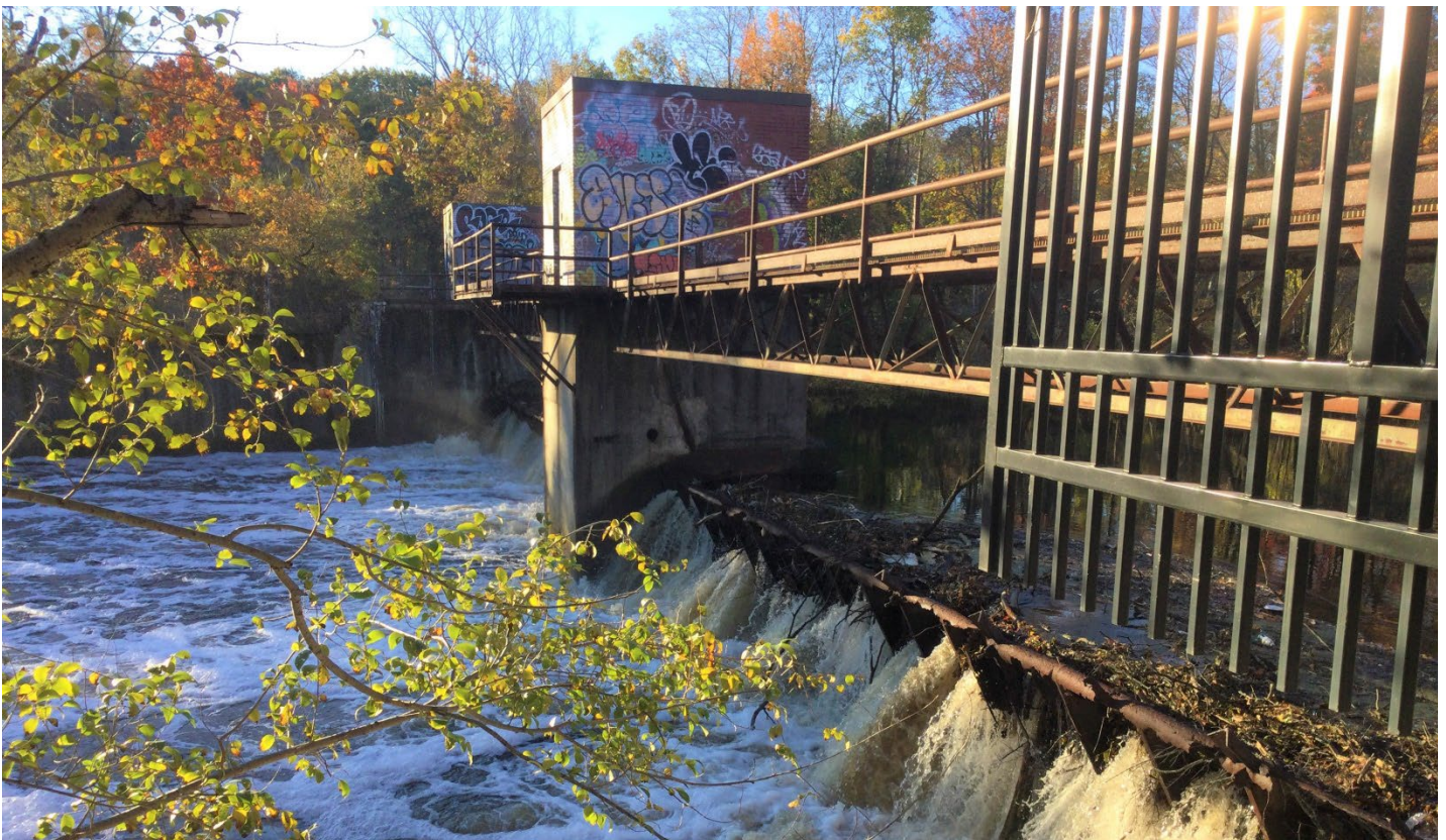
The Tileston and Hollingsworth dam on the Lower Neponset River.
