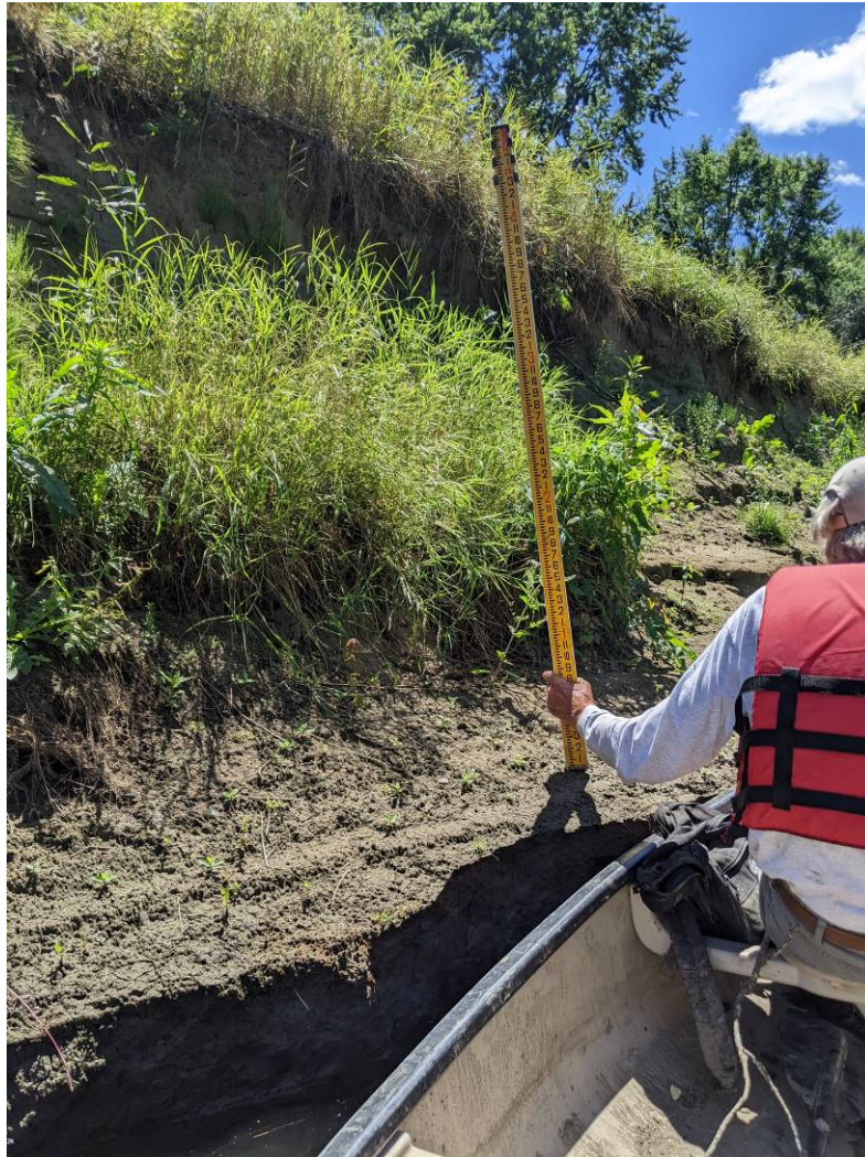
BEHI – VERY HIGH RATING EXAMPLE Station 233+25 Left Bank (Bank No – L130)
