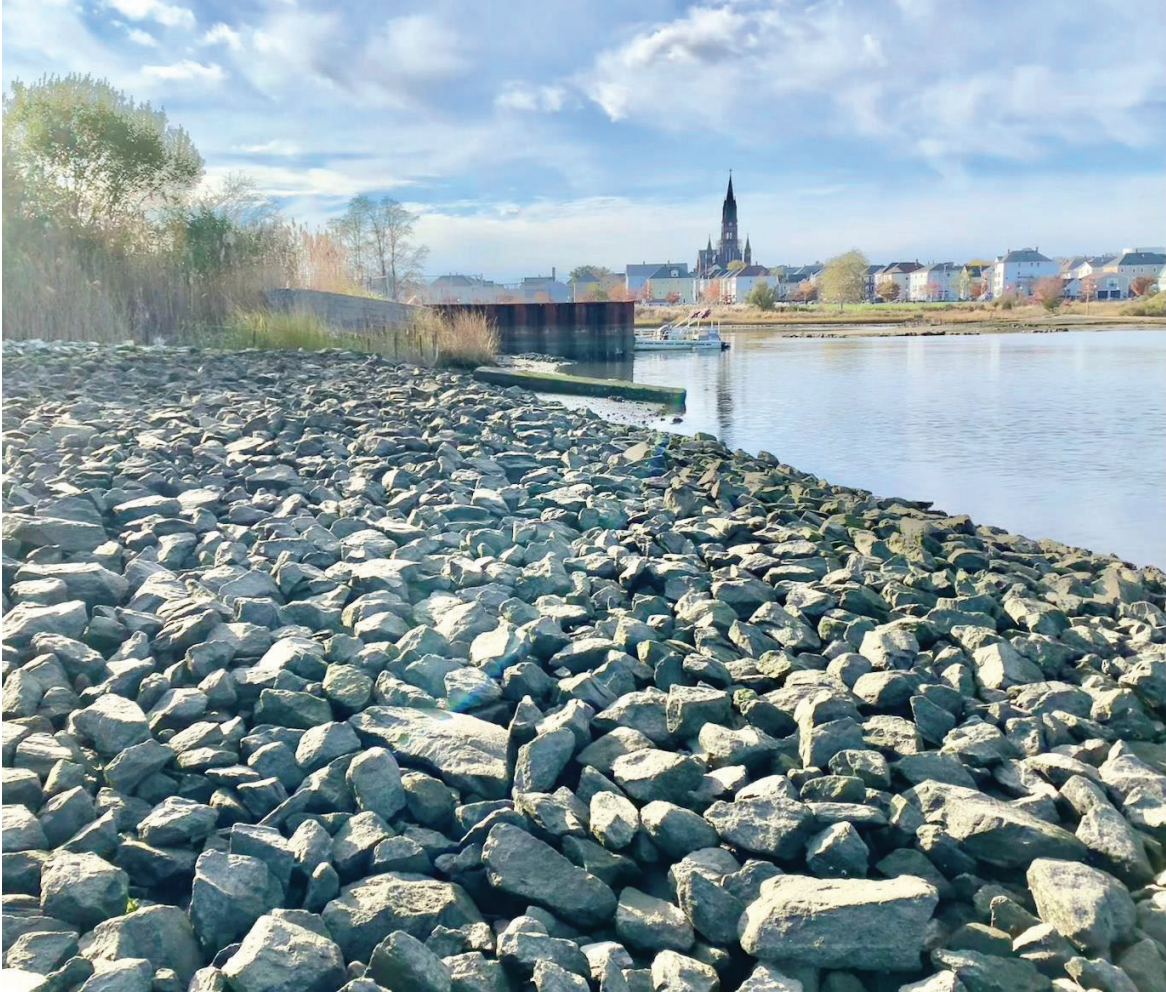
Figure 20: Pilot CDF Shore- line Cap: looking west showing the northern edge of the cap.
