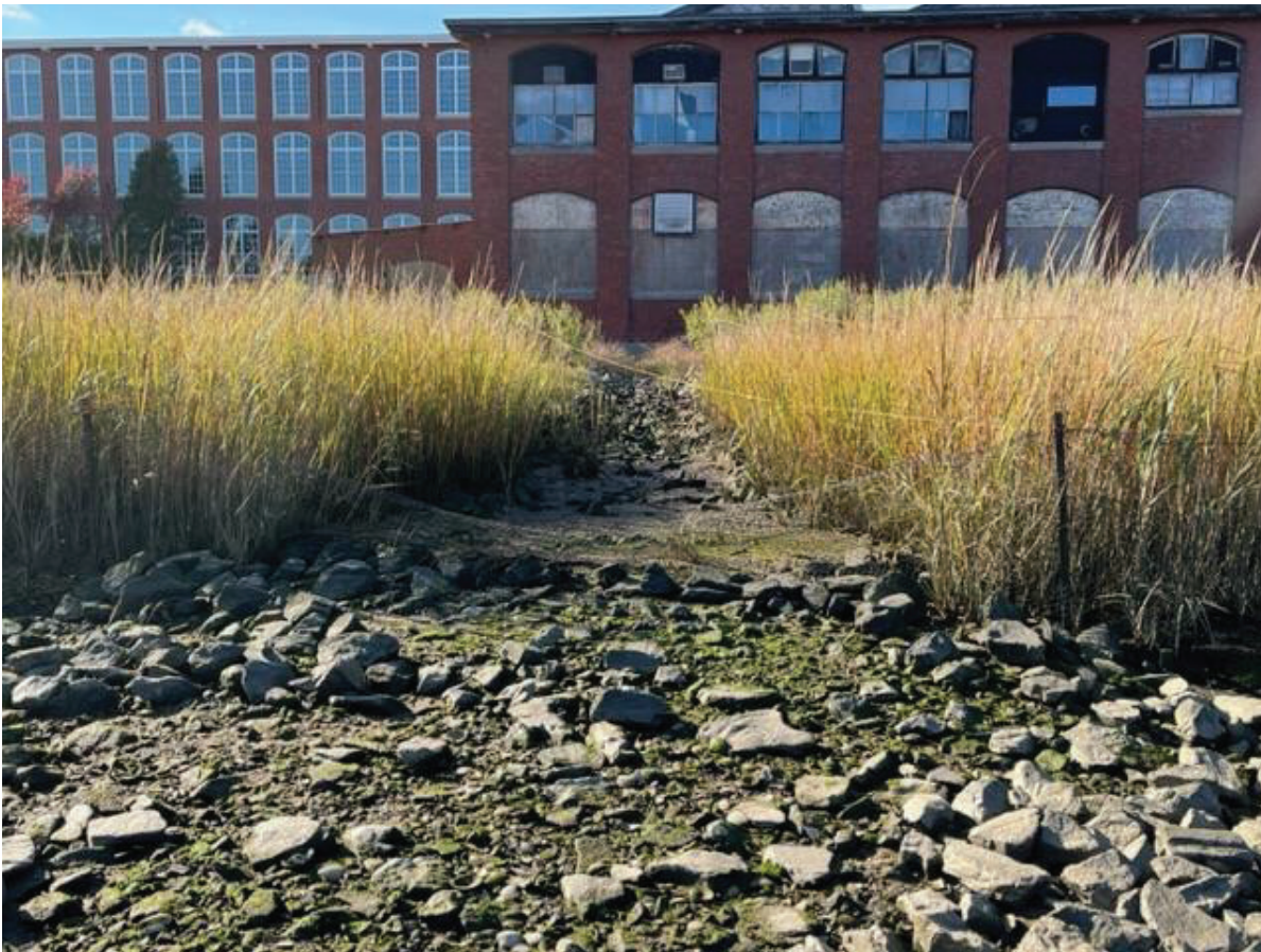
Figure 15: L-014 Cap: Looking west showing the drainage swale where original WZ4 topsoil was likely discharged onto the cap.
