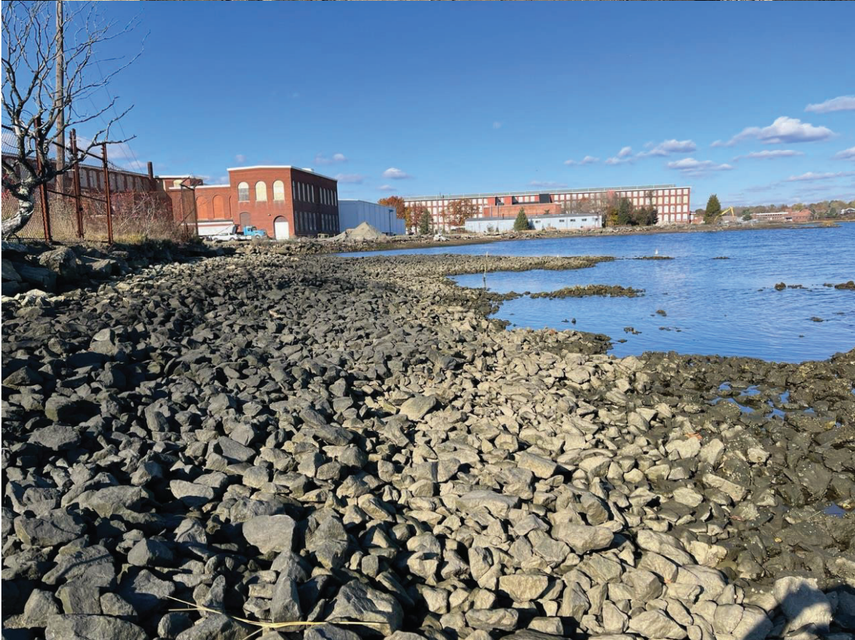
Figure 8: Crib Cap: Looking north.
