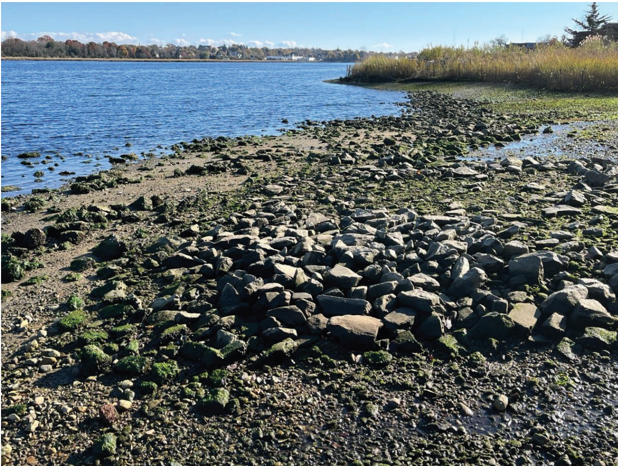
Figure 14: L-014 Cap: Looking south showing area where original topsoil from the abutting WZ4 restoration washed into the armor stone (WZ4 topsoil was subsequently replaced).
