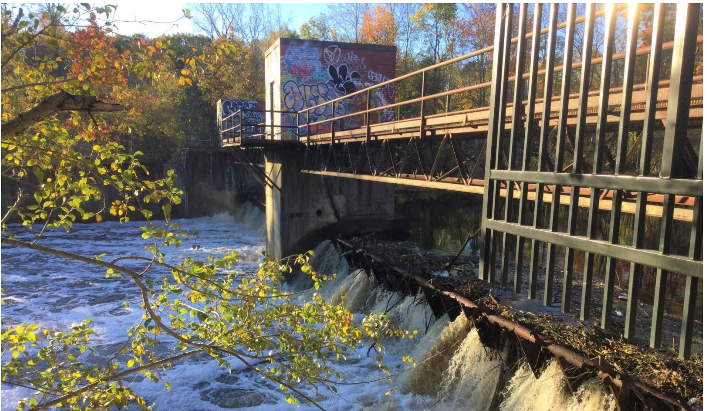
La represa Tileston and Hollingsworth en el Lower Neponset River.
