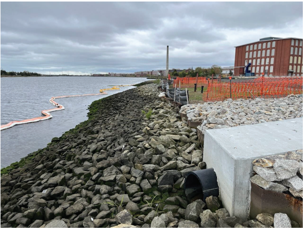
Figure 4: Aerovox Cap: Looking south showing the new South Trench discharge structure in foreground. Emergent salt grass noted in previous inspection remains near outfall.
