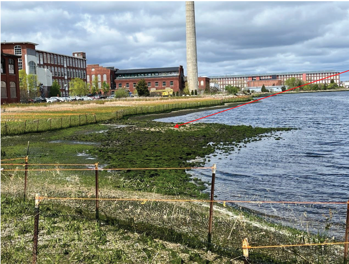
Figure 9: L-014 Cap looking north. Light brown color is silt/topsoil deposition from a WZ-4 drainage swale.
