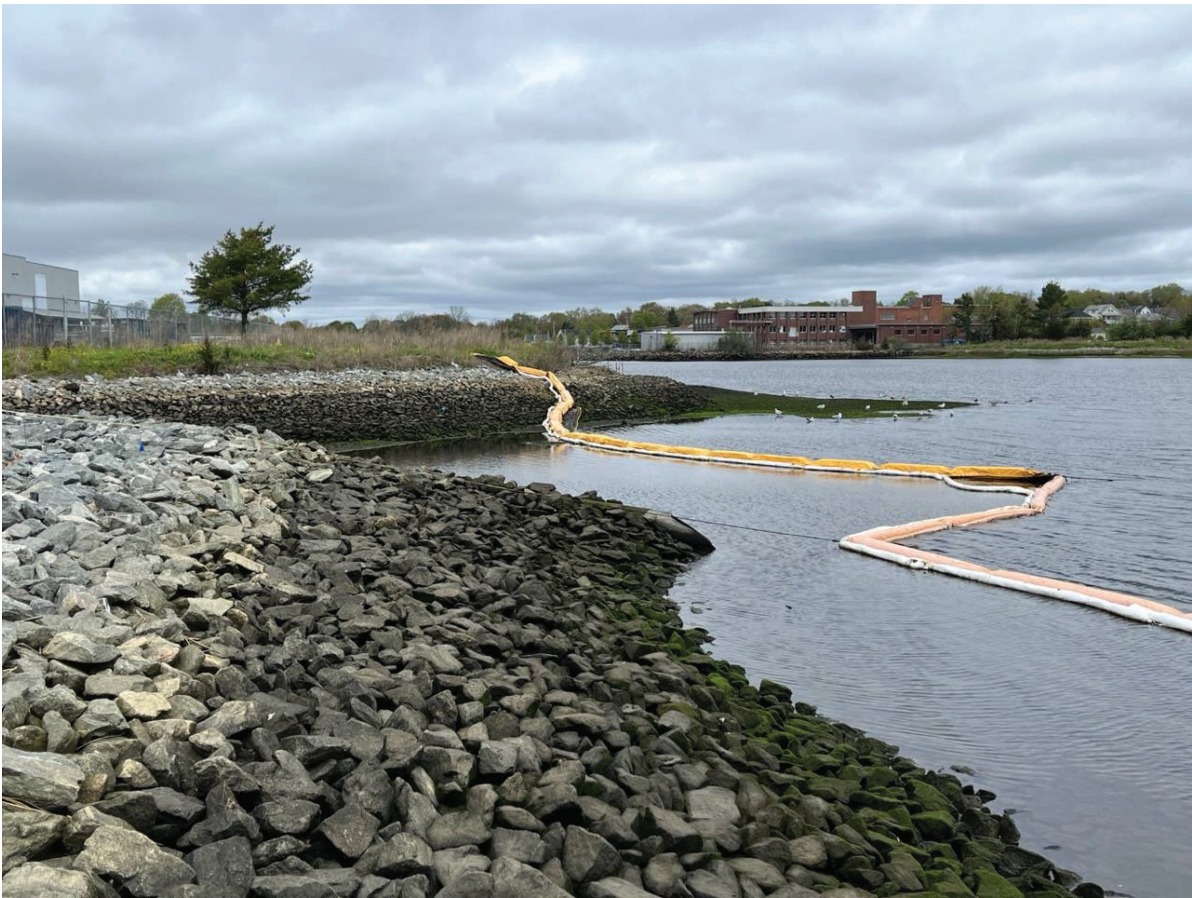
Figure 3: Aerovox Cap: Looking north showing the northern portions of the cap. The silt curtain and oil boom are from on- going 21E operations.
