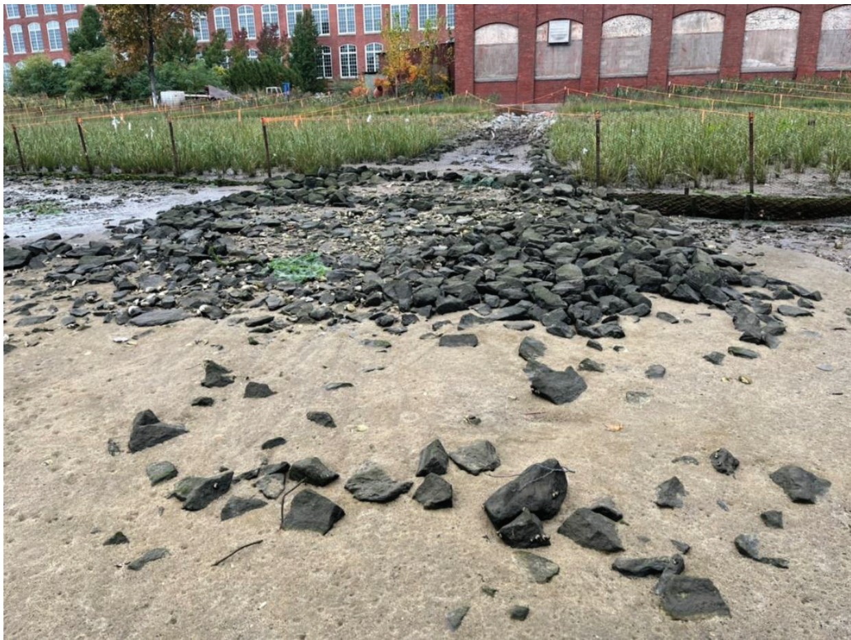
Figure 12: L-014 cap looking west, showing drainage swale and topsoil washed onto cap surface. Restored WZ4 saltmarsh in background.
