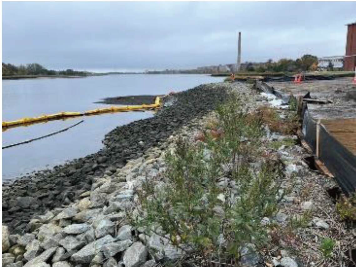
Figure 4: Aerovox cap looking south. Note native high tide bush ( Iva frutescens ) emerging at top of slope. Underlying this part of the armor stone is the original, large-stone-size seawall, thus non-woody vegetation such as this is fine (and may help stabilize the surface).
