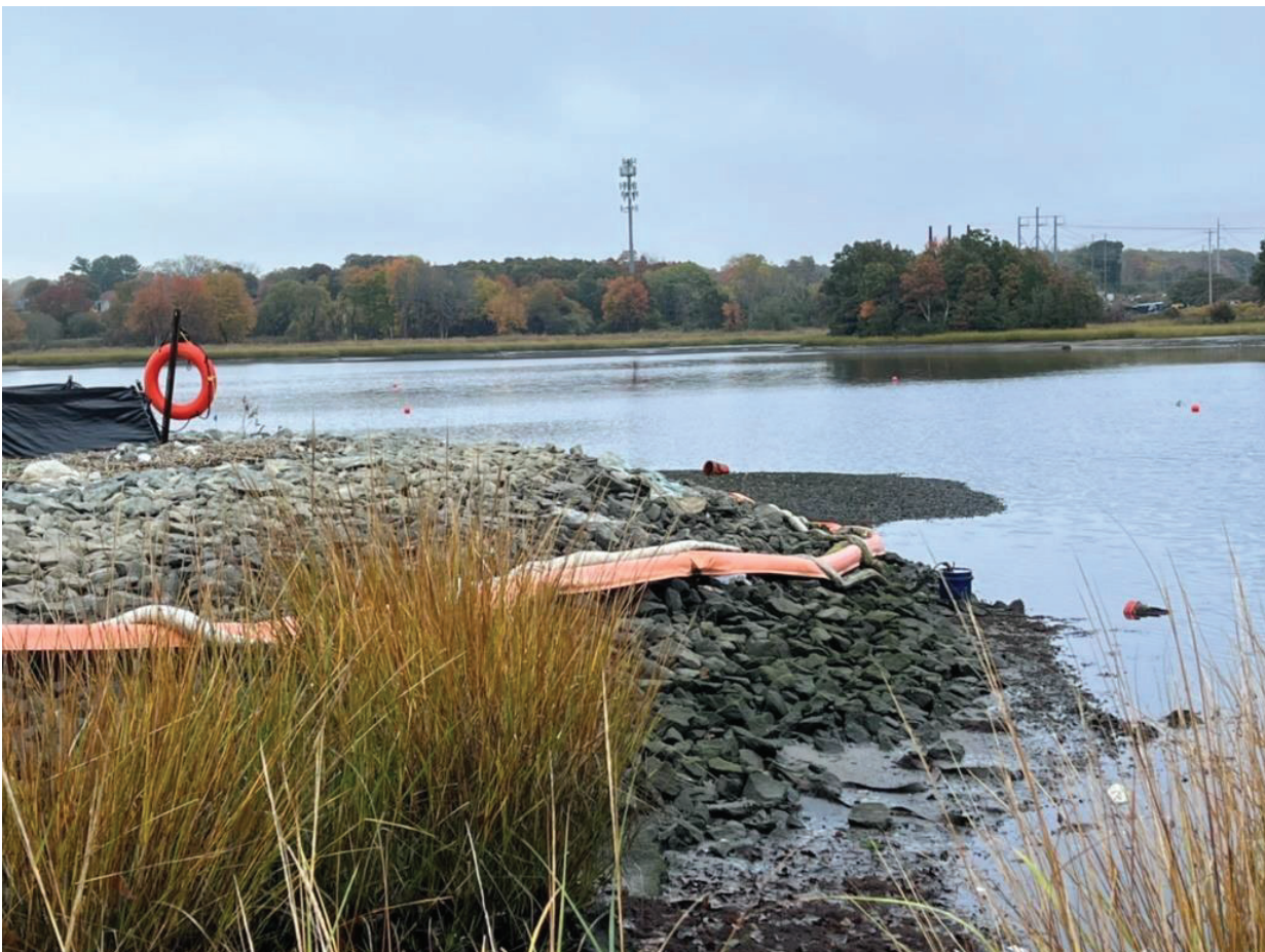
Figure 6: Aerovox cap looking east from the southern edge of the cap. Foreground is the east end of the large Hadley Street storm drain.
