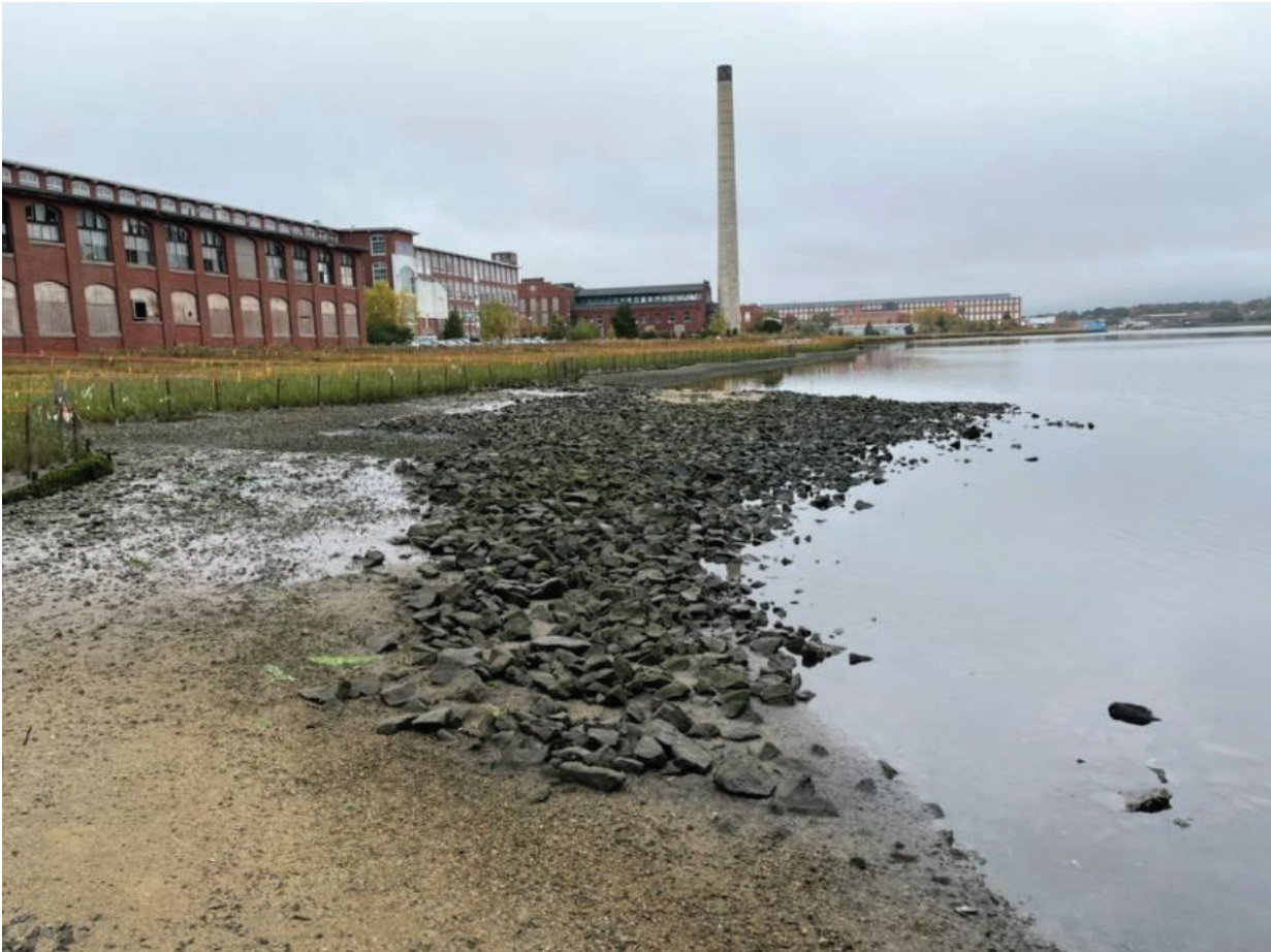
Figure 11: L-014 cap looking north, after “smoothing” operations during WZ4 Remedial Action (RA) in May 2022. Restored WZ4 saltmarsh is in the background.
