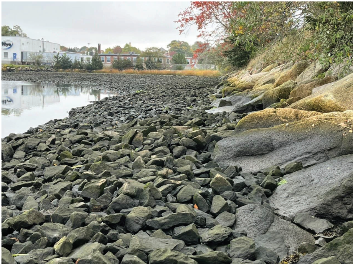
Figure 24: Cogg-East Cap looking east from near the bridge opening.
