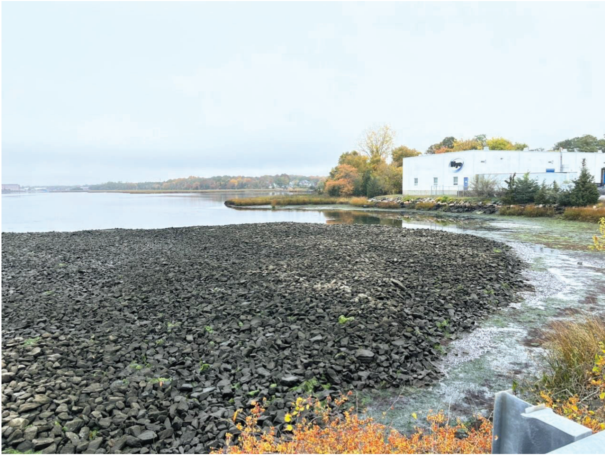
Figure 23: Cogg-East Cap looking north from the eastern edge of the cap.
