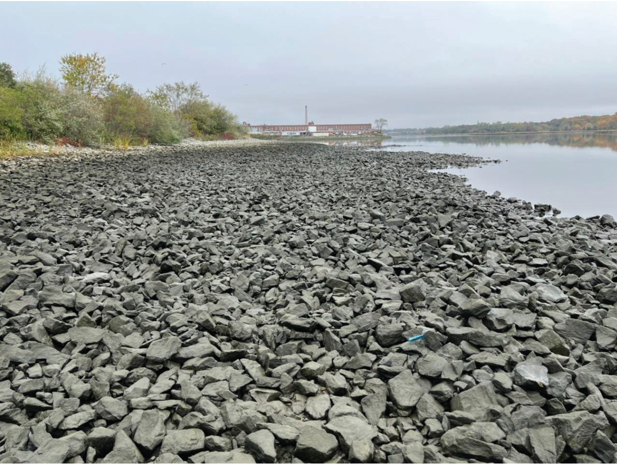
Figure 15: Pilot CDF Shoreline Cap looking north.
