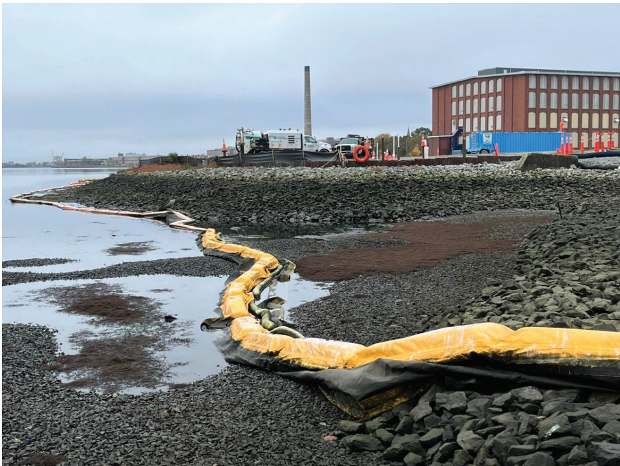
Figure 2: Aerovox cap looking south from the northern area of the cap. The oil boom is from the ongoing Aerovox 21E work. The brown color is a seaweed mat.
