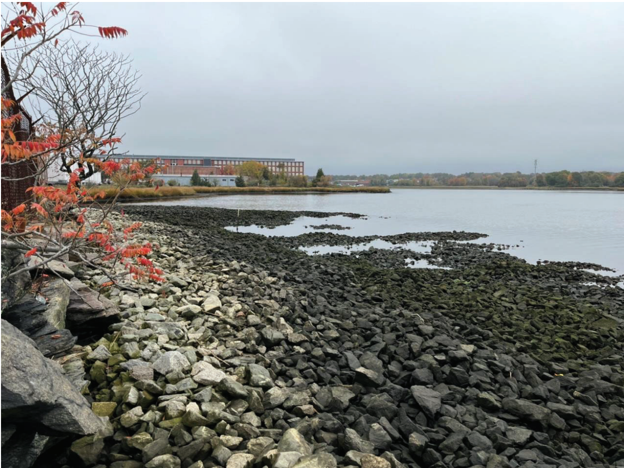
Figure 7: Crib cap looking north from the south end of the cap. White pole is the location of an outfall pipe (extended through cap during cap construction).
