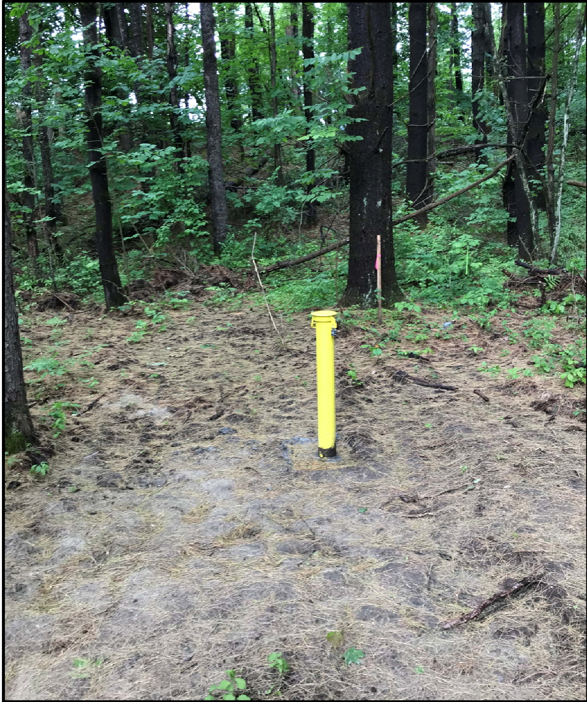
Figure 16. View West of Monitoring Well 2022-1 in in Area B with Gravel Mine Berm in the Background.
