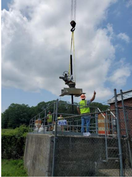
Photo 7: Removing gate actuator.
