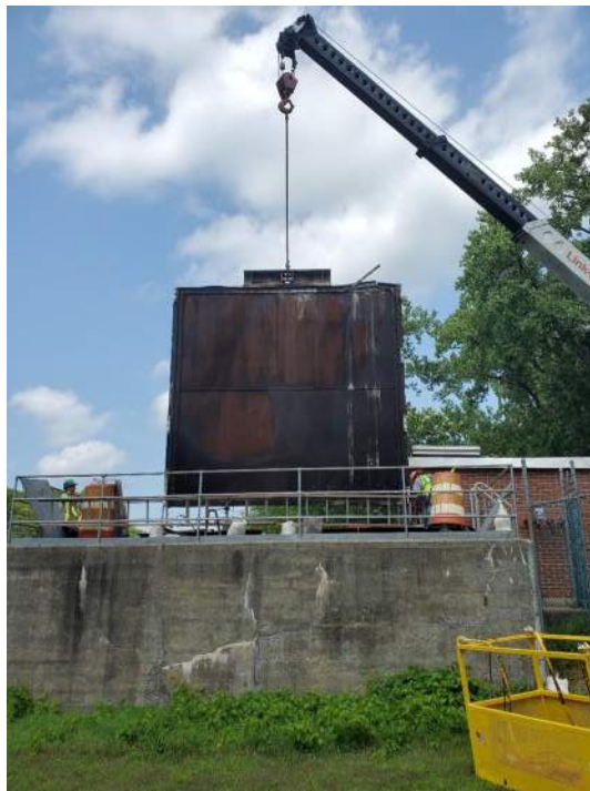
Photo 8: Removing slide gate.
