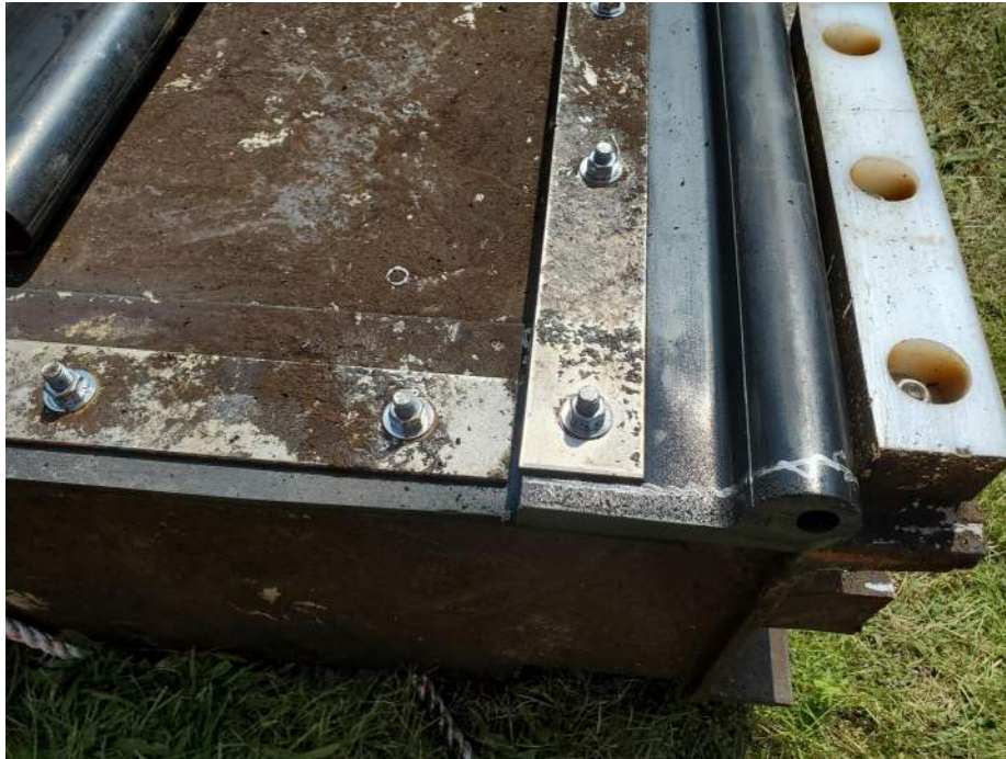
Photo 13: Side seal of gate after replacement.
