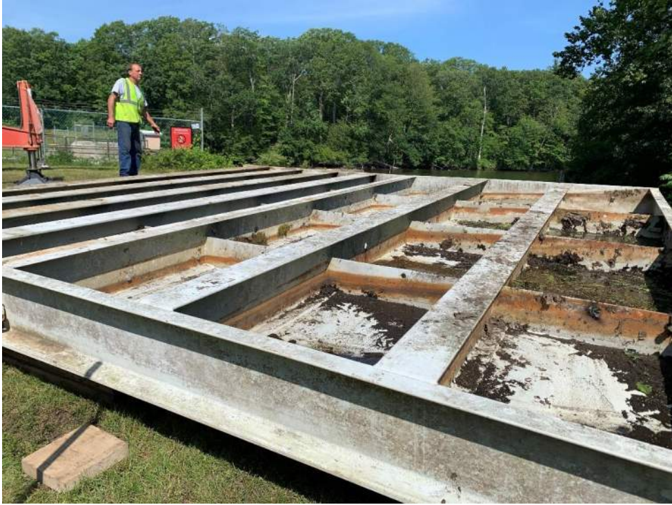
Photo 1: Temporary bulkhead section prior to insertion.
