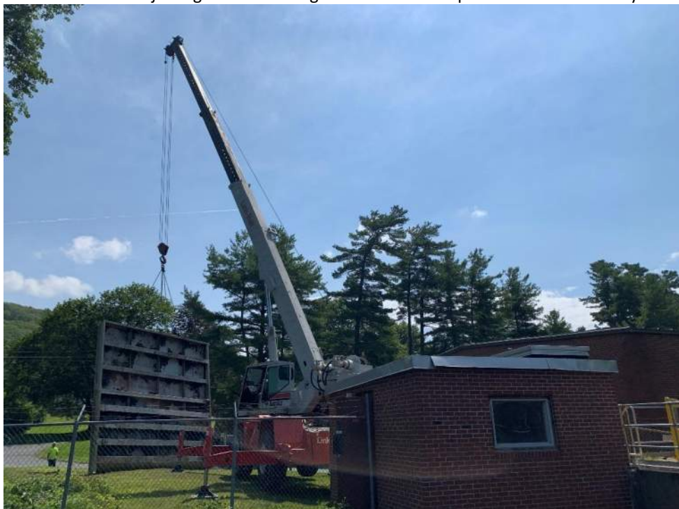
Photo 4: Lifting temporary bulkhead (after panels connected).
