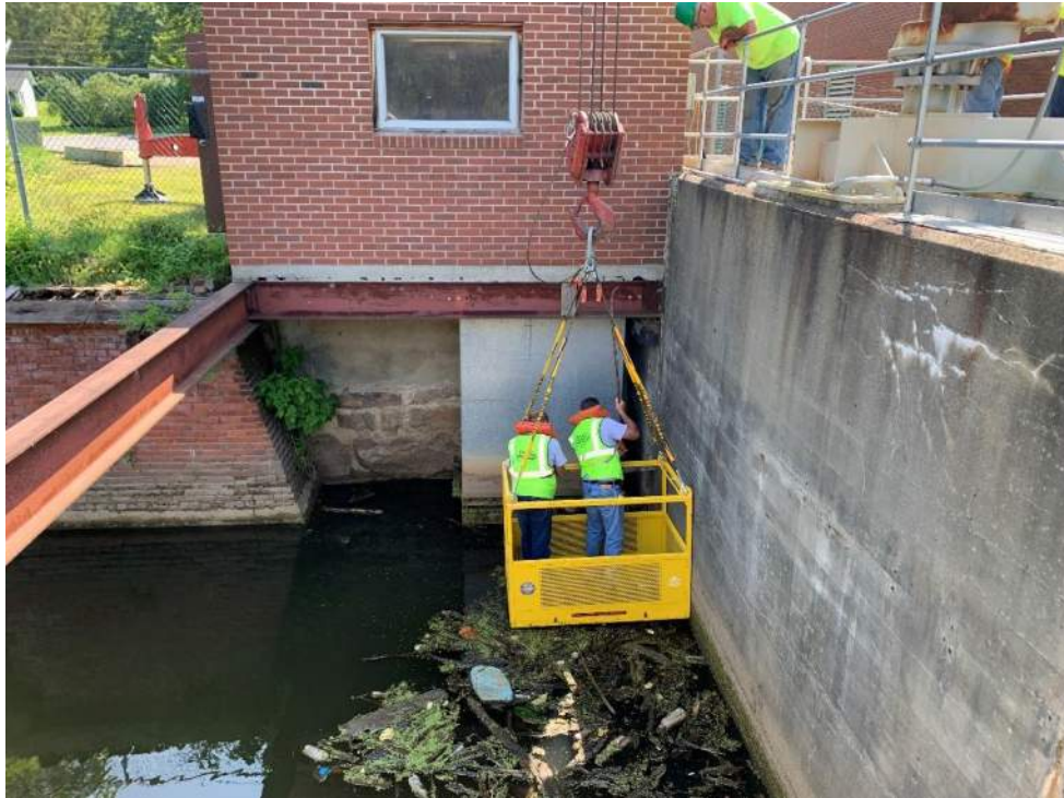
Photo 3: LB adjusting the bulkhead guide brackets on upstream face of forebay.
