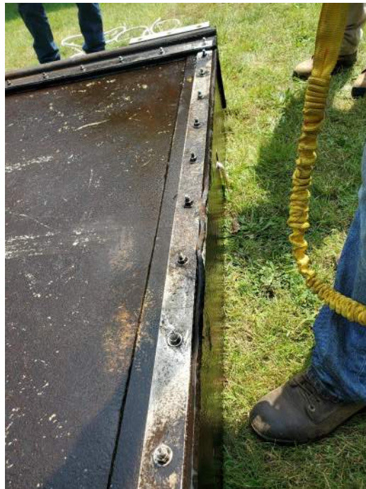
Photo 10: Side seal of gate prior to replacement.
