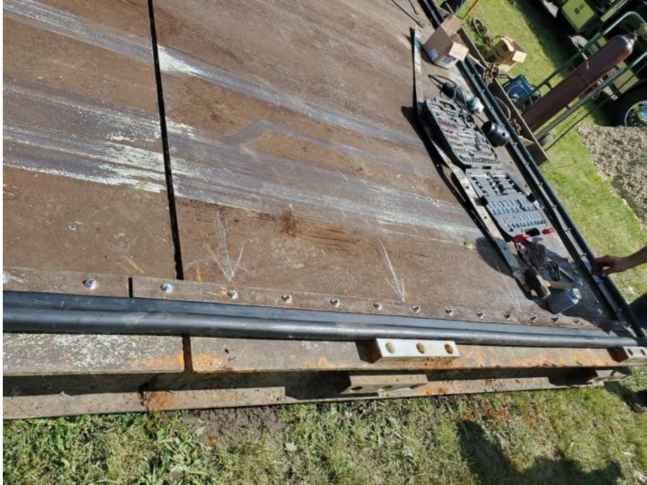
Photo 11: Seal replacement in progress.
