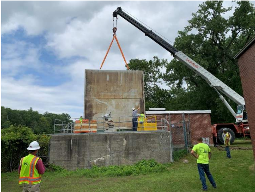
Photo 5: Setting temporary bulkhead in place.
