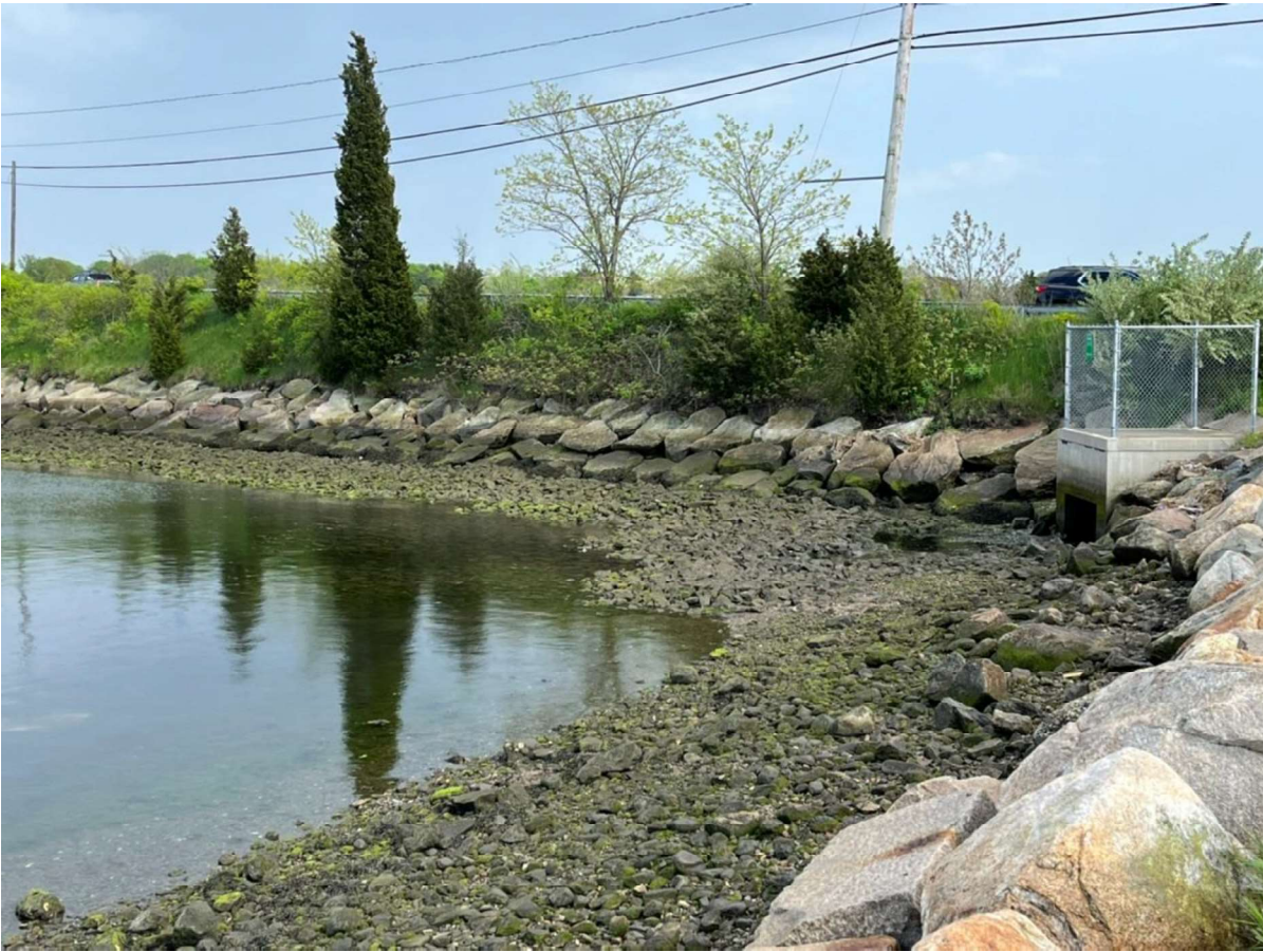
Figure 17: Cogg-West cap looking south showing the city storm drain.
