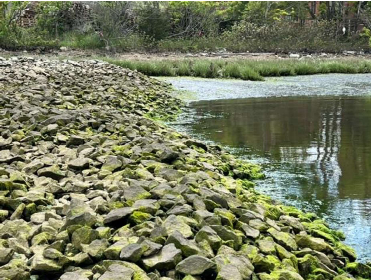
Figure 8: Crib cap looking west showing the northern E/W-trending edge of the cap.
