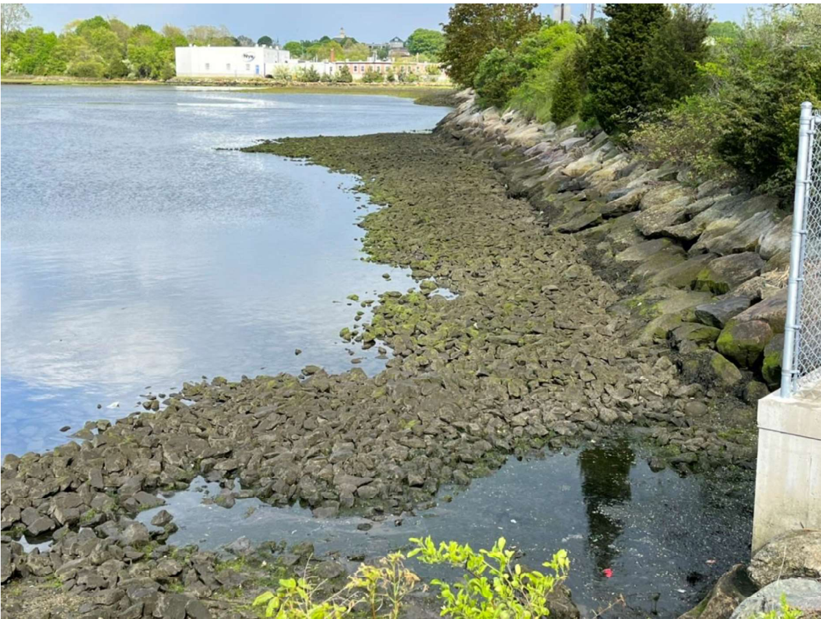
Figure 18: Cogg-West cap looking east showing the Coggeshall Street bridge embankment.
