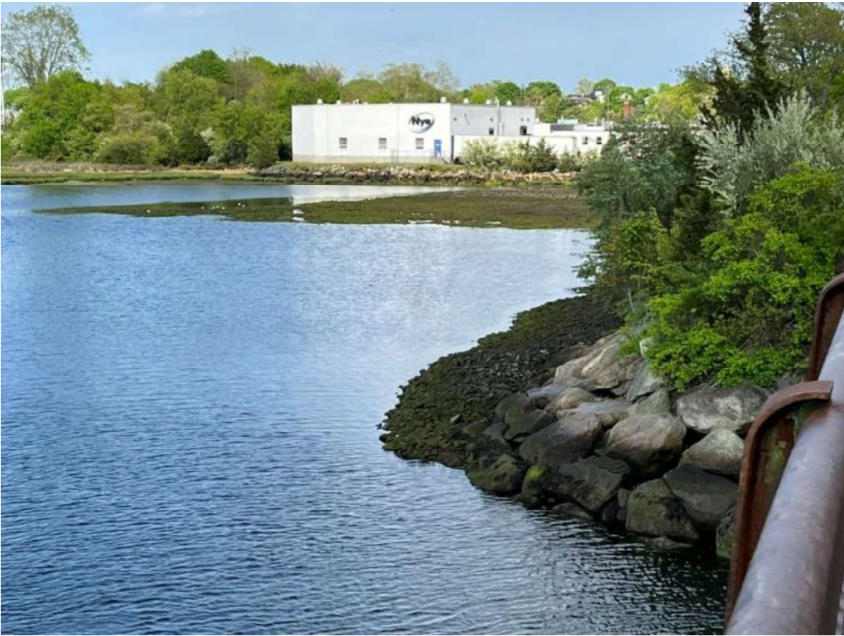
Figure 19: Cogg-West cap looking east showing the Coggeshall Street bridge opening.
