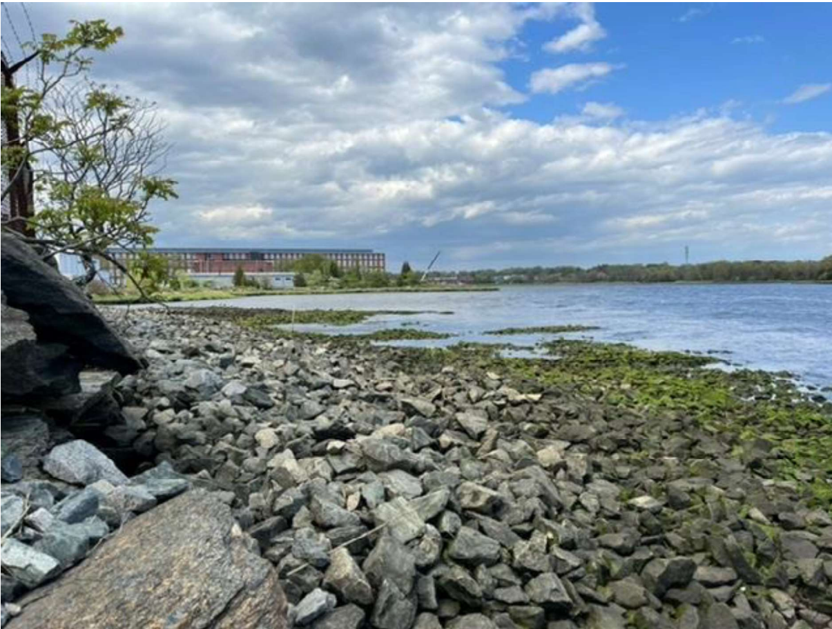
Figure 5: Crib cap looking north from the southern area of the cap.
