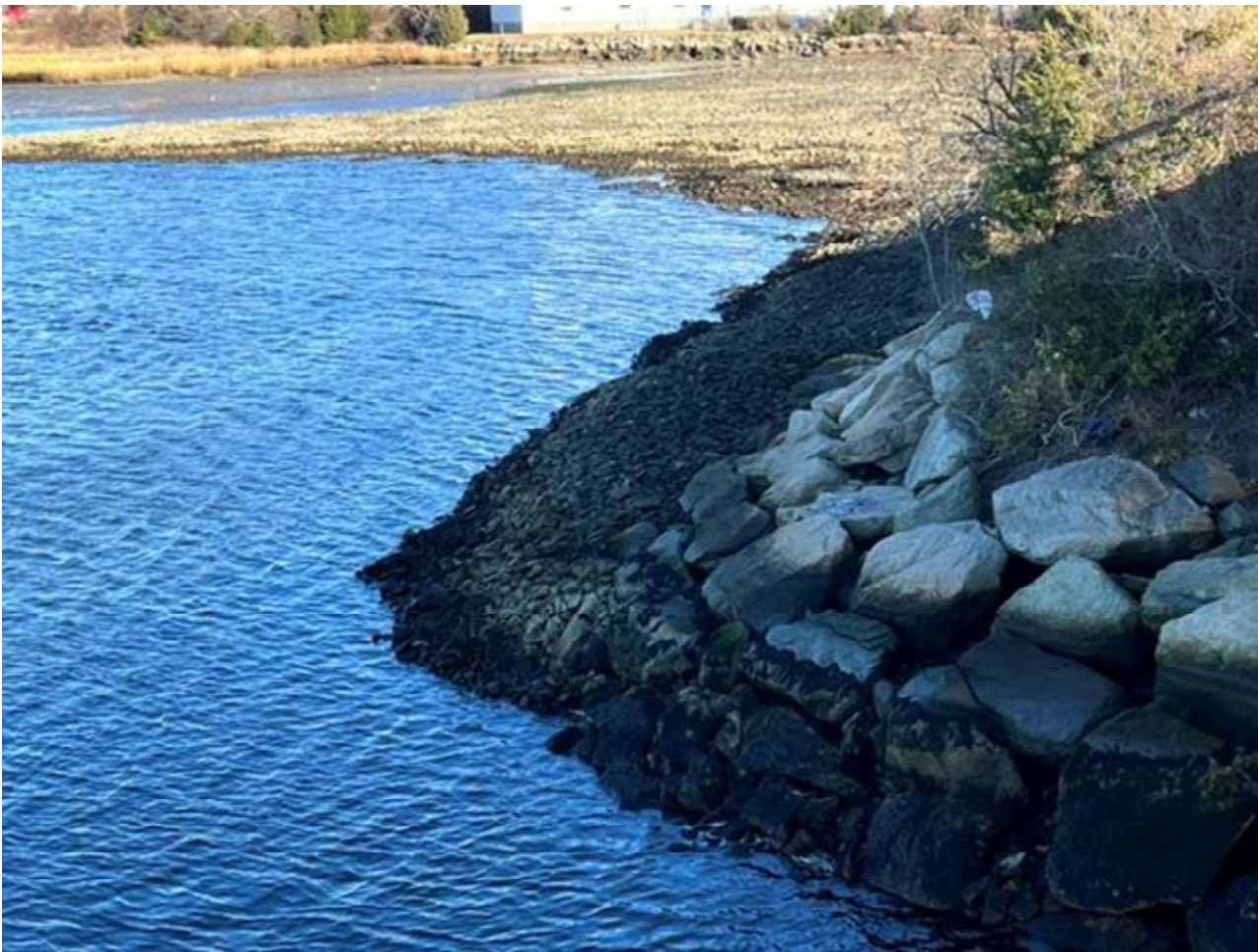
Figure 25: Cogg-East cap looking east. Bridge opening in fore-ground.
