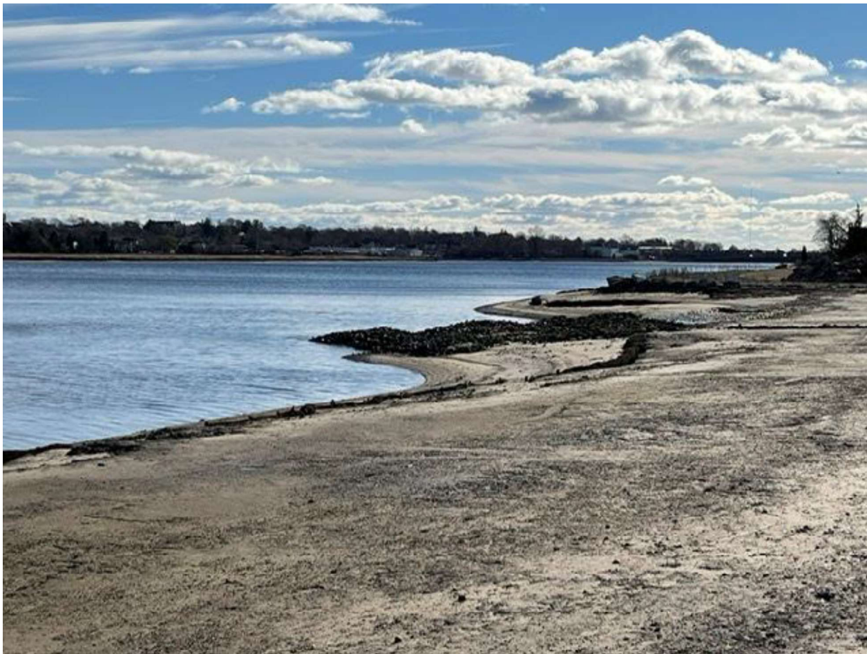
Figure 14: L-014 cap looking south. Bare soil is WZ-4 backfill waiting to be planted as saltmarsh in spring 2022 (after replacement of topsoil lost in October 2021 nor'easter).
