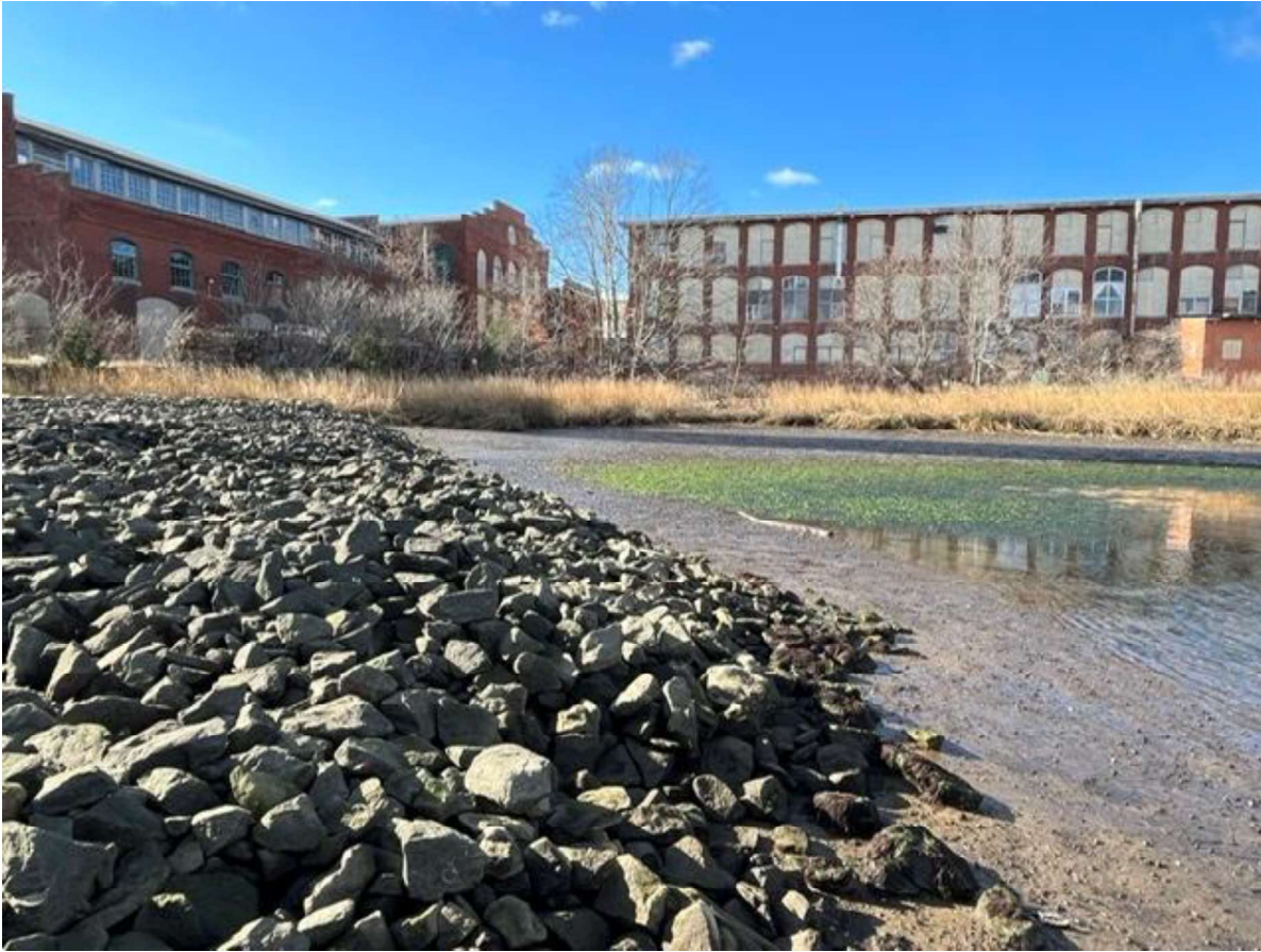
Figure 13: Crib cap. Looking west along northern edge of the cap.
