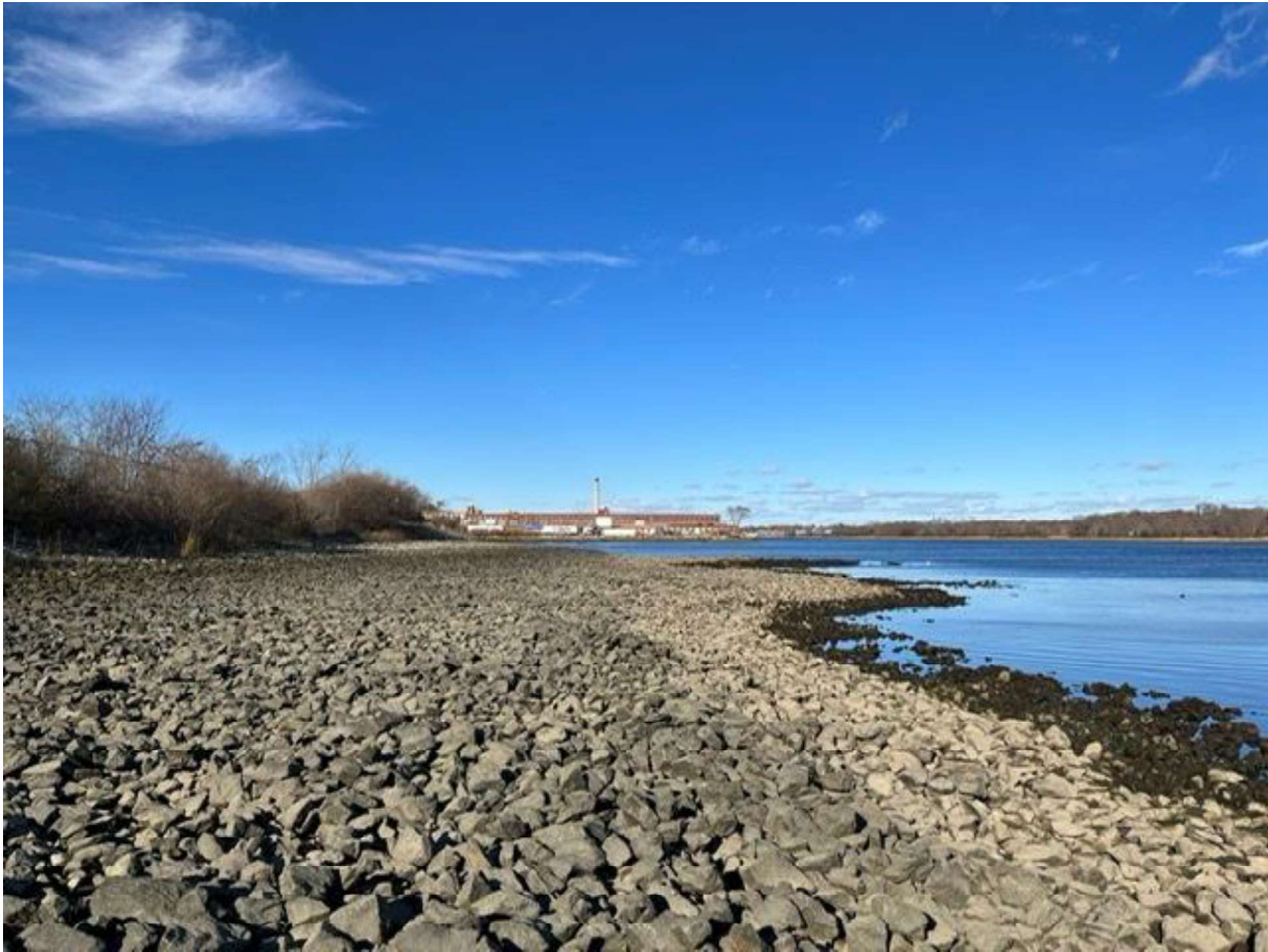
Figure 19: Pilot CDF shoreline cap, looking north.
