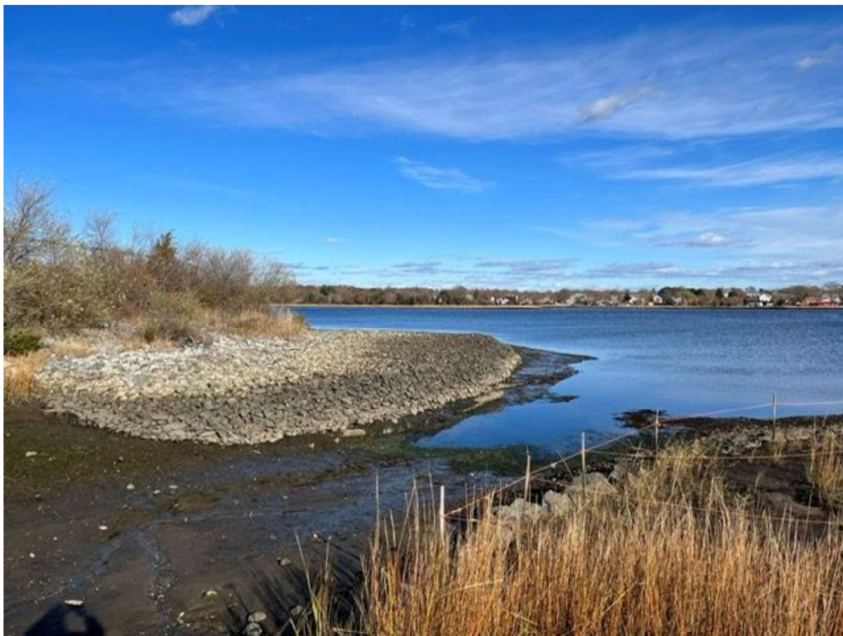
Figure 18: Pilot CDF shoreline cap , southern end, looking north. Parcel 265 saltmarsh replanting in fore-ground.
