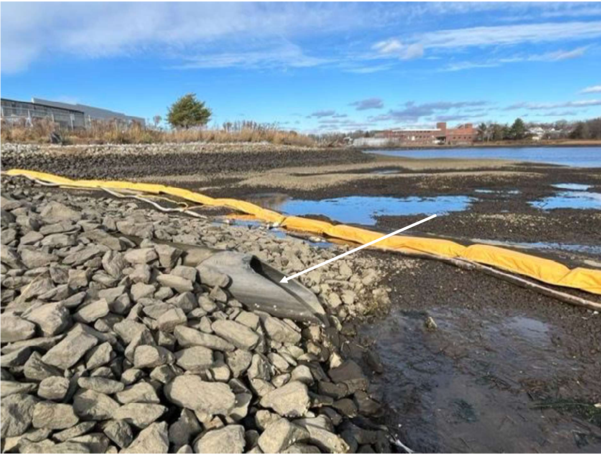
Figure 5: Aerovox cap looking north showing the North Trench outfall.
