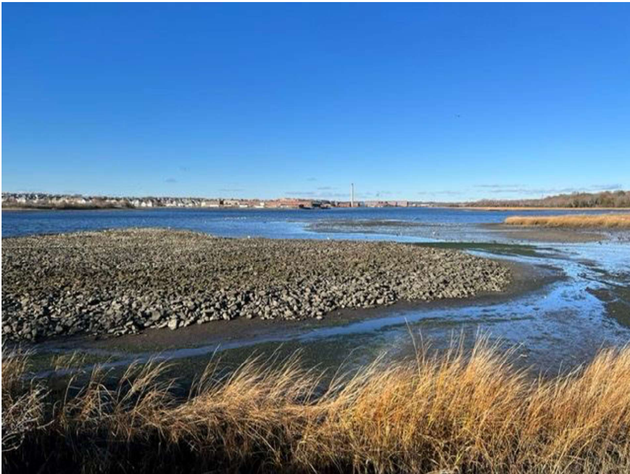
Figure 26: Cogg-East cap , eastern end, looking north.
