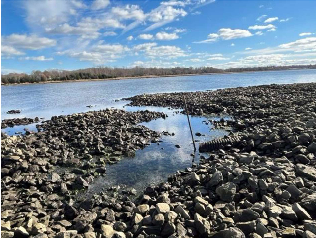
Figure 12: Crib cap looking SE showing storm drain outfall.
