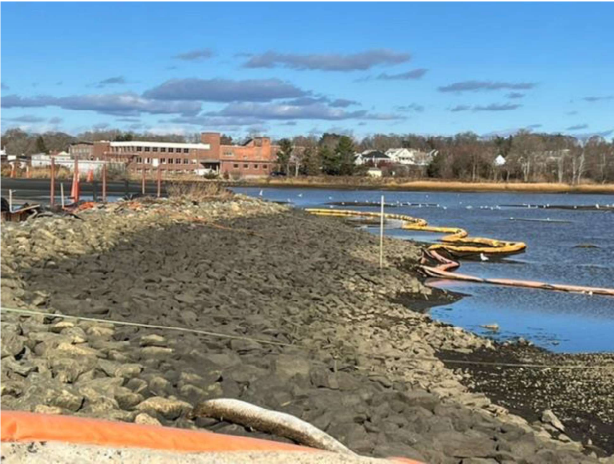
Figure 9: Aerovox cap , southern E/W leg, looking east. Note the serrated pattern at the lower edge of the bank armor stone.
