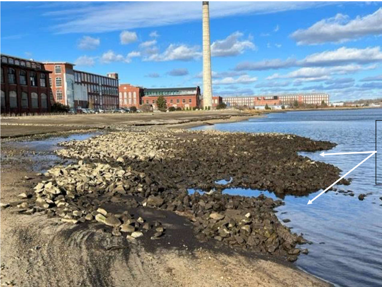
Figure 16: L-014 cap , looking north.
