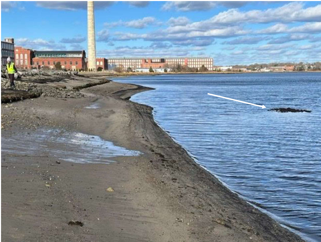
Figure 17: L-114 cap , looking north. Only a small area of emerging armor stone can be seen at extreme low tide.
