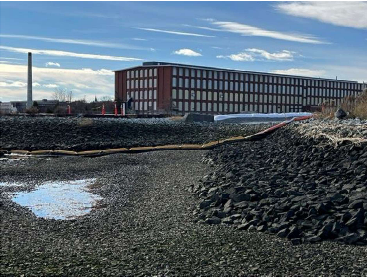
Figure 3: Aerovox cap looking south showing “capacitor cove.” Titleist building in background.
