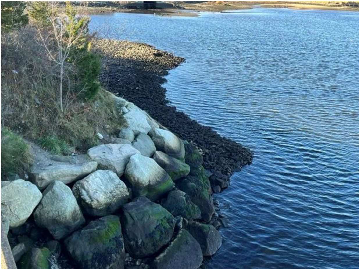
Figure 24: Cogg-West cap looking NW. Bridge opening in foreground.
