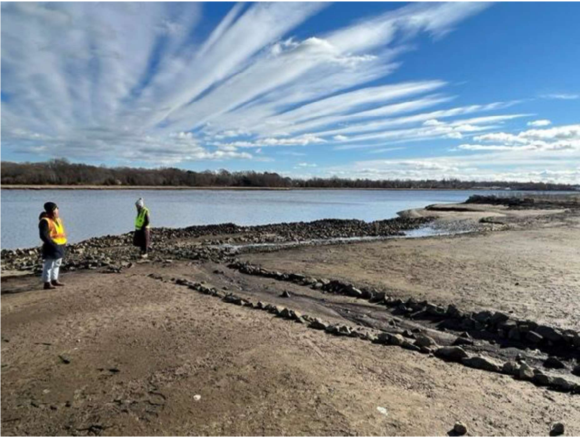
Figure 15: L-014 cap looking SE. Swale in foreground was installed as part of WZ-4 restoration.
