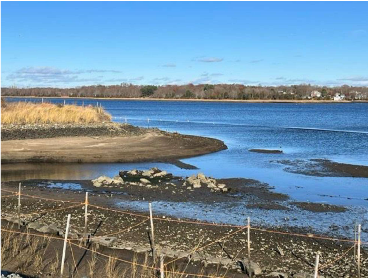
Figure 22: Parcel 265 stone cap looking NE.
